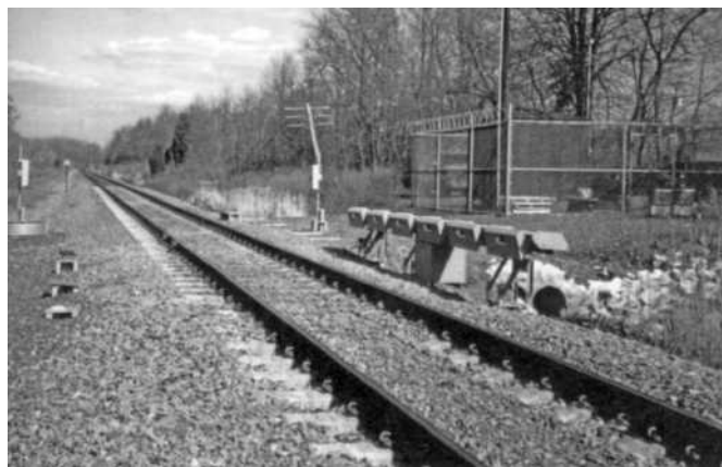
(c) Early detection of defective bearings
