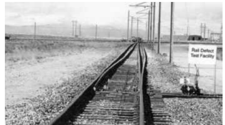
(b) Internal rail defect inspection
