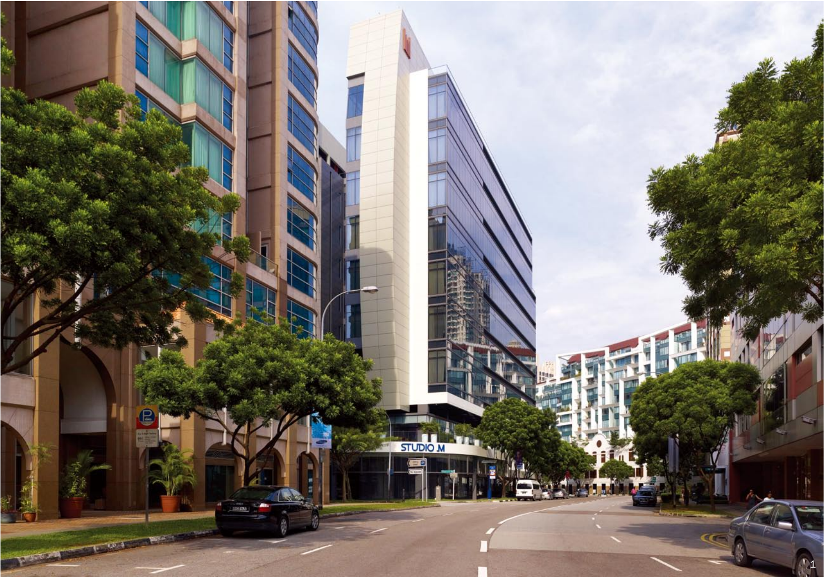
1. Front view of hotel 2. Back view of hotel
