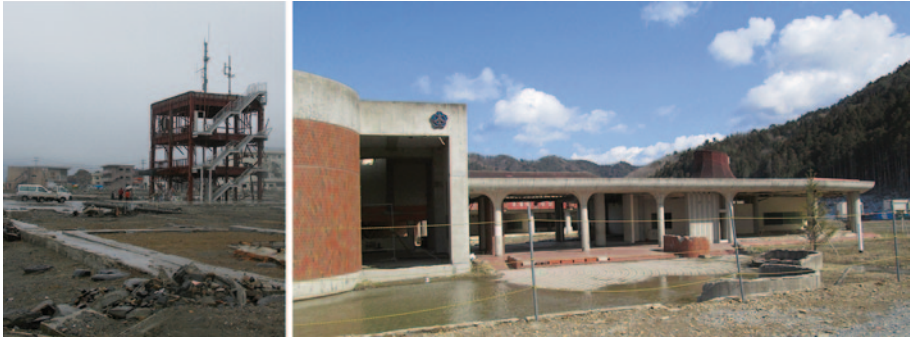
Fig. 2.4 The office building for disaster mitigation in Minamisanriku Town ( left ) and the Okawa Elementary School ( right ) in March 2014
