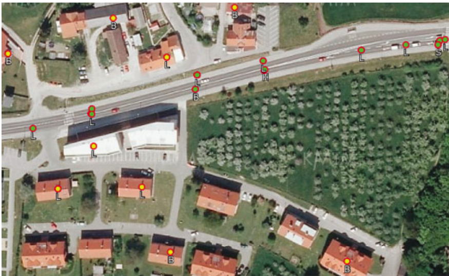
Figure 19.4. Questionable locations of traffic accidents attached to objects with house numbers (yellow markers), actual locations of traffic accidents on the roads (green markers). For a color version of the figure, see www.iste.co.uk/jacob/safety.zip
