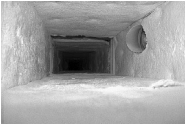
13.7 HVAC duct encapsulant lining.
