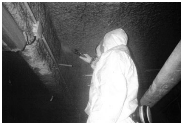
7.7 Worker removing indoor friable asbestos.
