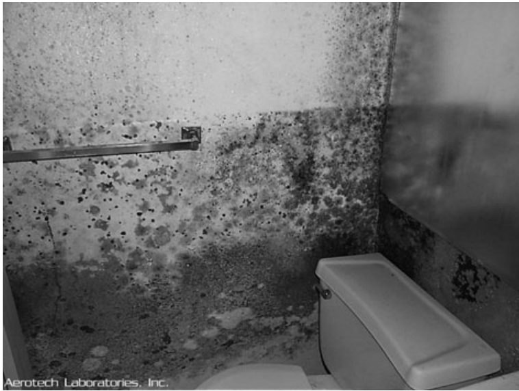
13.2 Bathroom mixture of Cladosporium , Aspergillus , and Penicillium on painted drywall surface.
