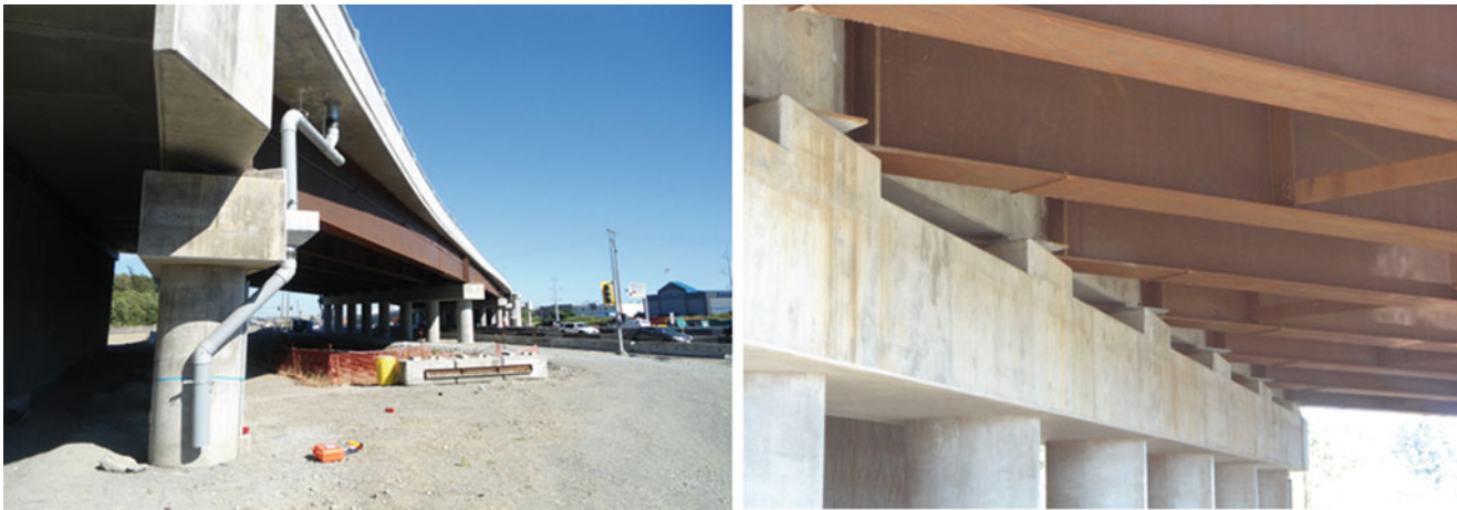
Fig. 15.4 Highway 1 and Lougheed highway underpass (LHH-EB underpass)
