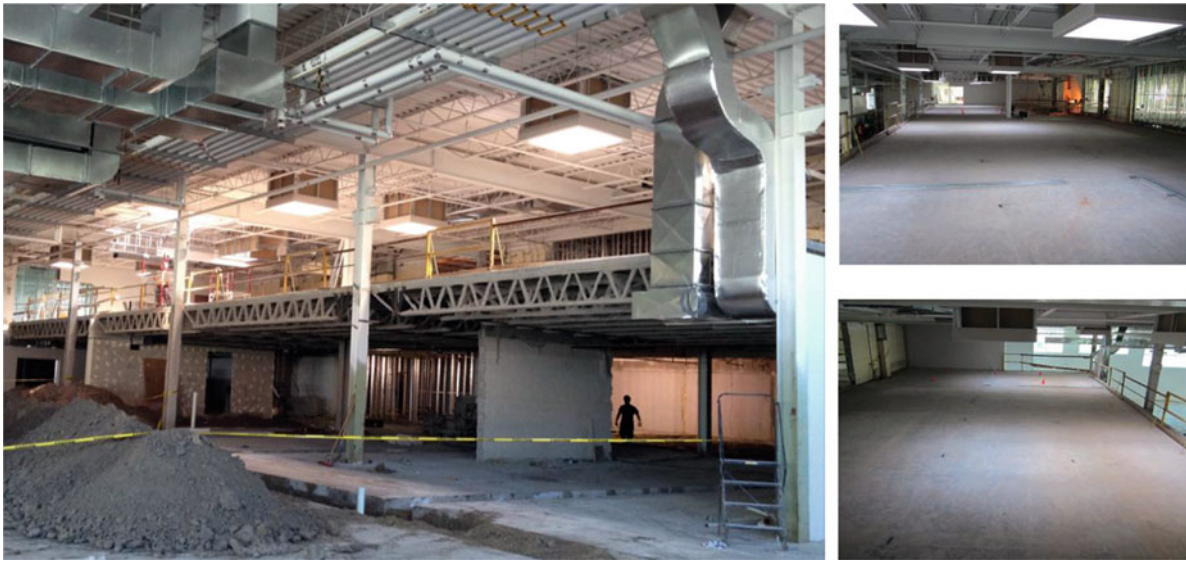
Fig. 47.1 Photos of the mezzanine floor assessed in this study
