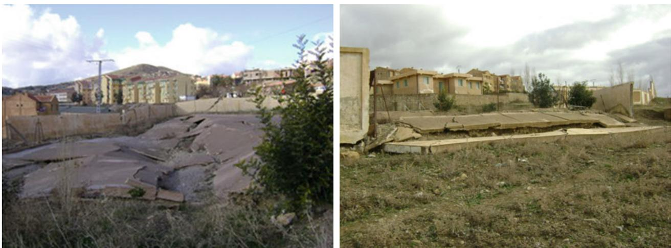
**Fig. 191.2** Landslide causing disorders to the stadium and surrounding wall
