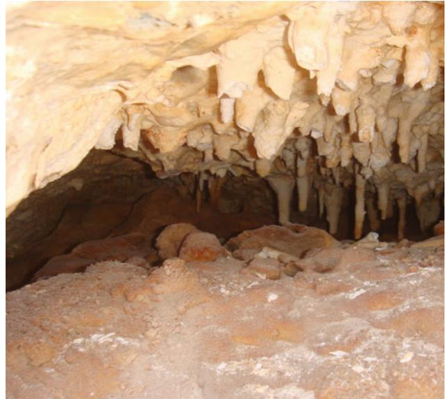
**Fig. 38.3** Karstic cavity in the tunnel T2
