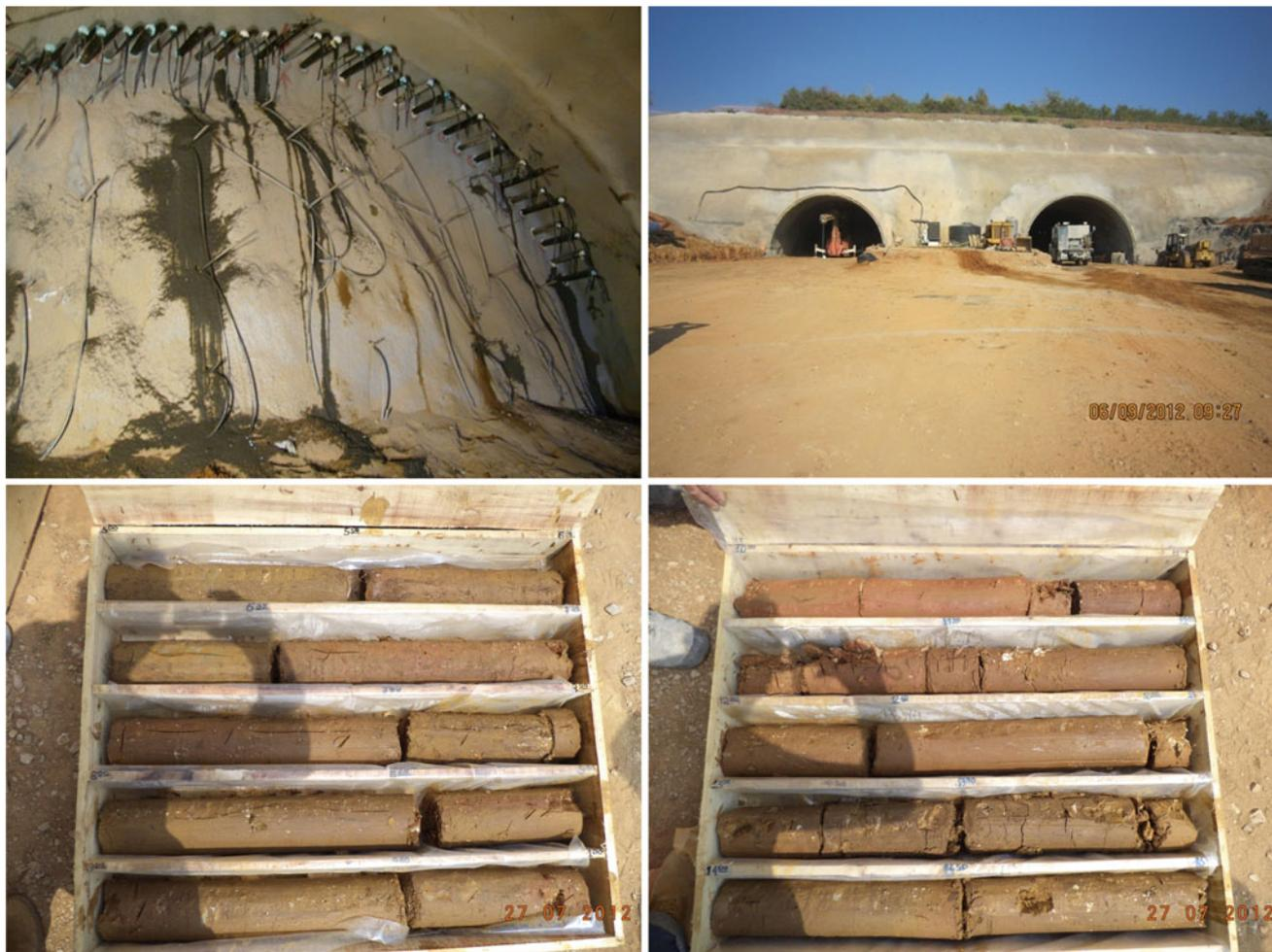
**Fig. 55.1** View on borehole core samples, tunnel tubes and forepoles as a face protection
