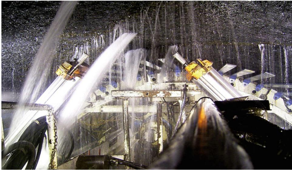
**Fig. 180.1** Random, heavy water inflow through massive basalts (*Kárahnjúkar Hydroelectric Project, Iceland. Headrace Tunnel*)
