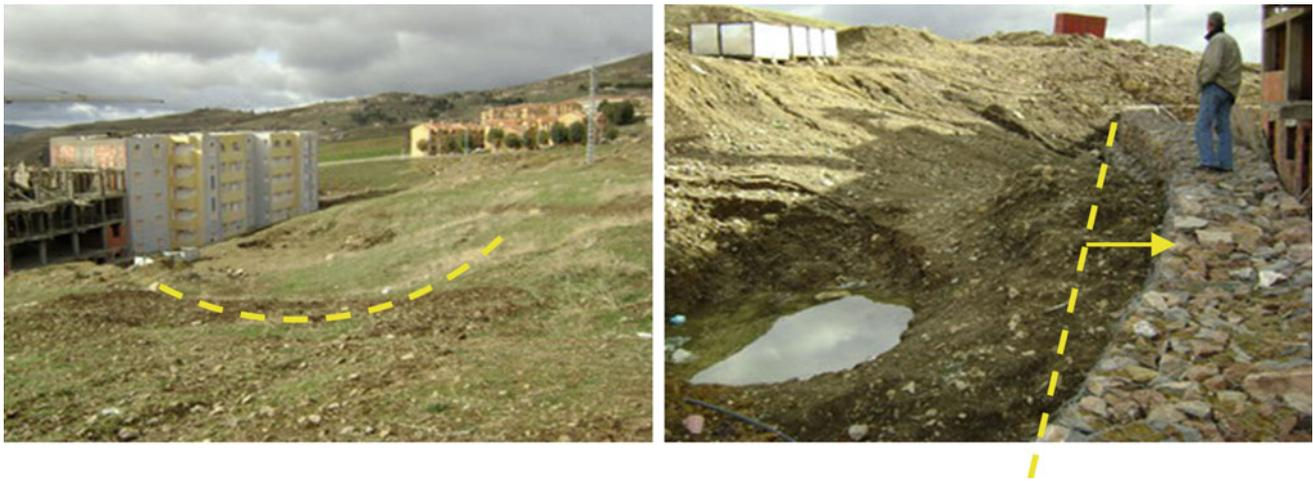
**Fig. 191.3** Tilted and moving retaining wall
