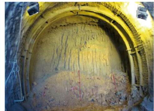
**Fig. 107.4** Excavation and Support Class “A” for the tunnel
