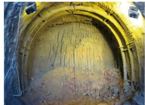
**Fig. 107.4** Excavation and Support Class “A” for the tunnel
