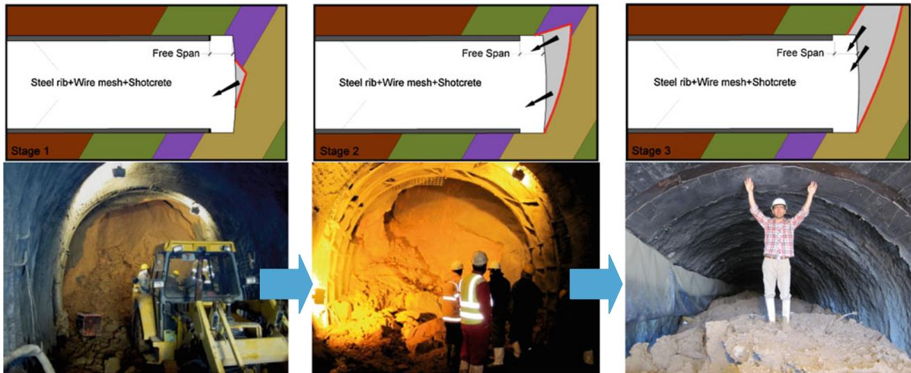
**Fig. 107.5** Collapse in initial part of Sabzkuh tunnel (T1) (Eftekhari et al. 2013b)
