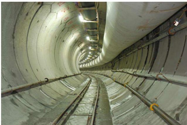
Fig. 171.1 Excavation of HRT by using TBM
