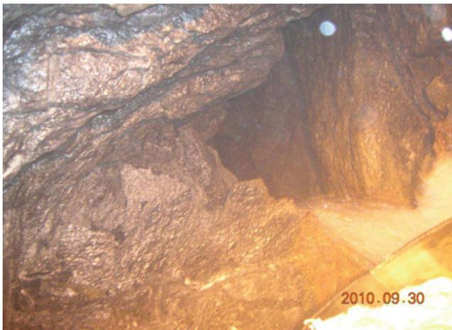
**Fig. 171.5** Close view of cavity and water ingress (which was later on diverted in to drift) above segment No. 1905 in HRT (TBM)
