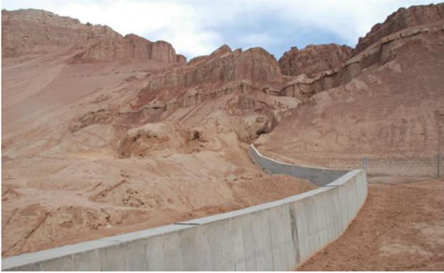
**Fig. 30.5** Diversion ditch for mudflow control
