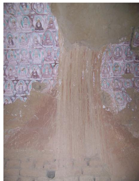
**Fig. 32.12** The cave roof rainwater infiltration induced by poor drainage
