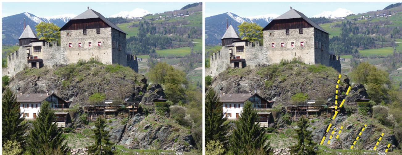
**Fig. 17.1** Eastern Flank of the hill of Summersberg Castle with a clearly visible fault and associated fractures dipping to south. The
