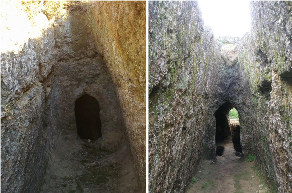
**Fig. 18.4** Entrance of tombs showing the presence of fractures and deterioration of the walls by erosion processes
