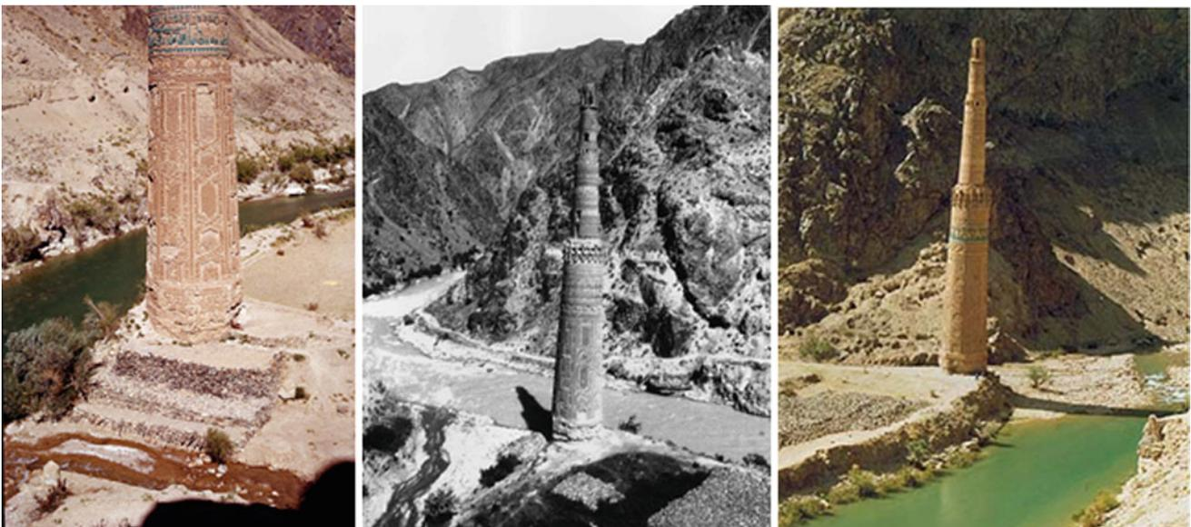
**Fig. 1.9** The embankment in 1963, 1986 and 1999, showing the river Hari Rud quite close to the minaret
