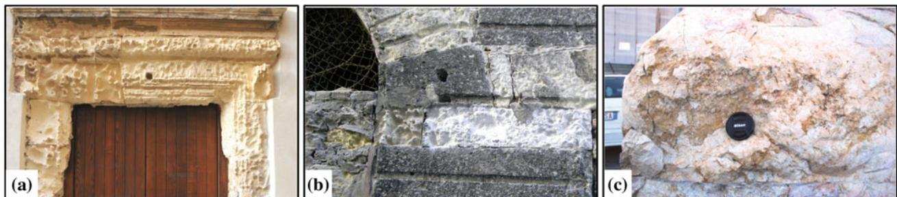
**Fig. 22.1** Different types of degrade: **a** Alveolization of the *Pietra Cantone*, **b** Detachment of material from a wall of *Tramezzario*, **c** Detachment of material from an architectural element of *Pietra Forte*
