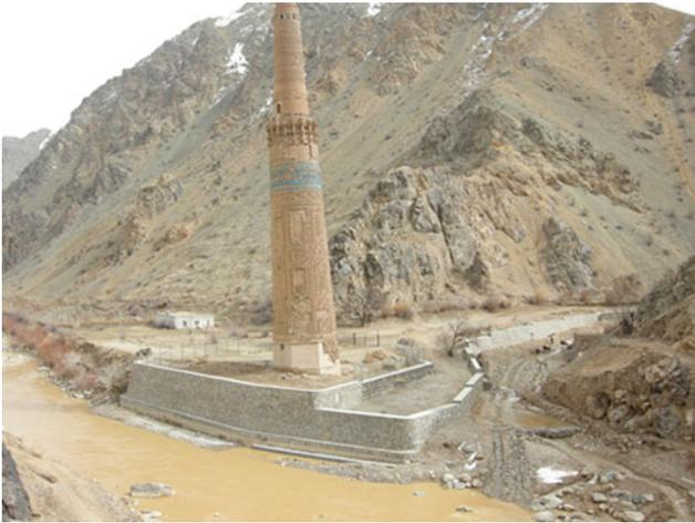
**Fig. 1.12** The emergency restoration work of Jam embankment after the destruction caused by a flooding in 2007
