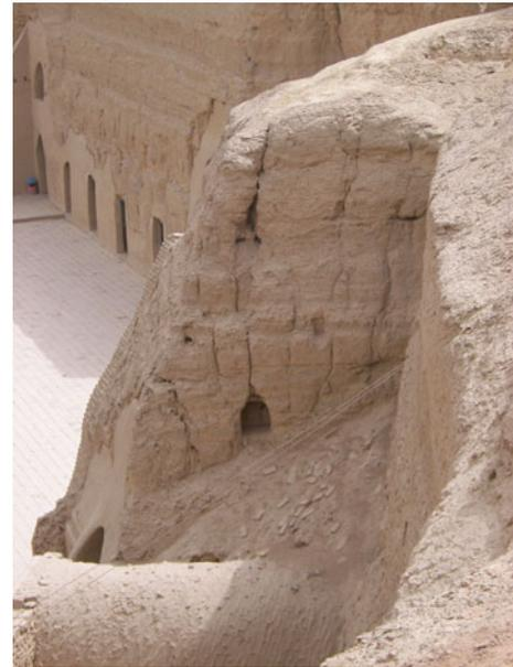
**Fig. 32.8** Facade fissure of the dangerous cliff
