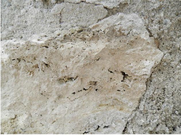
**Fig. 82.6** Travertine in the wall of glass production centre
