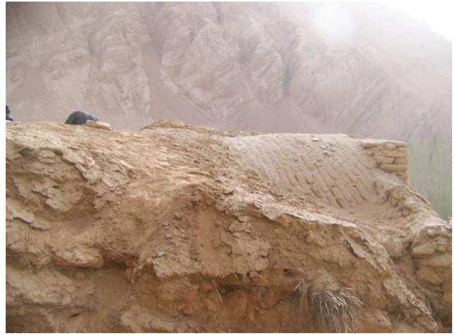
**Fig. 32.11** The cave roof collapsed
