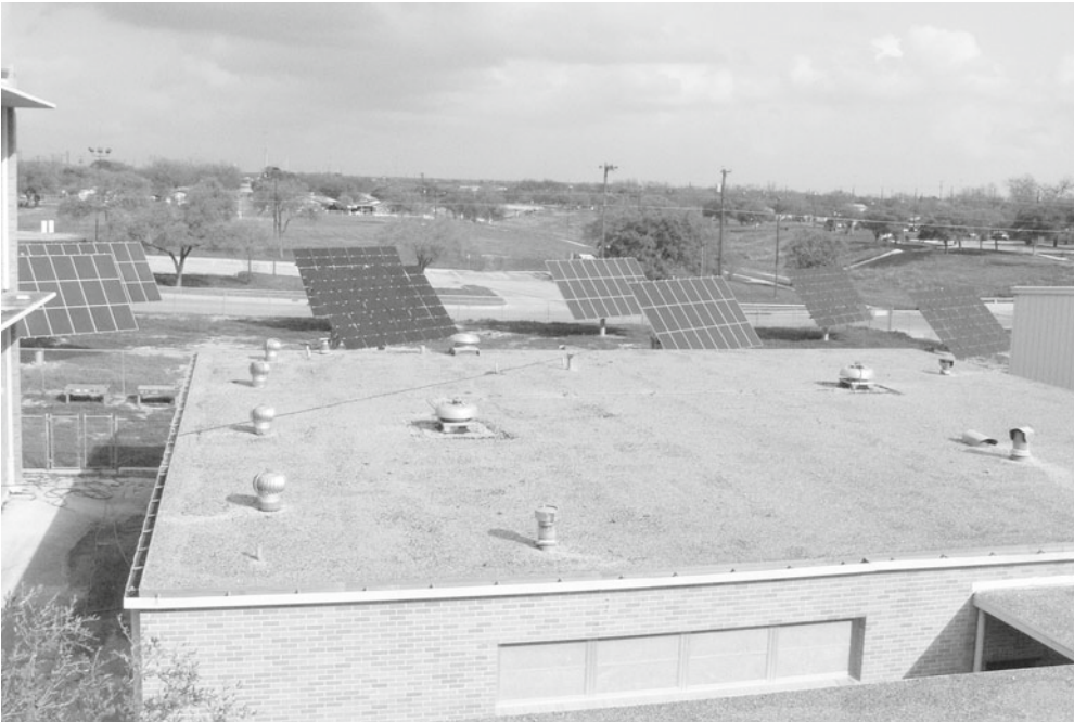
Figure 5.6. Mission Verde Center solar power system
