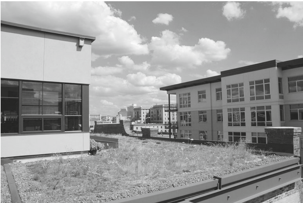
Figure 4.1. Ecotrust roof blooms, Portland, Oregon
