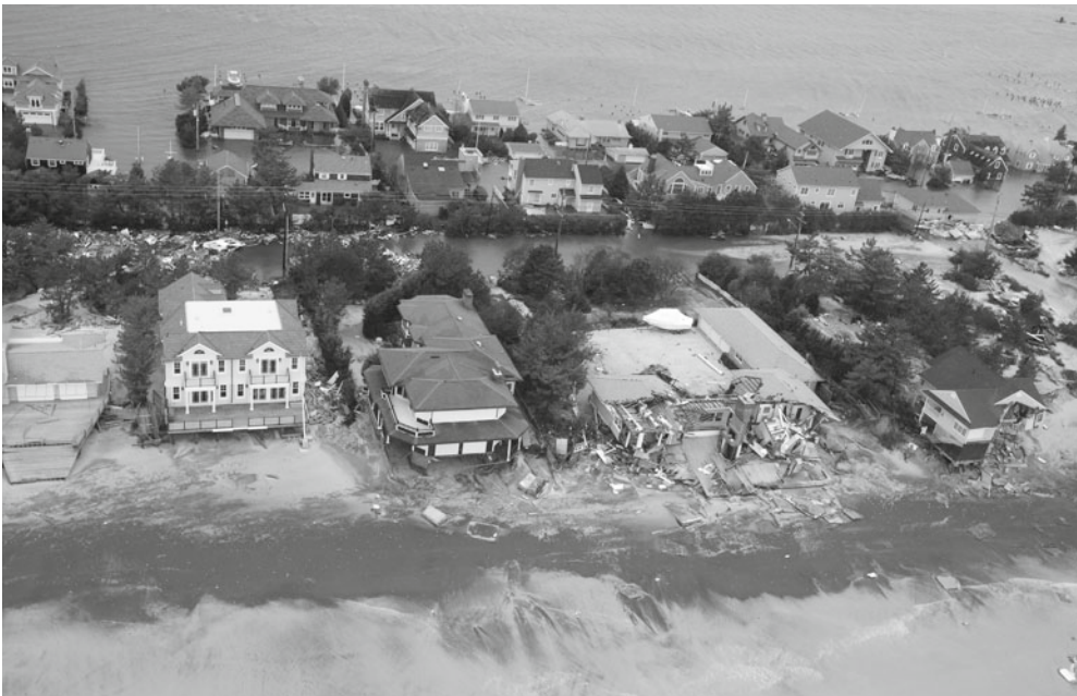
Figure I.2. Hurricane Sandy damage, Long Beach Island
