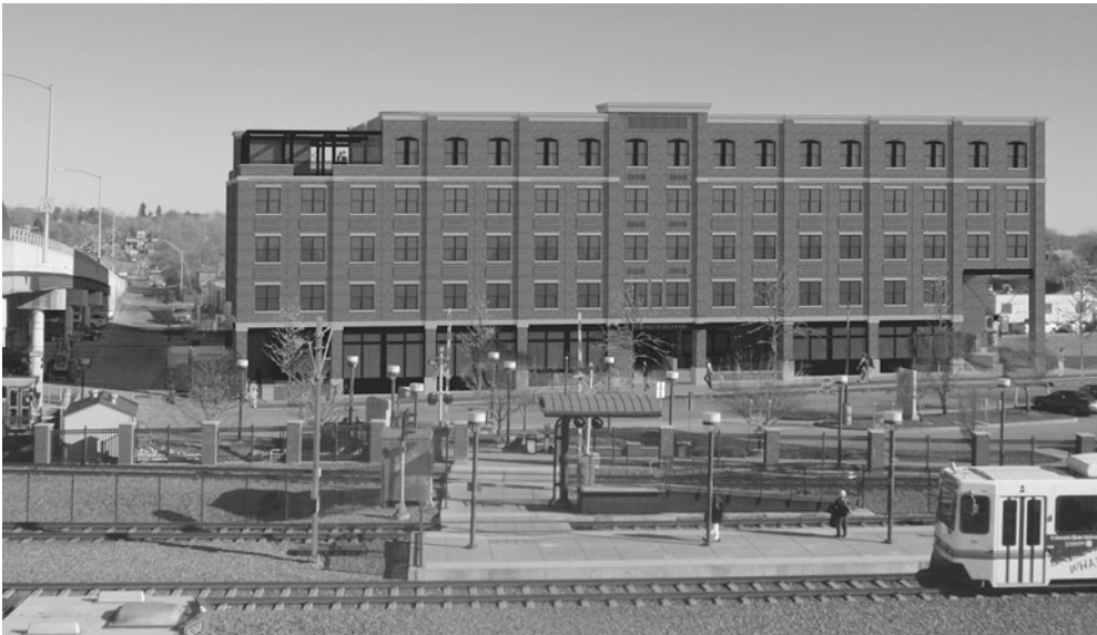
Figure 5.7. Evans Station Lofts project, Denver, Colorado
