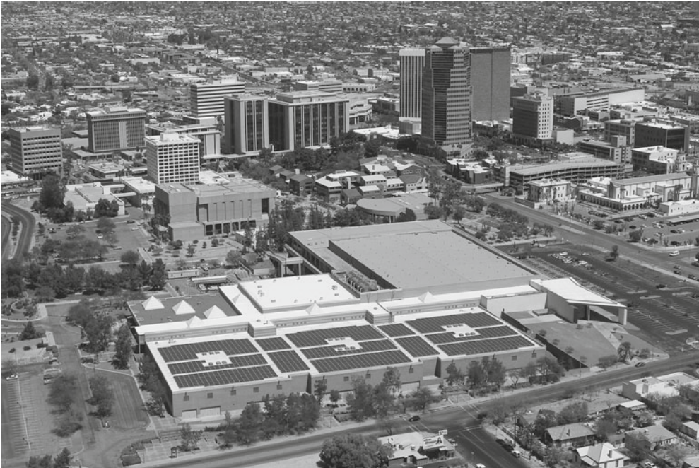
Figure 5.2. Tucson, Arizona, solar installation
