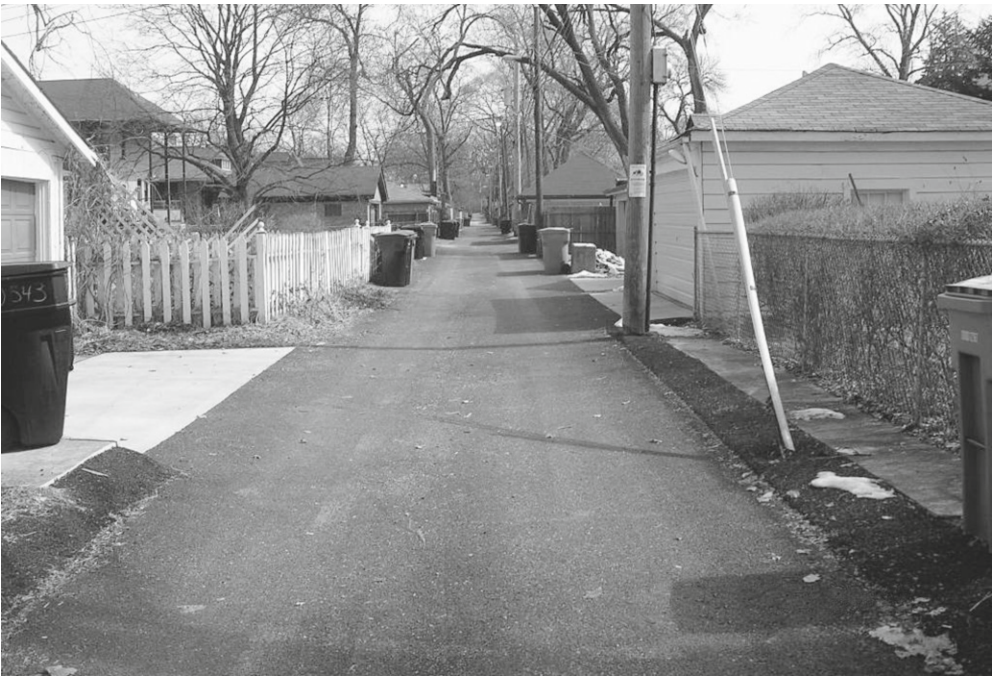
Figure 4.7. Permeable asphalt alley, Chicago
