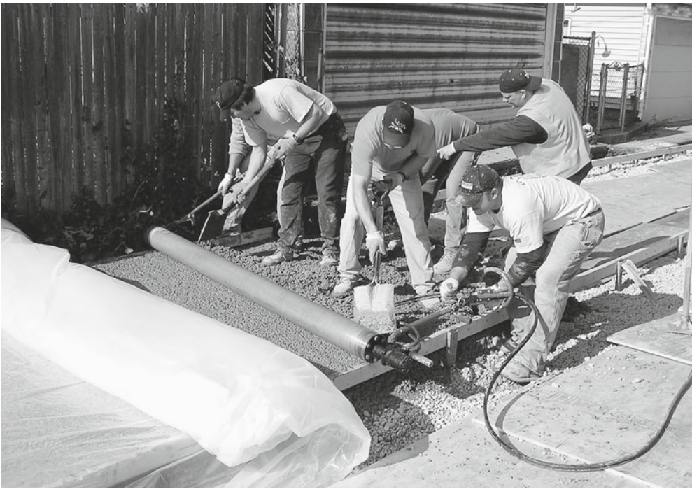
Figure 4.6. Green alley installation, Chicago
