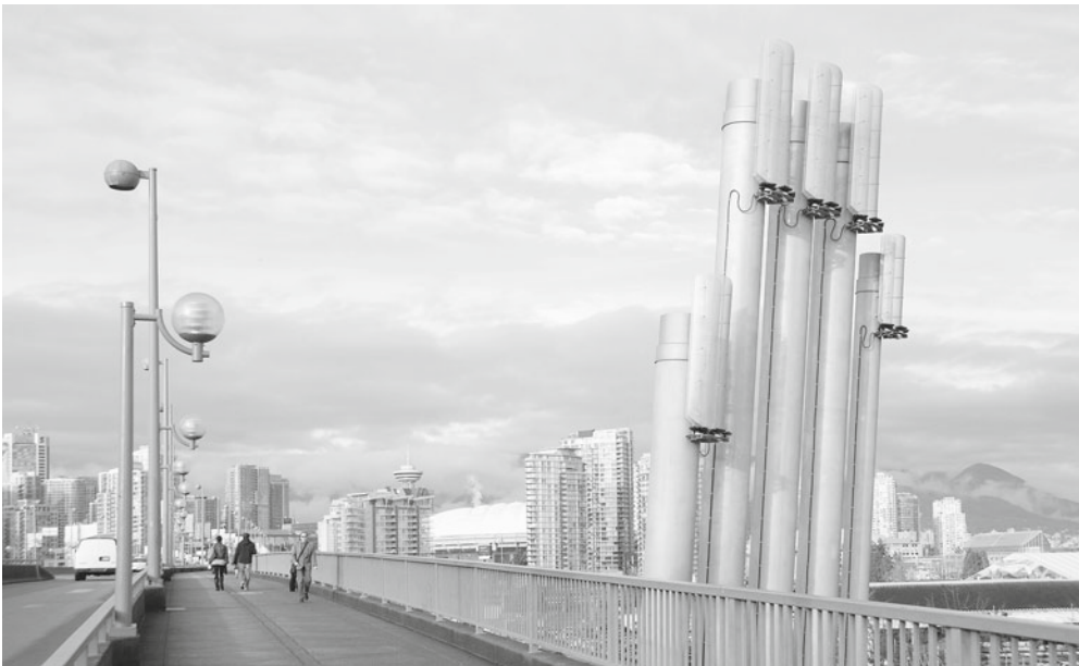
Figure 1.4. Vancouver district energy stack
