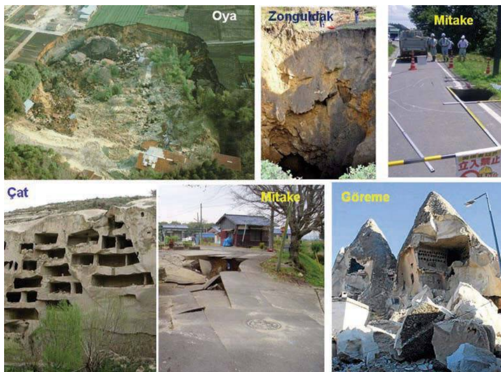
Figure 1.1 Collapse of some underground openings involving time-dependent characteristics of rocks.
