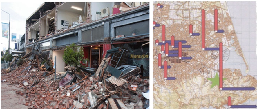
Fig. 1.5 Destruction caused by vertical shock in Christchurch, 22nd February, 2011 (left) ( http://www.shutterstock.com/pic-71750008/stock-photo-christchurch-nz-feb-destruction-caused-by-earthquake-on-february-in-christchurch.html?src=vIQW8OCGcQm0BrtHWeo6bA-1-53 ). Vertical ground acceleration was 2.2 g . The green star indicates earthquake epicentre (right) [91]
