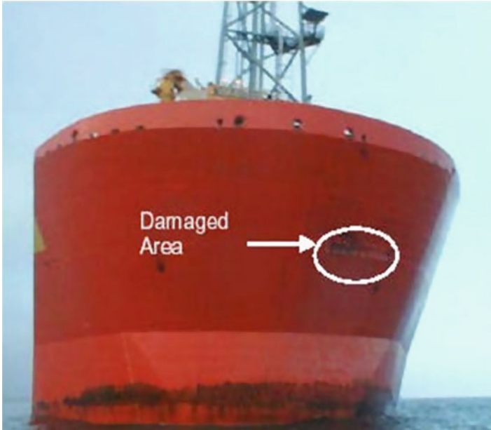
Fig. 6.43 Photograph showing a damaged area as a result of local loading of the hull by a steep wave [64]
