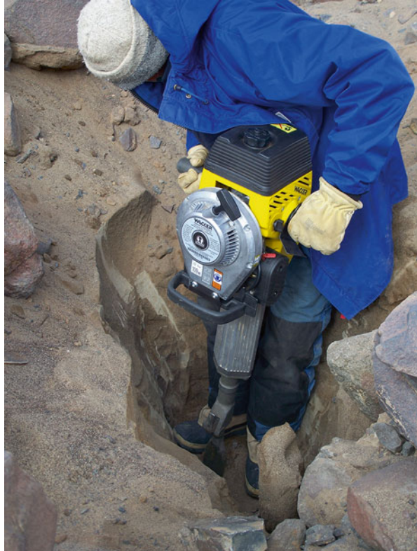
Fig. 3.5 Portable gasoline-powered hammer used to excavate frozen soil in Beacon Valley, Antarctica (Photo by M. Kurz)
