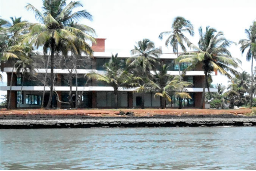
Fig. 7.41 A hotel under construction on the Goa coast ( 15^{\circ} 29' 5.1''\text{N} and 73^{\circ} 47' 40.9''\text{E} ); photograph taken on 4 April 2013 by Ms. Ankita Mitra (Environmentalist)
