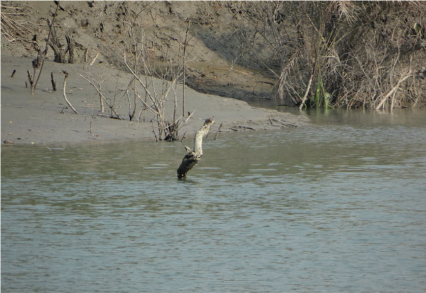
Fig. 8.18 Steep intertidal mudflats are prone to erosion leading to a failure of the afforestation programme
