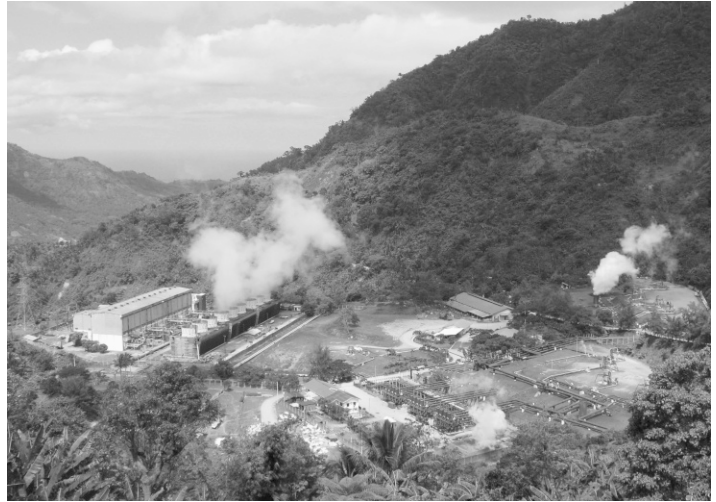
The Palinpinon Geothermal Power Plant in Negros Oriental, Philippines.
