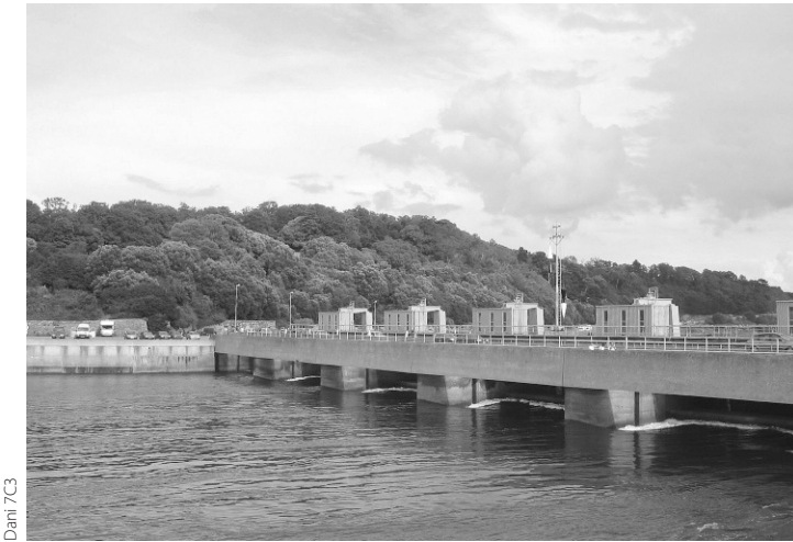
Dam of the tidal power plant on the estuary of the Rance River, Brittany, France. It has been in operation since 1966.
