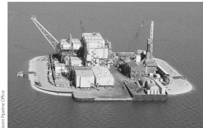
An oil and gas drilling installation on an artificial island built for the purpose in the Beaufort Sea north of Alaska.
