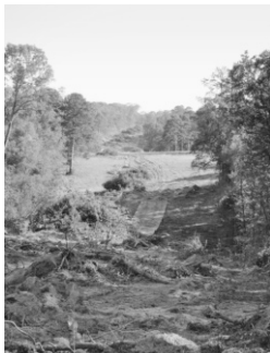
clearcutting the pipeline route
