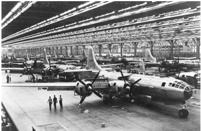
The flow of output: a B-29 assembly line in 1944.
