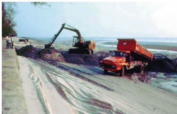
Fig. 4.10 Renourishment of the beach at Morib, Malaysia, by dumping sand from lorries. © Geostudies
