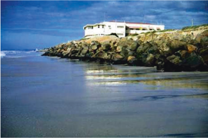
Fig. 2.16 Beach at Surfers Paradise, Queensland, lowered by large waves reflected from a boulder wall during a tropical cyclone. © Geostudies
