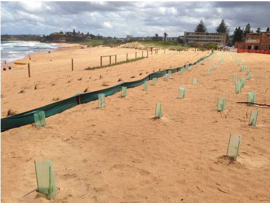
Fig. 3.12 Planting of dune vegetation on Mona Vale Beach, Australia in 2013 in an attempt to halt erosion by restoring and stabilising the dune system. The stabilised dune is intended to protect coastal properties, avoiding the need for structural engineering or other ‘soft’ measures such as beach renourishment. © Nick Lewis
