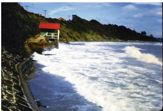
Fig. 5.1 The shore south of Black Rock in 1968, when storm waves at high tide were eroding the base of the backing bluff. © Geostudies
