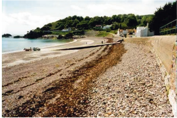
Fig. 4.6 The shingle beach at Anne Port, Jersey, renourished with gravel shipped from Ireland. © Geostudies
