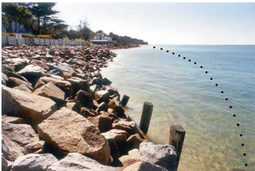
Fig. 2.9 The yacht club at Somers, Western Port Bay, Australia, was built on a sand lobe (out-line: dotted line ) that had migrated to this position, and then moved on along the coast. A boulder rampart has been inserted to halt erosion here. © Geostudies
