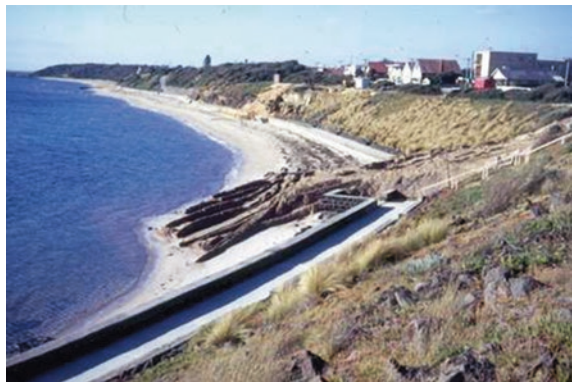
Fig. 4.3 Sand dumped from lorries on the shore at Black Rock, Victoria, Australia. © Geostudies
