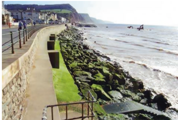
Fig. 4.16 The sea wall at Sidmouth in South Devon was reinforced by dumping stone blocks after the bordering beach was depleted by erosion. Shingle was then added to restore the beach, which now looks similar to that at Seaford (Fig. 4.15). © Geostudies
