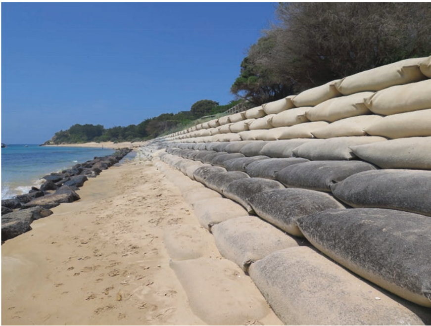
Fig. 2.11 A sandbag rampart marks the site of beach erosion at Portsea, Port Phillip Bay, Australia, in 2013. © Geostudies
