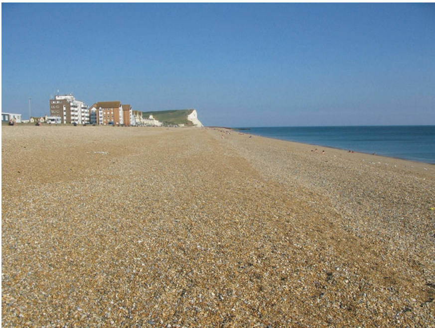
Fig. 4.15 The renourished shingle beach at Seaford, Sussex in 2013. The renourished beach is retained by a breakwater at the eastern (downdrift) end. © Geostudies
