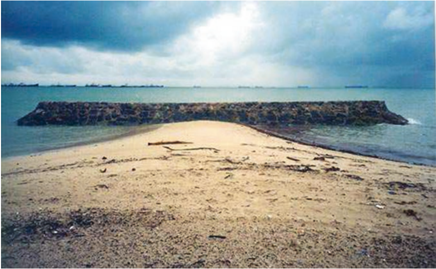
Fig. 3.9 Tombolo formed in the lee of a breakwater on the coast of Singapore. © Geostudies
