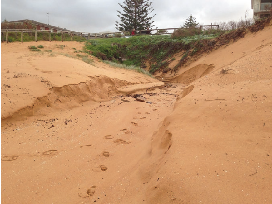
Fig. 2.14 A channel cut through the beach and dune on Collaroy-Narrabeen beach, Sydney, Australia caused by storm water discharging from a drainage outfall. © Nick Lewis
