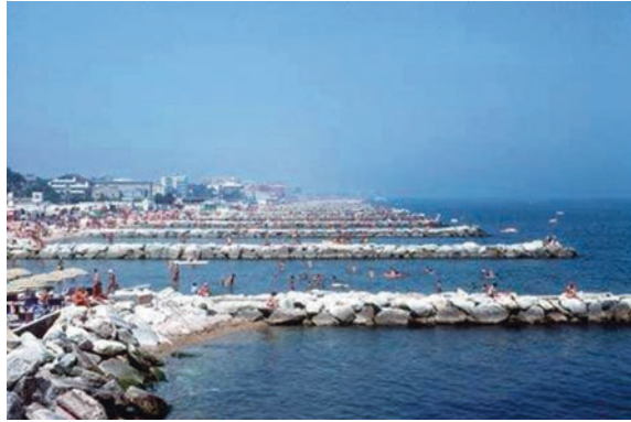
Fig. 3.5 Groynes on the Italian coast at Ravenna have failed to retain beach sediment, which has been withdrawn seaward and lost alongshore. © Geostudies
