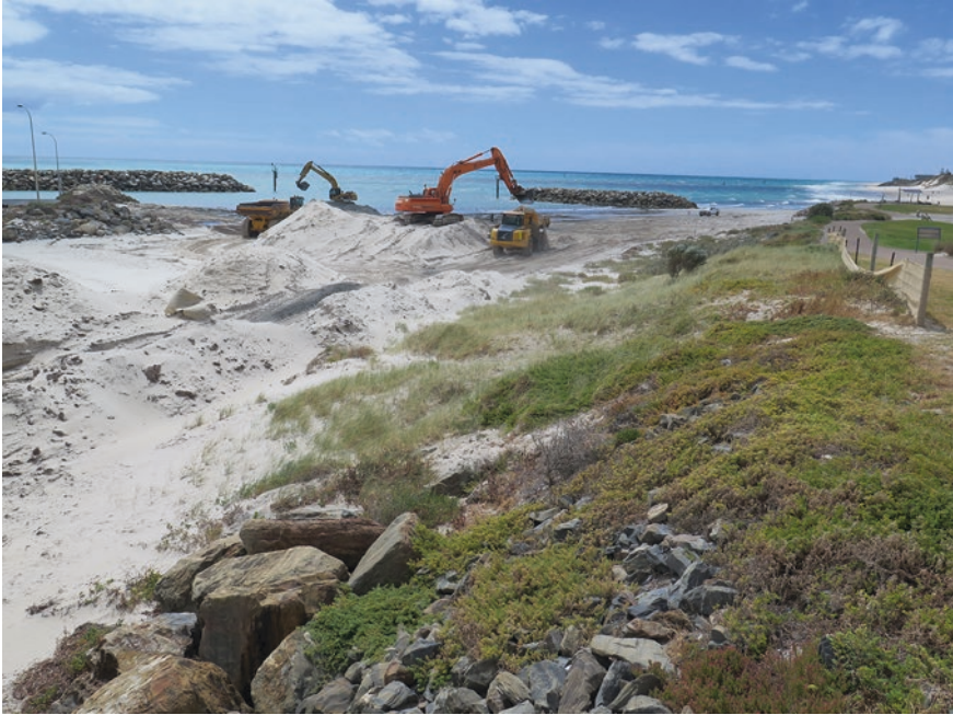
Fig. 4.24a Northward drifting sand on the Adelaide coast trapped by a breakwater near West Beach is loaded into trucks and carried southward along the beach to Glenelg (Fig. 4.24b). © Geostudies
