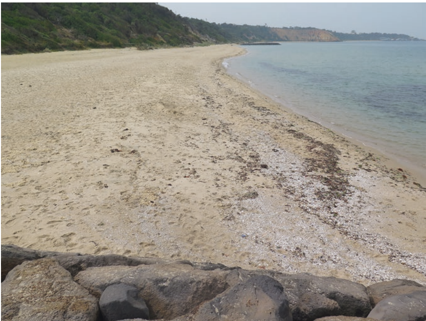
Fig. 5.6 The renourished beach between groynes at Sandringham, Port Phillip Bay, in 2010. © Geostudies
