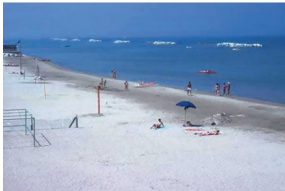
Fig. 3.8 Chain of boulder breakwaters protecting the beach on the coast at Rimini, Italy. © Geostudies
