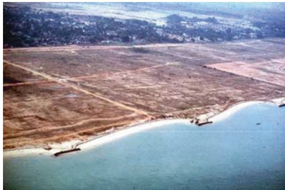
Fig. 3.6 Headland breakwaters separating beach compartments fronting reclaimed land on the south-east coast of Singapore in the 1970s. South-westerly wave action formed asymmetrical beaches between the breakwaters, but these did not remain stable, erosion continuing on the asymmetrical alignments. © Geostudies
