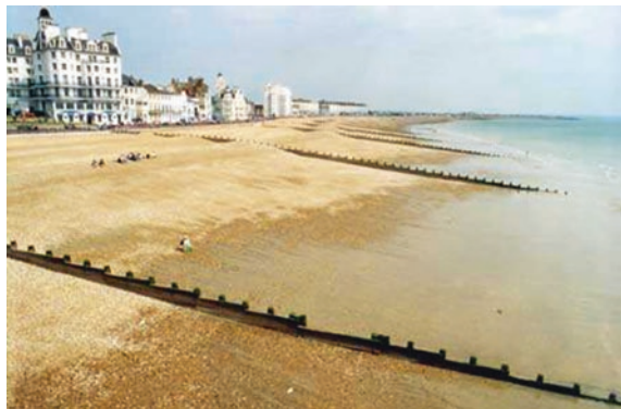
Fig. 3.2 Groynes defining beach compartments at Eastbourne on the Sussex coast, England. © Geostudies
