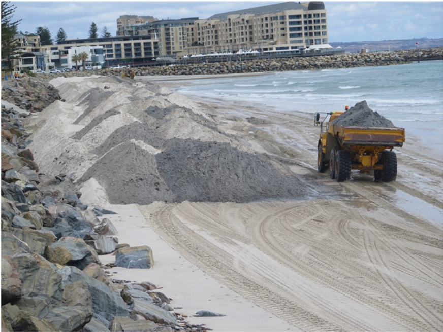
Fig. 4.24b Sand heaps delivered to the depleted southern end of the beach at Glenelg, Adelaide for beach renourishment. © Geostudies
