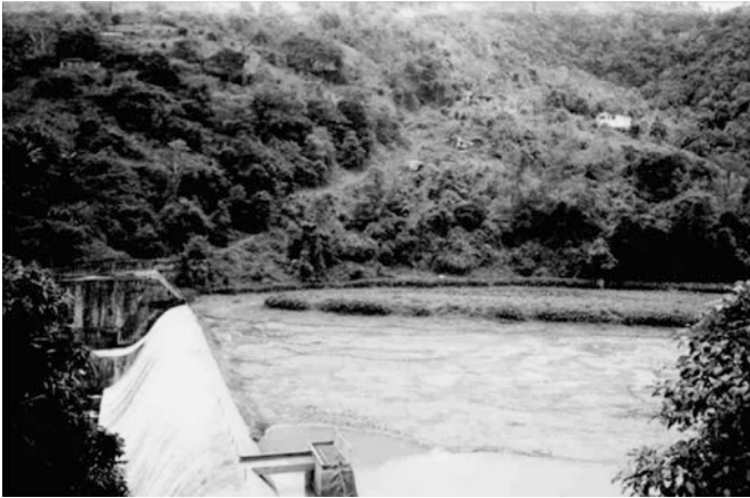
Fig. 1.4 Photograph presenting complete sedimentation in Comerío Reservoir in 1989. The reservoir was built in 1914 with a storage capacity of 6.06 \times 10^6 \text{ m}^3 and by 1935, was almost 70 % filled with sediment (Nevares and Dunlop 1948)
