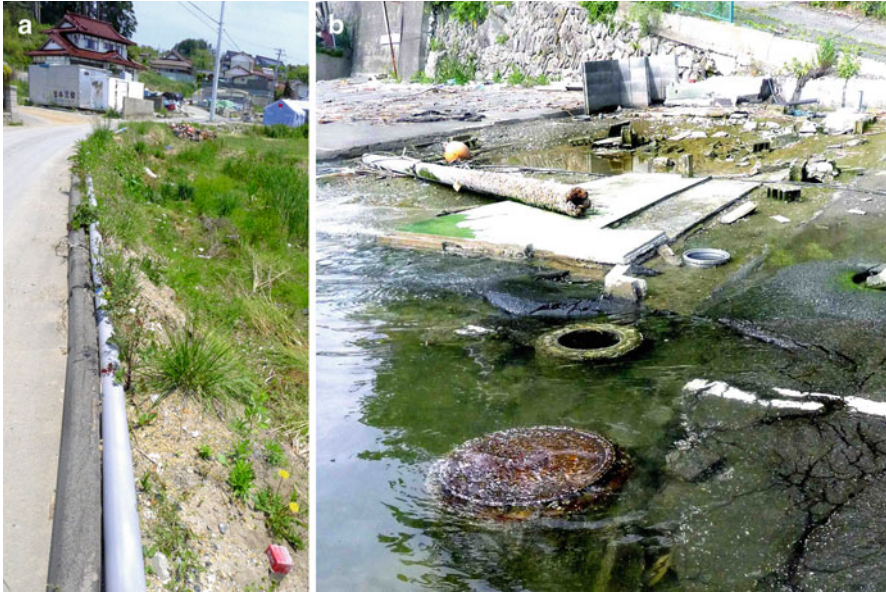
Fig. 1.39 (a) and (b) Provisional water supply PVC line and submerged drainage, a commonality along Sanriku cities and towns
