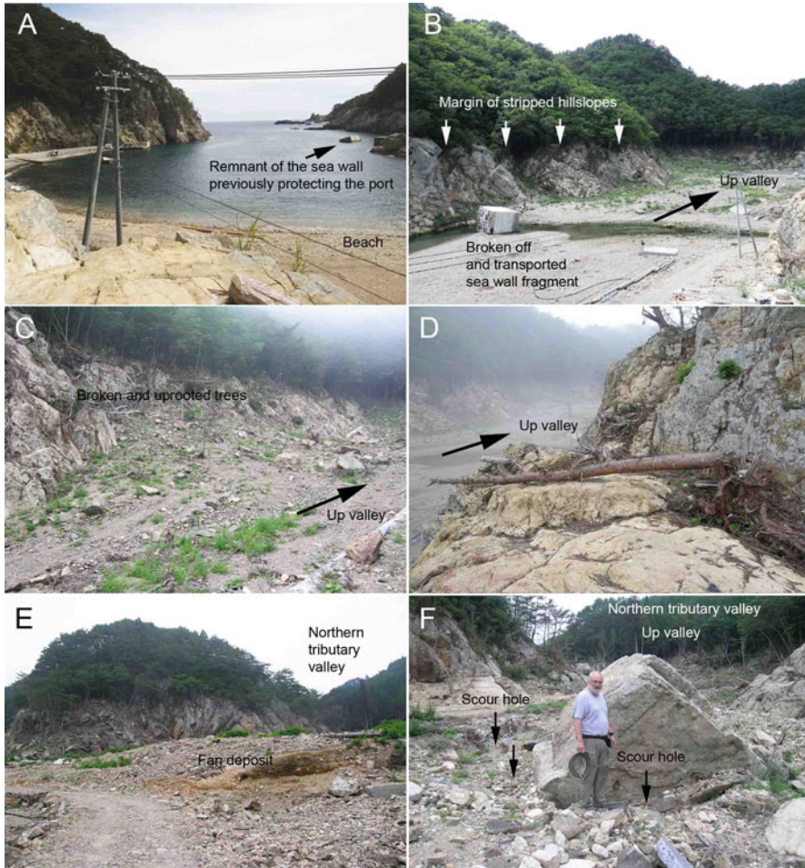
Fig. 13.3 Erosional and depositional features observed at Aneyoshi. (a) The Aneyoshi port and a remnant of the destroyed sea wall. The gravel-rich beach was eroded and probably provided some of the sediment that was deposited in the northern tributary valley. The electric lines were installed after the tsunami. (b) A large concrete section of the sea wall protecting the Aneyoshi port. The section was broken off, transported and deposited by the tsunami onto the former beach. Note the stripped hillslopes. (c) Stripped hillslopes along the main valley. (d) A tree knocked over by the tsunami high above the valley floor. (e) Gravel-rich sediment, visible in the fan deposit. This was at least partially deposited by the tsunami waves as velocities decreased up the northern tributary valley. (f) Scour hole generated around a large boulder over 5 m in size, located in the northern tributary valley
