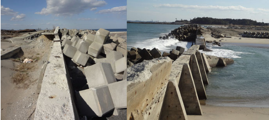
Fig. 16.1 Levees broken by the tsunami on the Yamamoto Coast of the Southern Sendai Bay Coast
