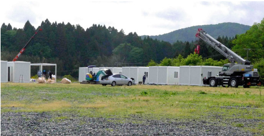
Fig. 1.11 Wooden temporary housing being built in Utatsu; Miyagi prefecture
