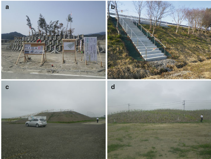
Fig. 17.7 (a) Seawall making use of tsunami debris in Rikuzen-Takata city (29/4/2012), (b) Stair on expressway in Sendai city (25/1/2012), (c) Increasing land elevation in Natori city (3/8/2012) and (d) Hill of thousand years hope in Iwanuma city (3/8/2012)
