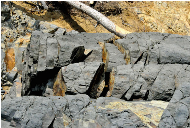
Fig. 1.15 Broken cliff formation in Motoyoshi, Miyagi prefecture
