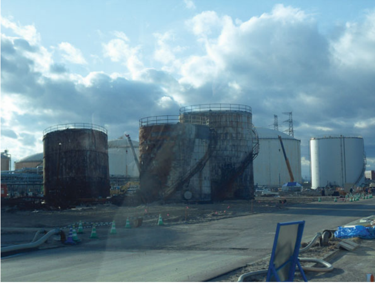
Fig. 15.7 Fires and threats to surrounding facilities: Case of a Japanese refinery damaged by fires that occurred during the sequence earthquake-tsunami Tohoku, March 2011 (Author’s pictures)
