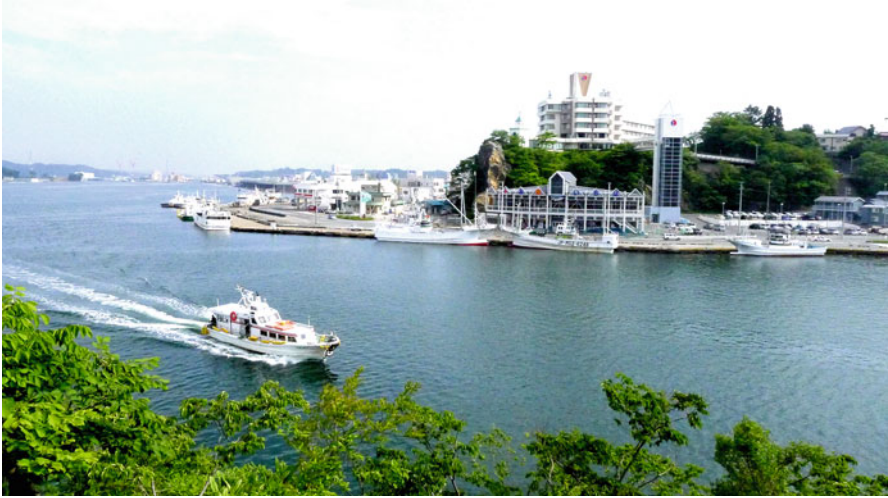
Fig. 1.36 Kessunma City port being reconstructed in 2102; Miyagi
