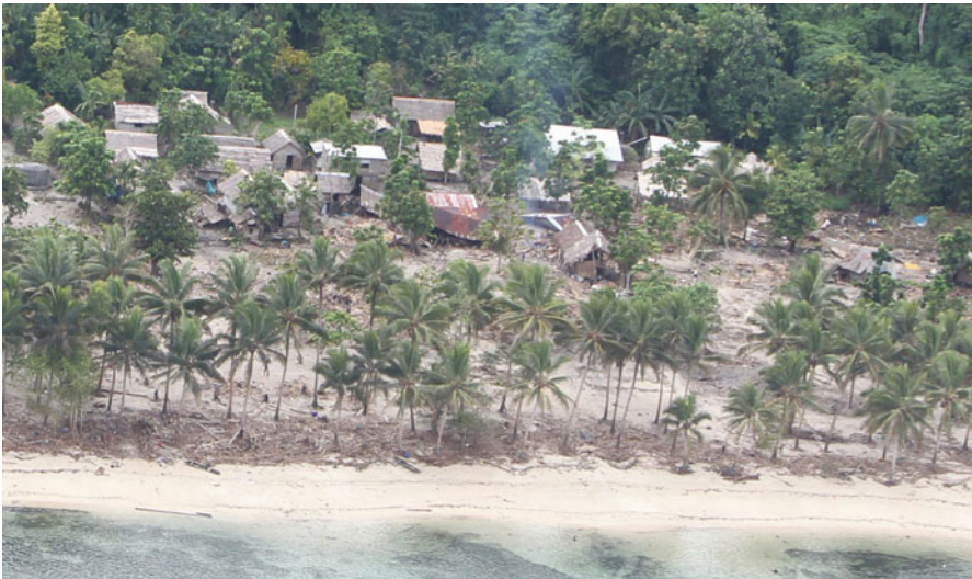
Fig. 22.3 Aerial photograph of west Nendo Island (Santa Cruz Island), showing damage to homes from the 6 February 2013 tsunami (Source: Solomon Islands National Disaster Management Office, Royal Australian Air Force)
