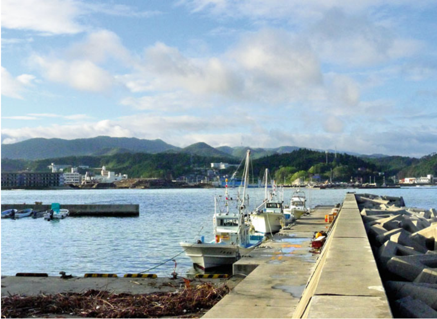
Fig. 1.44 Sea fences could not match the power of the tsunami run-up along the coast of Miyagi
