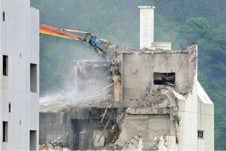
Fig. 1.46 Removal of a tsunami-damaged Senior Home building in Minamisanriku
