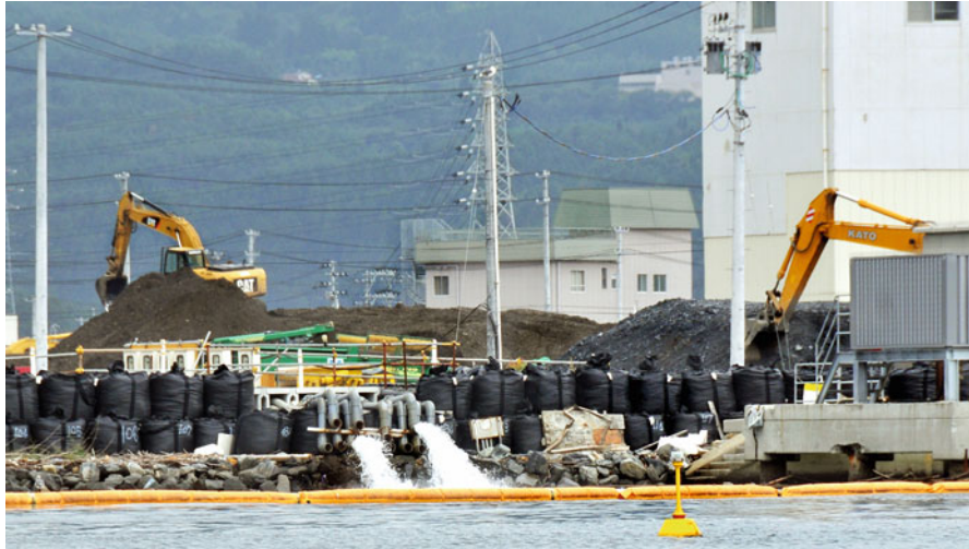
Fig. 1.18 Leveling-up the ground in Ksennuma port
