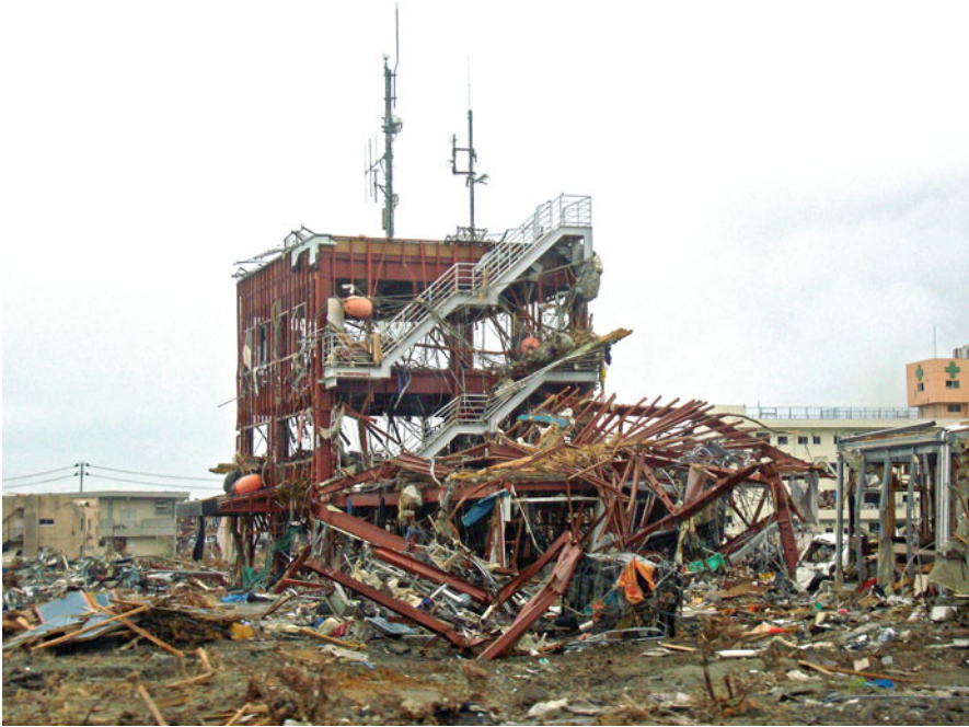
Fig. 1.2 Minamisanriku city hall; 2011
