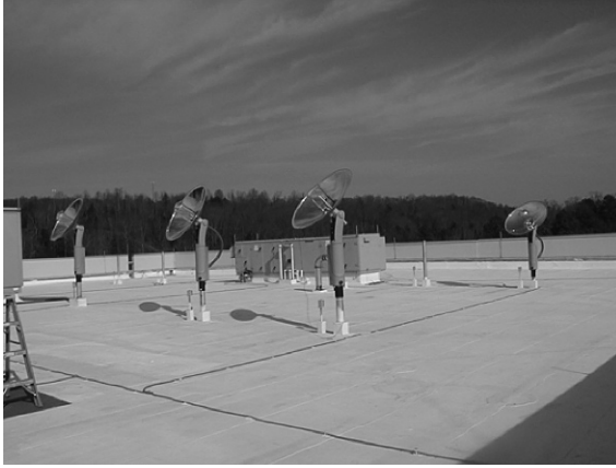
Fig. 5.18 Four HSL units being installed on newly constructed ORNL building
