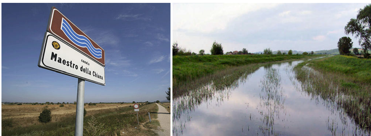
Fig. 9.22 The canale maestro della Chiana (main canal of the Chiana valley), in Tuscany, an artificial canal that runs for 62 km from the Chiusi lake to the Arno river. The canal was part of a drainage system
