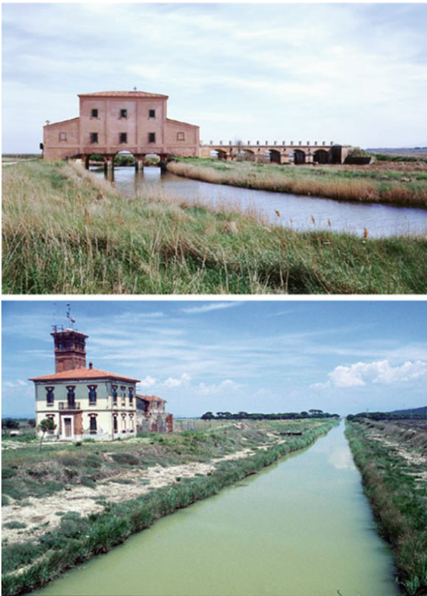
Fig. 9.23 Two images of the Grosseto plain (Tuscany) initially submitted to the colmata system, which exploited the cloudy waters of the Ombrone river and then drained by pumps (the white building in the picture below is that where the pumps are located). Photo by Agnelli
