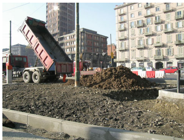
Fig. 10.3 Soil excavation, transport and re-distribution is typical of an urban setting
