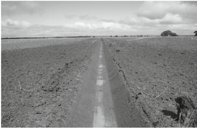
Fig. 6.17 Regular surface drains (Photo courtesy of TG Drains, Lake Road, Victoria)
