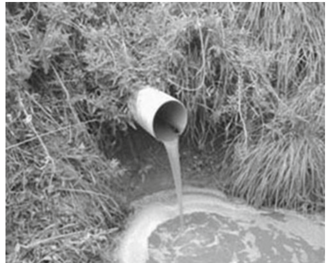
Fig. 6.19 Pipe drainage (Photo courtesy of USDA-NRCS)
