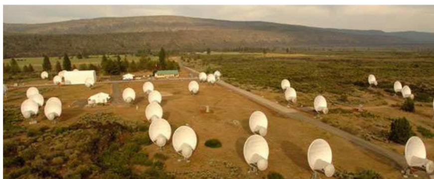
Fig. 7.3 Top: The 305 m radio telescope in Arecibo, Puerto Rico [13]. Bottom: The Allen telescope array in Hat Creek, California [14]
