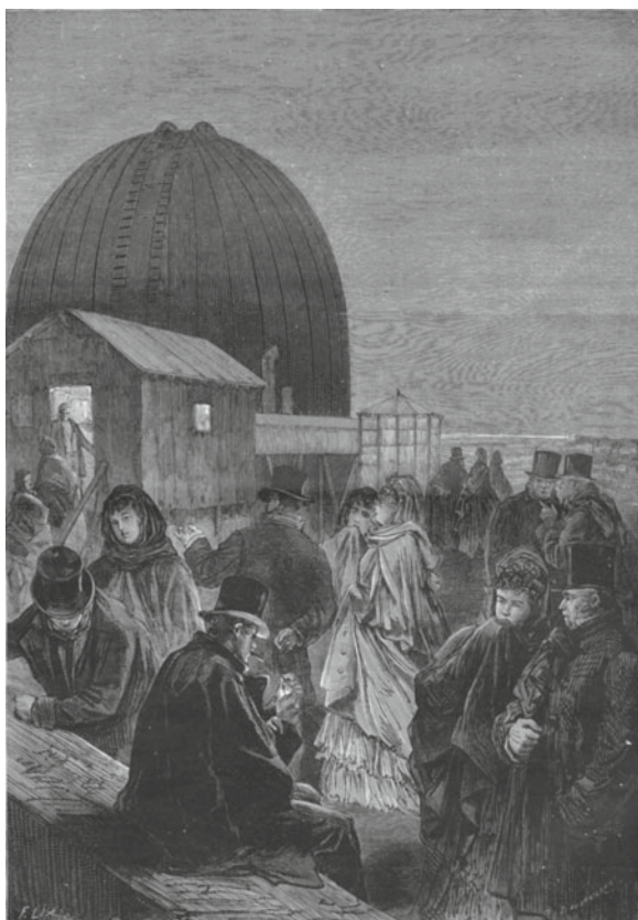
Fig. 5.17 Cornu's measurement in 1874 (external view). The provisional shelter on the terrace of the Observatory contains the principal station for measuring the velocity of light. The elongated part contains the tube of 38 cm equatorial, dismantled for the occasion. The light beam (in reality totally invisible) is sent to the Montlhéry tower, where a 15 cm aperture refractor with a mirror sends back the light to the Observatory. This experiment is the opportunity for a society gathering
