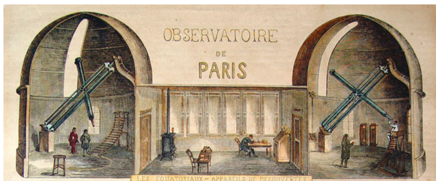
Fig. 4.16 Interior view of the twin domes in 1862. Given the dates, the drawing can only correspond to a project. The two 24-cm refractors have an English-type equatorial mount but it is not certain that it corresponds to reality. The twin domes still exist, the one to the East containing the equatorial of the Carte du Ciel , indeed with an English mount
