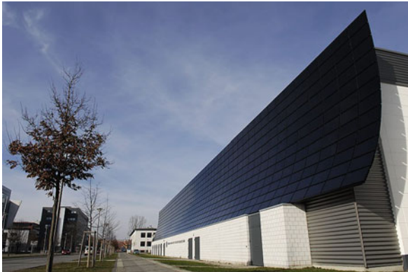
Fig. 8 Application of Sulfurcell BIPV modules
