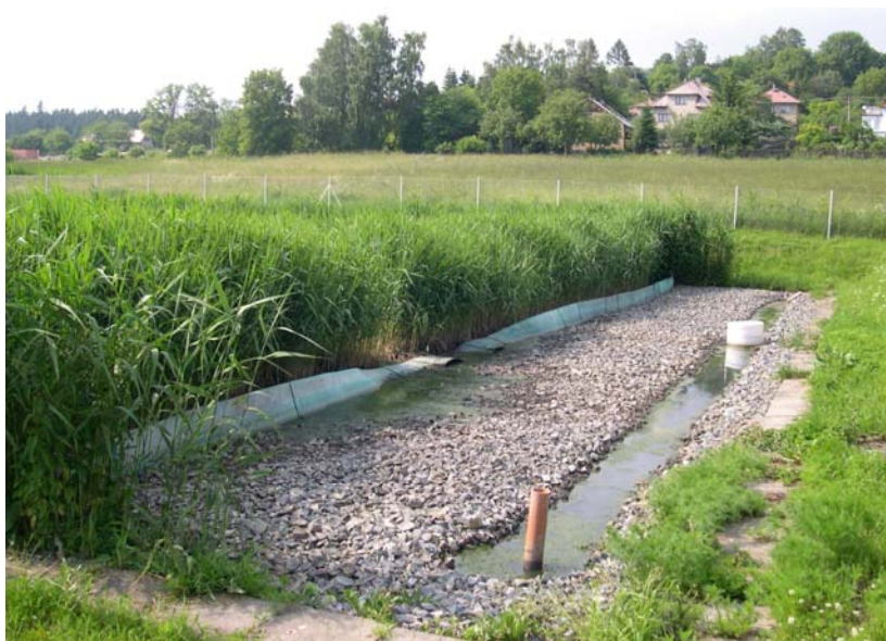
Figure 5-30. Deep zone distribution of wastewater in HF CW Ondřejov, Czech Republic. Photo by Jan Vymazal.
