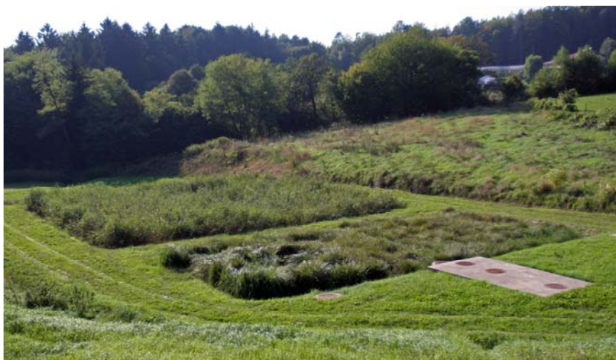
Figure 7-24. HF constructed wetlands for municipal sewage in Slovenia. Top: Ponikva, a 600 m 2 system built in 1992 (photo by Tjaša Griessler Bulc, with permission); middle: Velika Nedelja, a hybrid system consisting of HF bed (100 m 2 ), two VF beds (350 m 2 each), HF bed (100 m 2 ) and FWS pond (64 m 2 ) built in 2000 for 400 PE (photo by Tjaša Griessler Bulc, with permission); bottom: Sveti Tomaž, a 700 m 2 HF system with four beds for 250 PE built in 2001 (photo by Bogdan Macarol, with permission).
