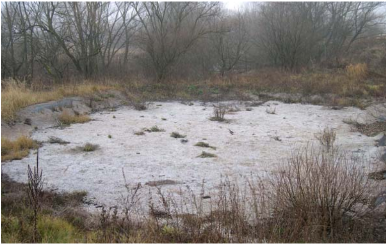
Figure 7-21. HF constructed wetland at Nálepkovo, East Slovakia (500 m 2 ) designed for tertiary treatment of dairy wastewaters. The system built in 1992 is currently out of operation because the dairy was closed down. Photo by Jan Vymazal.
