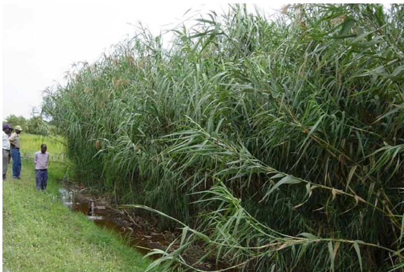
Figure 5-5. Constructed wetland at Kasese, planted with Phragmites mauritianus in Uganda treating effluent from cobalt recovery processing plant. Photo by Frank Kansime, with permission.
