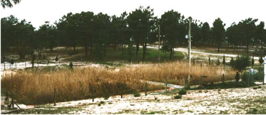
Figure 7-18. First full-scale HF constructed wetland for domestic wastewater in Portugal was built in Pinheiro da Cruz (200 PE, 578 m 2 ). Photo by Jan Vymazal.
