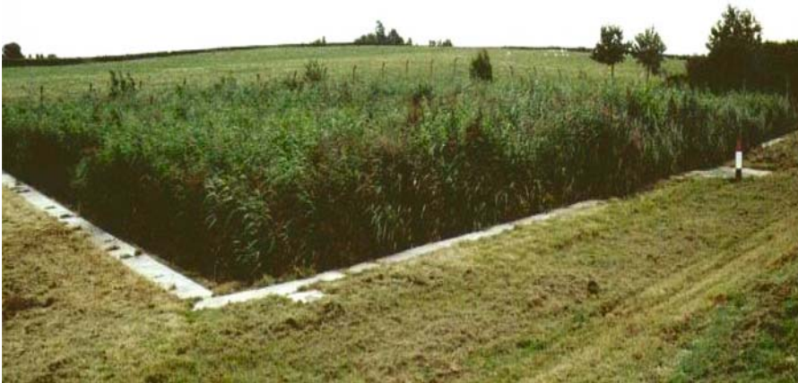
Figure 7-30. HF constructed wetland for tertiary treatment of municipal wastewater at Leek Wootton. Photo by Paul Cooper, with permission.
