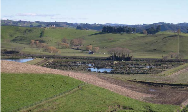
Figure 4-54. A 3 ha tertiary FWS-HF constructed wetland at Otorohanga, New Zealand. FWS part in front is planted with Eleocharis sphacelata and Scirpus tubernaemontani , HF part in the back is planted with Baumea articulata and Carex secta . Photo by Jan Vymazal.
