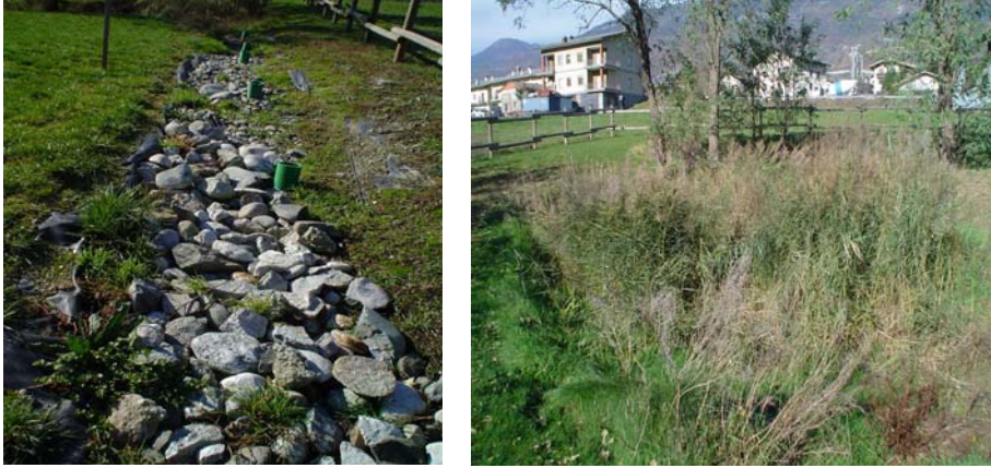
Figure 6-3. HF constructed wetlands for treatment of wastewaters from a cheese-making factory in Aosta Valley, north-west Italy Photos by Roberta Gorra, with permission.
