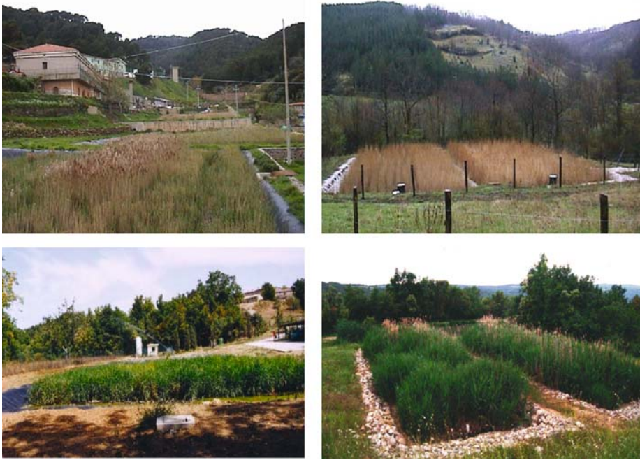
Figure 7-15. Four HF constructed wetlands in Tuscany, Italy. Top left: Gorgona Island, top right: Moscheta, Bottom left: Pentolina, bottom right: Spannocchia. For design details see Table 7-5. Photos by Fabio Masi, with permission of IRIDRA S.r.l.
