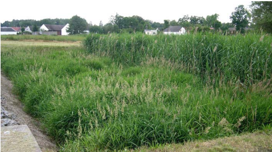
Figure 5-46. Top: HF constructed wetland Čejkovice, Czech Republic planted with Phalaris arundinacea as single species. Bottom: HF constructed wetland Příbraz, Czech Republic planted with Phalaris arundinacea (at left) and Phragmites australis in bands perpendicular to flow path. Photos by Lenka Kröpfelová.
