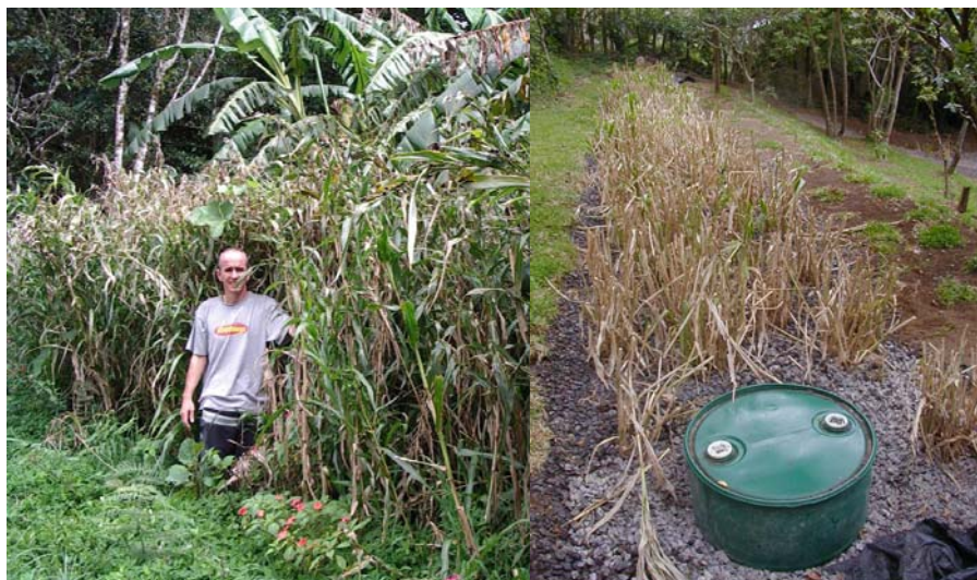
Figure 7-40. HF constructed wetland at Santa Elena-Monteverde, Costa Rica planted with a local plant Coix lacryma-jobi . Photo by Stewart Dallas, with permission.
