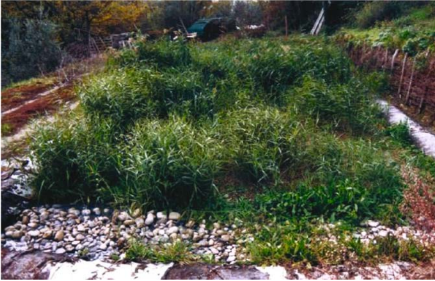
Figure 6-4. HF constructed wetland at Poggio Antico, Tuscany, Italy for the treatment of wastewaters produced during the organic farming activities. Photo by Fabio Masi with permission from IDRA S.r.l.
