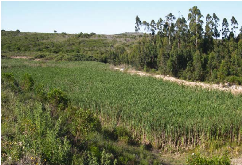
Figure 4-36. FWS constructed wetland planted with Typha domingensis for treatment of soft drink enterprise wastewaters NATIVA II in Uruguay. Photo by Jan Vymazal.
