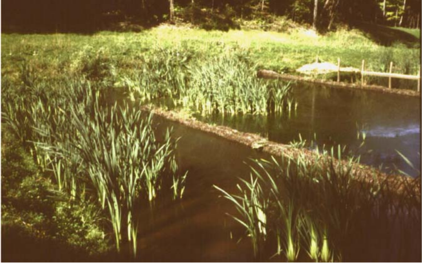
Figure 4-31. FWS constructed wetland for acid mine drainage in Lick Run, Ohio, USA. For details on performance see Mitsch and Wise (1998). Photo by Jan Vymazal.
