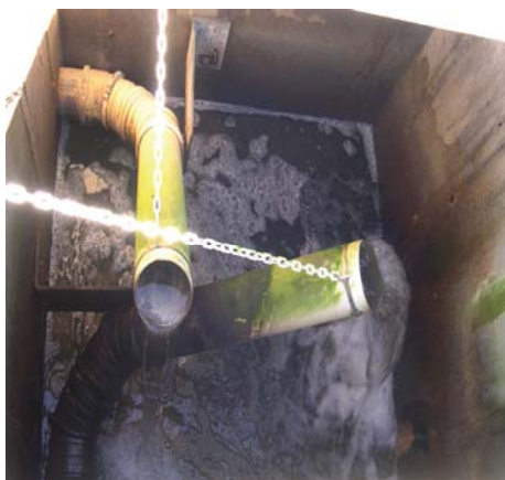
Figure 5-34. Swivelling elbows hanging on a chain in CW Sklené, Czech Republic(left) and Waikeria, New Zealand (right). Photos by Jan Vymazal.
