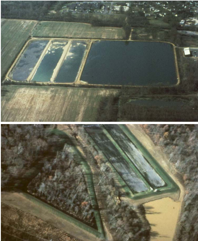
Figure 7-35. Tennessee Valley Authority demonstration HF constructed wetlands at Benton (top) and Hardin (bottom), Kentucky shortly after construction. Photo courtesy Jim Watson.
