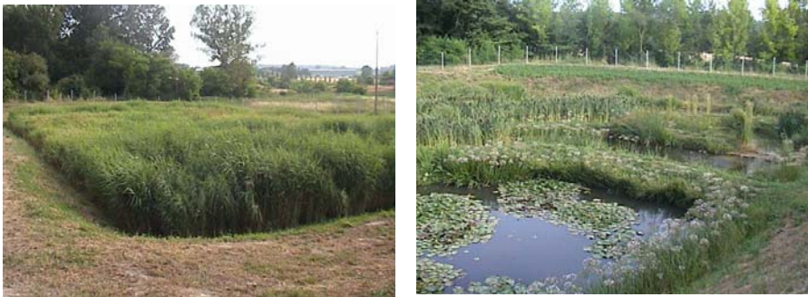
Figure 4-55. HF (450 m 2 ) - FWS (850 m 2 ) constructed wetland at Casa Vincicola, Cecchi, Italy. HF part is planted with Phragmites australis , FWS part is planted with dominance of Nymphaeae sp., Typha sp. and Juncus sp. Photos by Fabio Masi, with permission of IRIDRA S.r.l.
