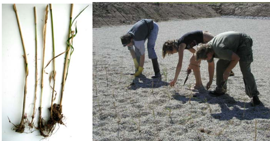
Figure 5-64. Bare-root seedlings of Phalaris arundinacea (left) and planting into a constructed wetland Libnič, Czech Republic. Photos by Lenka Kröpfelová.
