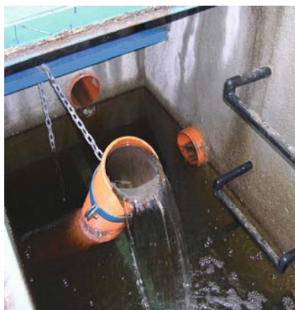
Figure 5-34. Swivelling elbows hanging on a chain in CW Sklené, Czech Republic(left) and Waikeria, New Zealand (right). Photos by Jan Vymazal.
