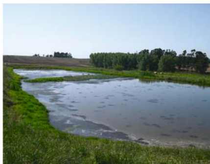
Figure 7-47. Anaerobic (left) and facultative anaerobic (right) lagoons as pretreatment units in HF constructed wetland San Jacinto treating meat processing enterprise wastewaters in Uruguay. For HW beds see Fig. 5-6. Photos by Jan Vymazal.
