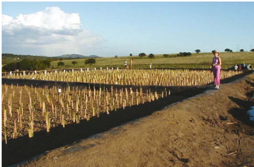
Figure 7-46. The first full scale HF constructed wetland in Uruguay (NATIVA I) designed for treatment of soft drink plant effluent. Photo by Silvana Perdomo, with permission.
