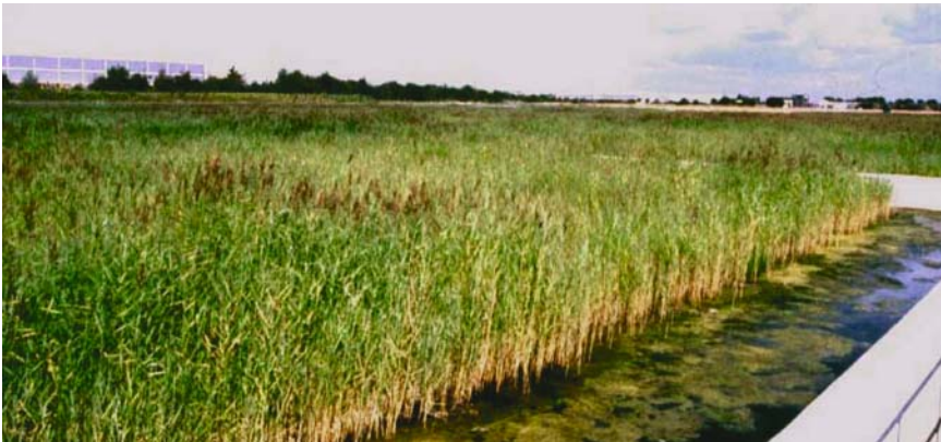
Figure 6-6. 2.08 ha HF constructed wetland as a part of the treatment system for runoff containing de-icing compounds at London Heathrow Airport. In front, there is an open water outflow zone. Photo by Jan Vymazal.
