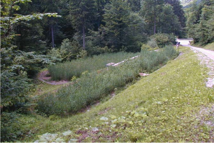
Figure 6-8. HF constructed wetland at Ljubevč, Slovenia for landfill leachate treatment. Two beds (150 and 125 m 2 ) are planted with Phragmites australis . Photo by Tjaša Bulc, with permission.
