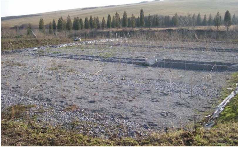
Figure 7-23. HF constructed wetland (700 PE, 1,500 m 2 ) for tertiary treatment of municipal sewage at Krásna Lúka, East Slovakia. Photo by Jan Vymazal.
