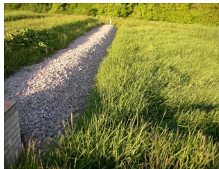
Figure 5-28. Distribution pipe laid down on the surface and overlaid by large stones. HF CW Mořina, Czech Republic. Left: March 2006 before plants start to sprout, right: May 2006. Photos by Jan Vymazal.
