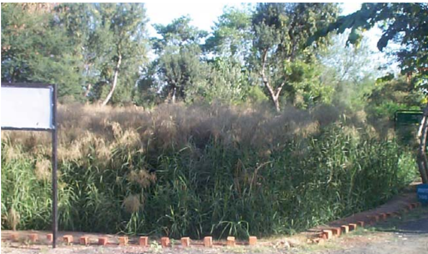
Figure 7-53. A 750 m 2 HF constructed wetland planted with Phragmites karka in Ekant Park (Bhopal) built in 2002. Daily flow 80 m 3 d -1 . Photo by Suresh Billore, with permission.
