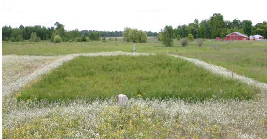
Figure 7-38. HF constructed wetland Morton Farm Preserve, Minnesota for 90 PE. Photo by Scott Wallace, with permission.
