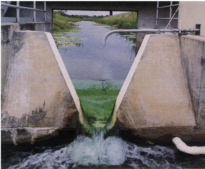
Figure 4-21. The H-flume structure for the outflow control from Lakeland FWS constructed wetland in Florida. From U.S. EPA (1993), with permission.
