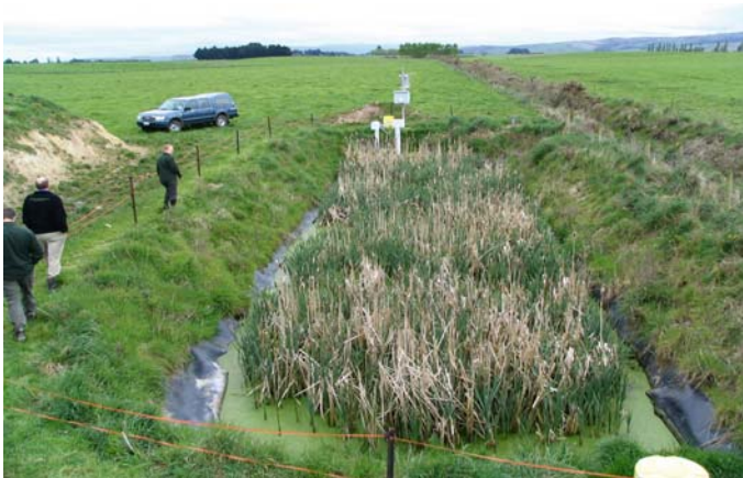
Figure 4-29. FWS constructed wetland (90 m 2 ) for removal of nitrate from a 1.7 ha pasture at Bog Burn, New Zealand (South Island). Photo by Chris Tanner, with permission.
