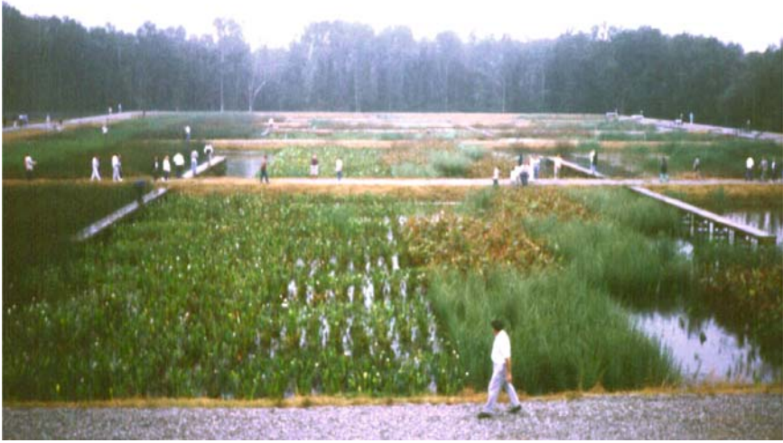
Figure 4-33. FWS constructed wetland for secondary treatment effluent from bleached kraft mill in Pensacola, Florida. (Details on performance in Knight et al., 1994). Photo by Jan Vymazal.
