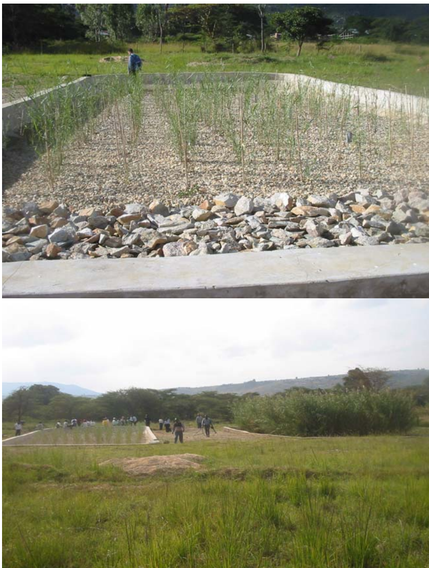
Figure 7-51. HF constructed wetland treating wastewaters from the Ruaha Secondary School in Iringa, Tanzania. Photos by Richard Kimwaga, with permission.
