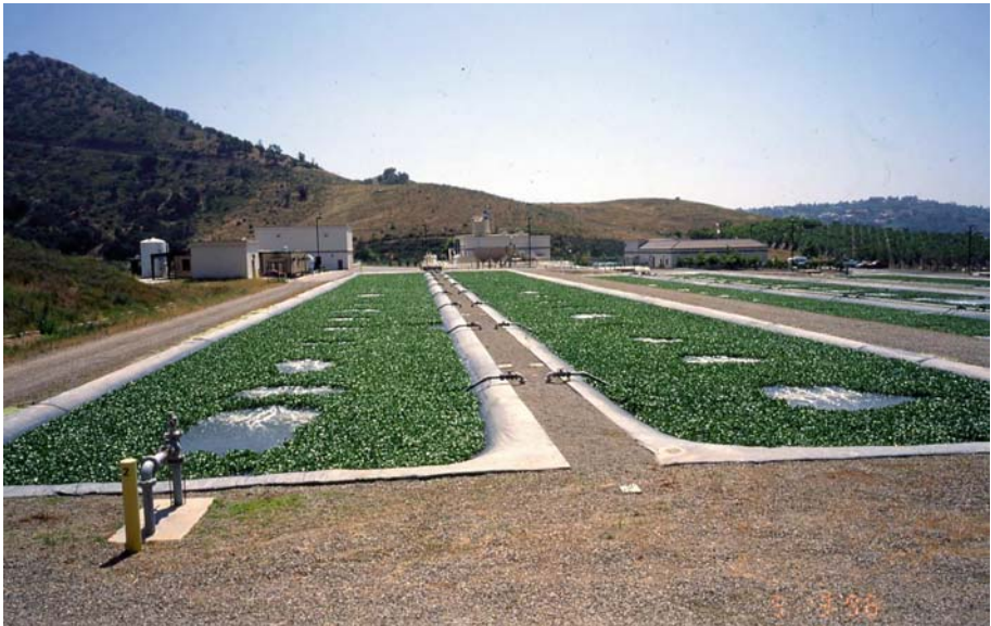
Figure 4-4. Constructed wetland with Water hyacinth Aqua III in San Diego, California, USA. Photo by George Tchobanoglous, with permission.
