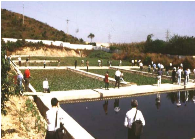
Figure 4-53. FWS-HF hybrid constructed wetlands at Yantian Industry Area in Baoan District, Shengzhen City. The system consists of up flow pond (247 m 2 ), three FWS cells (275 m 2 each) with Eichhornia crassipes and two HF beds (805 m 2 each) planted with Phragmites australis . Photo by Jan Vymazal.
