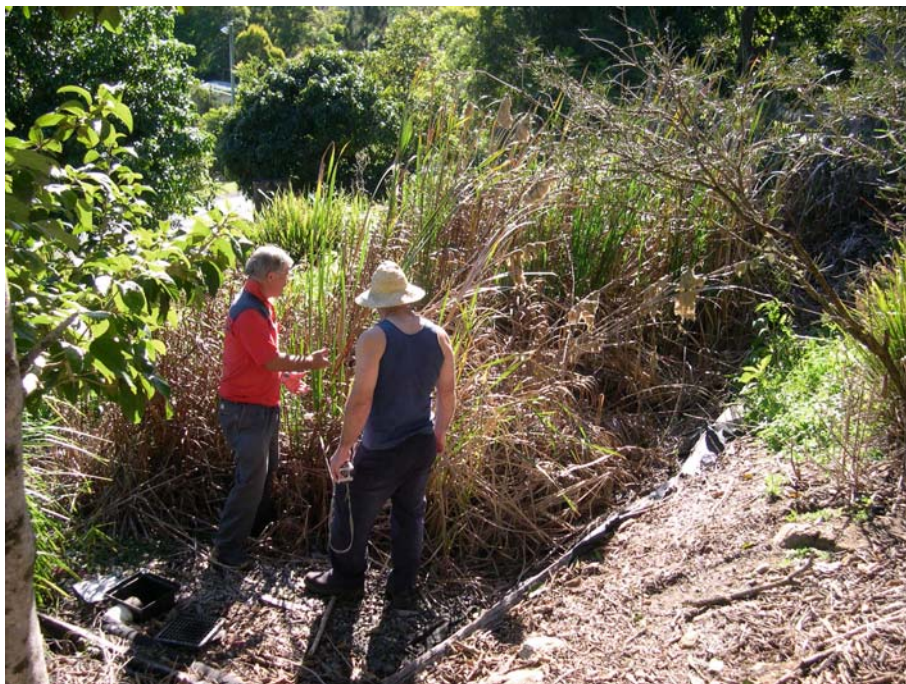
Figure 7-48. HF constructed wetland at The Channon treating wastewaters from a laundry. The bed is planted with a mixture of Typha orientalis (Cattail) and Bolboschoenus fluviatilis (Marsh clubrush). Photo by Jan Vymazal.
