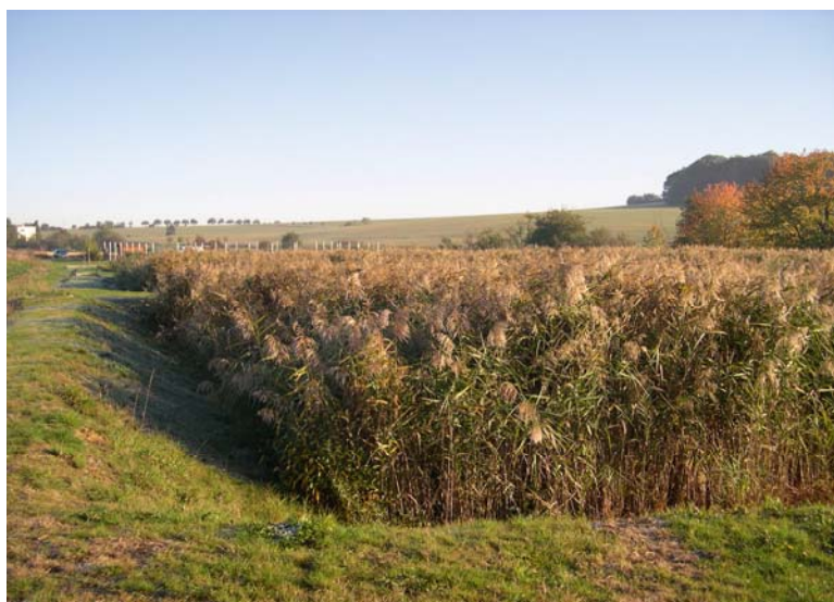
Figure 5-40. HF constructed wetland Machová in the Czech Republic planted with Phragmites australis . Photo by Lenka Kröpfelová.
