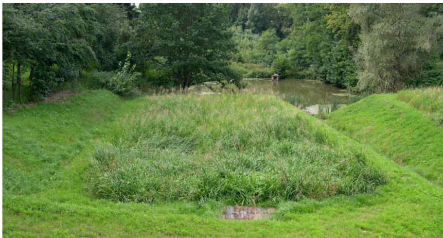
Figure 5-53. HF constructed wetland Sedlce, Czech Republic planted with Glyceria maxima . For detail see Fig. 5-51. Photo by Lenka Kröpfelová.
