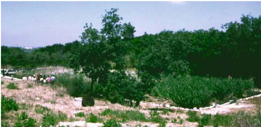
Figure 7-19. Constructed wetlands (VF-HF-pond) in Alcanadas, Portugal designed for landfill leachate treatment. Photo by Jan Vymazal.
