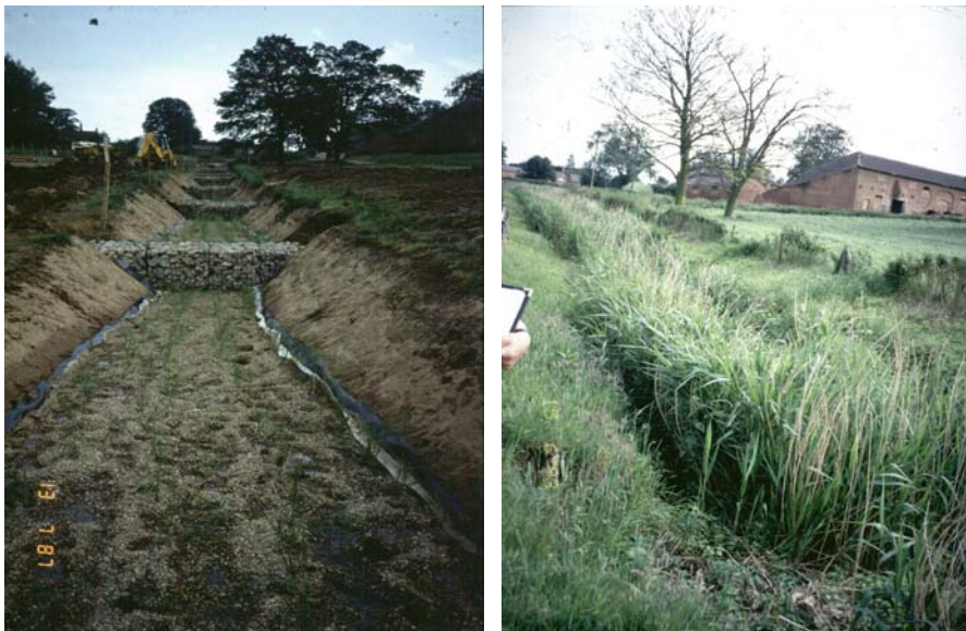
Figure 7-28. HF constructed wetland at Little Stretton, Leicestershire, United Kingdom in July 1987 (left) and November 1987 (right). Photos by Paul Cooper, with permission.
