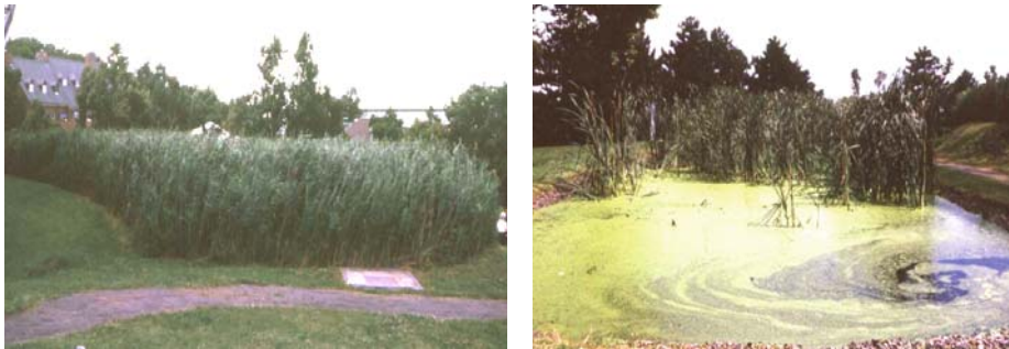
Figure 4-56. HF-FWS constructed wetland in Biosphère de Montréal, Canada. Left: HF stage, Right: FWS stage. Photos by Jan Vymazal.
