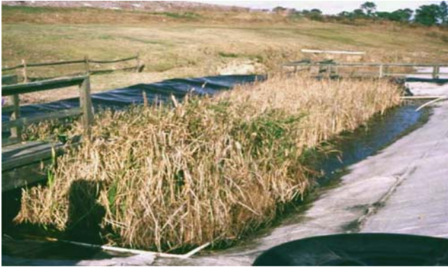
Figure 7-39. Pilot-scale (71.7 m 2 ) HF constructed wetland for landfill leachate at the New Hanover County landfill, North Carolina, U.S.A. Photo by Jan Vymazal.
