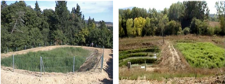
Figure 6-5. HF constructed wetland Azienda Agricola La Croche (left) and HF-FWS hybrid constructed wetland Casa Vinicola Luigi Cecchi and Sons (right), both Castellina in Chianti-Siena, Italy, for treatment of winery wastewaters. Photos by Fabio Masi with permission from IRIDRA S.r.l.
