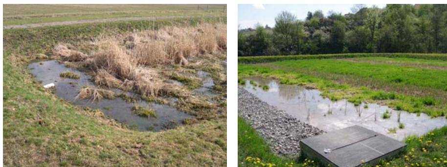
Figure 5-21. Surfacing (ponding) of wastewater in the inlet zone of HF constructed wetlands Břehov (left) and Mořina (right), Czech Republic. Photo by Lenka Kröpfelová.
