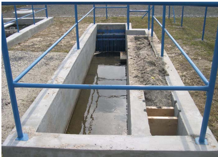
Figure 5-13. Horizontal flow grit chamber with side grit compartment. CW Sklené, Czech Republic. Photo by Lenka Kröpfelová.
