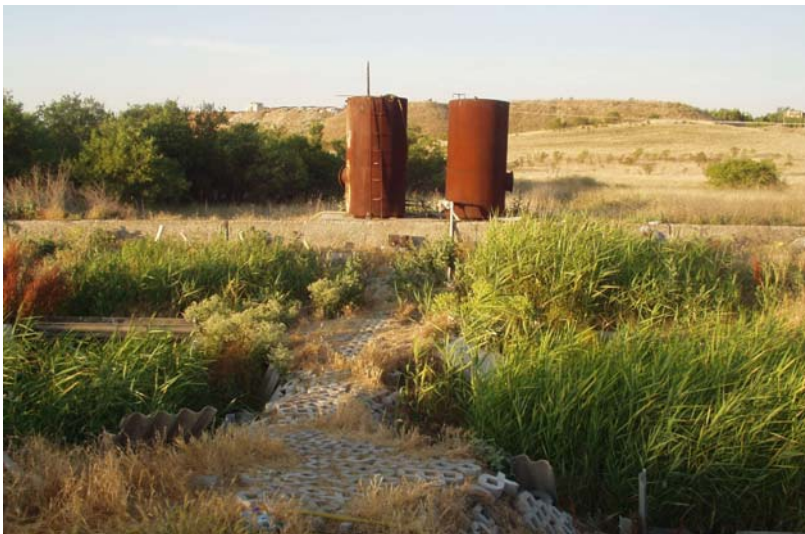
Figure 7-56. Pilot-scale VF-HF constructed wetland at the Middle East Technical University in Ankara, Turkey. Photo by Asuman Korkusuz, with permission.
