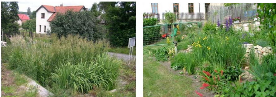
Figure 7-5. HF constructed wetlands for a single house wastewater treatment. Left: Kyjov (4 PE), right: Žitenice (6 PE). Photos by Jan Vymazal.
