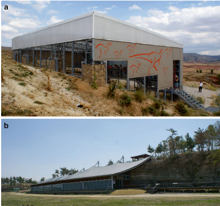
Fig. 4.6 Protection measures for dinosaur footprint sites (tracksites); all these photographs are reproduced with kind permission of Daniel Marty. (a) Early Cretaceous Las Cerradicas sauropod and ornithopod tracksite (Pérez-Lorente et al. 1997; Castanera et al. 2011) in Spain (Galve, Teruel Province) was protected by the construction of a metallic building as part of the Dinosaur Ichnites of the Iberian Peninsula Project (IDPI). This building is, however, not entirely closed and the site is still exposed to a certain degree of weathering. (b) Late Cretaceous Unhangri dinosaur, pterosaur, and bird tracksite (Lee and Huh 2002; Hwang et al. 2002, 2008) in South Korea (Haenam-gun County, South Jeolla Province, Natural Monument 394). This picture shows the building that protects the palaeosurface with pterosaur tracks shown in Fig. 4.5c
