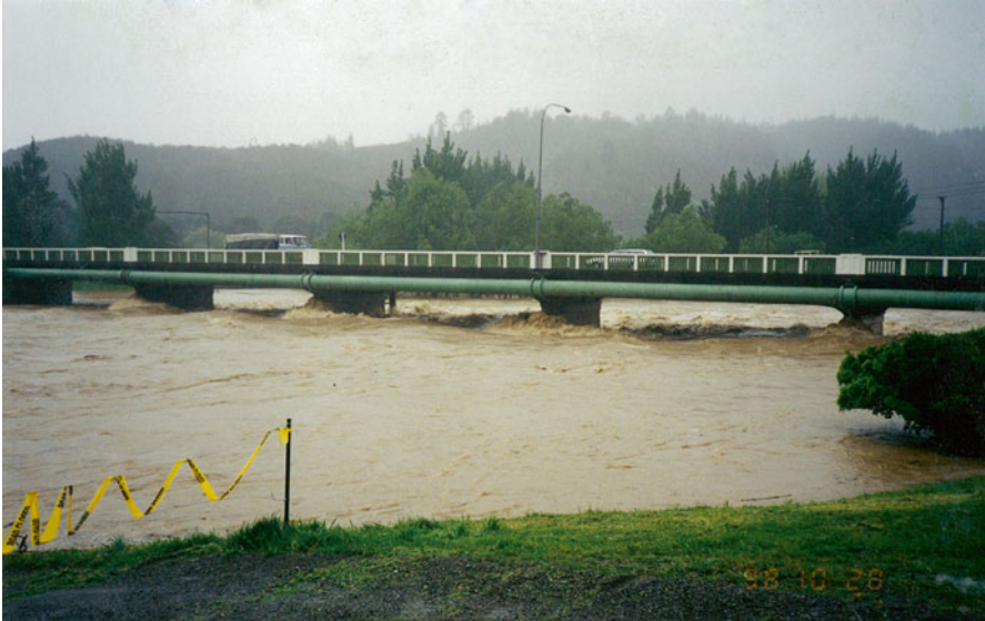
Fig. 4.30 Flooding of the Hutt river
