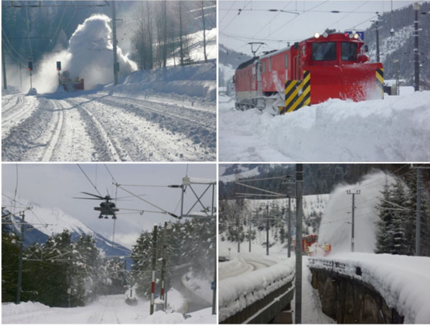
Fig. 4.24 Winter service ÖBB – West part of Austria in January 2012 (Photos: ÖBB)
