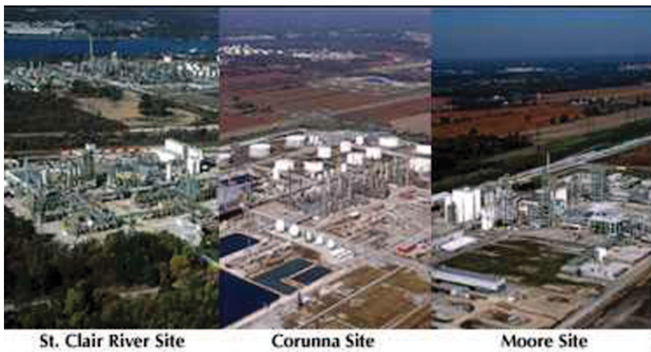
Fig. 9.5 Nova Chemicals Sarnia-Lambton operations. (Courtesy Nova Chemicals)
