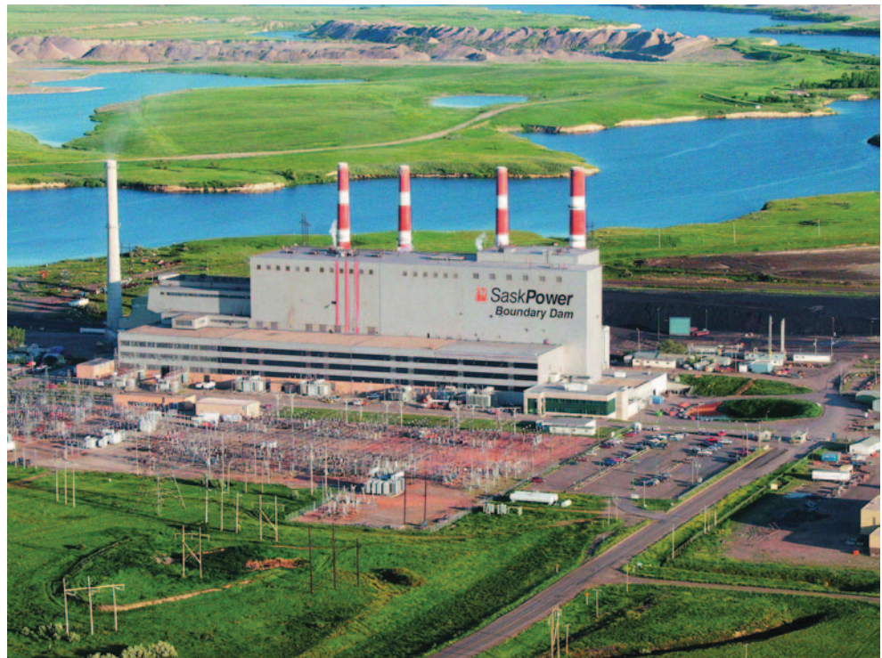
Fig. 9.7 Boundary dam power station near Estevan, Saskatchewan. (Photo provided by and property of SaskPower)
