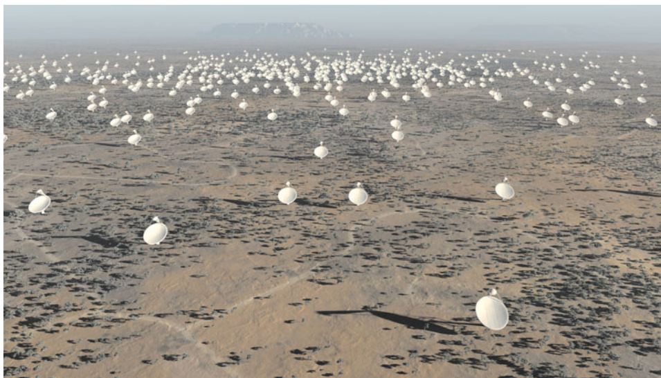
Figure 8.13 Artist's impression of the 15 meter \times 12 meter offset Gregorian antennas within the central core of the Square Kilometer Array (SKA). Dish antennas like these will form a substantial part of the SKA; around 3,000 dishes are currently planned. Many aspects of the SKA dish design are without precedent, not only because of the large numbers of dishes required, but also because of the huge sensitivity that will result (SPDO/TDP/DRAO/Swinburne Astronomy Productions).
