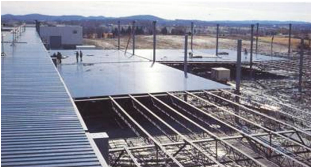
Fig. 12.6 Raised-roof construction
