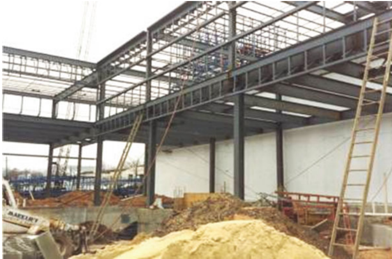
Fig. 12.5 Steel frame and brick construction
