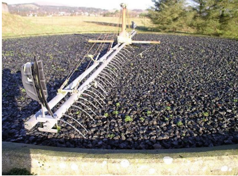
Fig. 18.8 Typical percolating (trickling) filter
