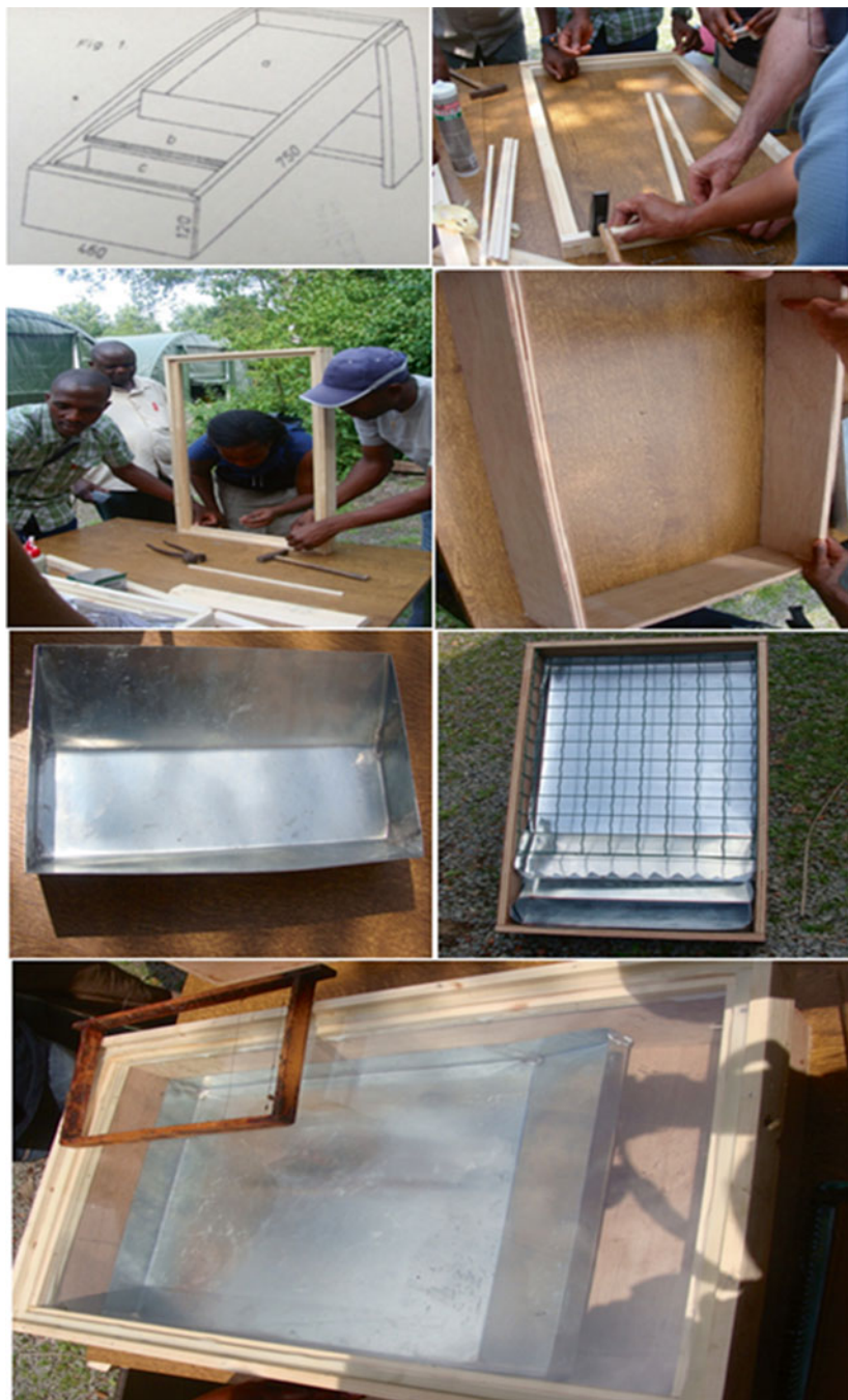
Fig. 21.8 Making your own solar wax melter
