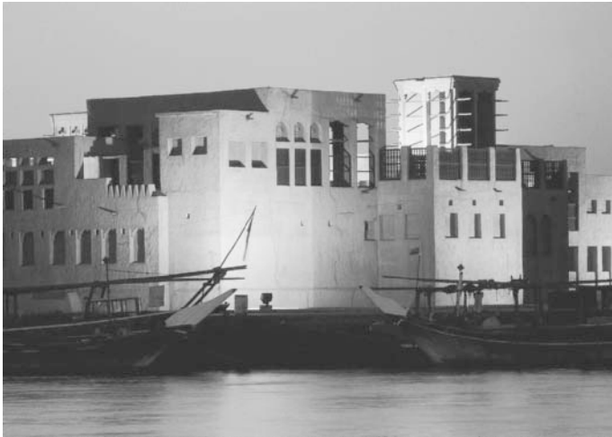
FIGURE 5.9 | Dubai's heritage in the Bastaqya and Shindagha area (H.H. Sheikh Saeed's house)
