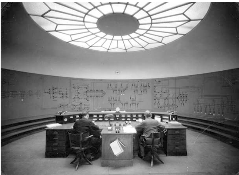
Figure 8.3 The dispatchers at the control center of the Norwegian Power Pool in the 1930s. Source: Statnett. Used by permission.
