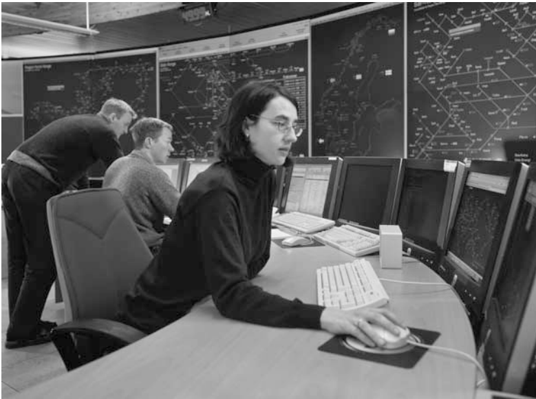
Figure 8.4 Statnett’s national control center coordinates the operations of all players involved in the Norwegian main grid with its international connections.
