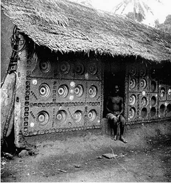
2.5 House with inset plates in the wall. Ikwerri, Southeastern Nigeria, 1930s
