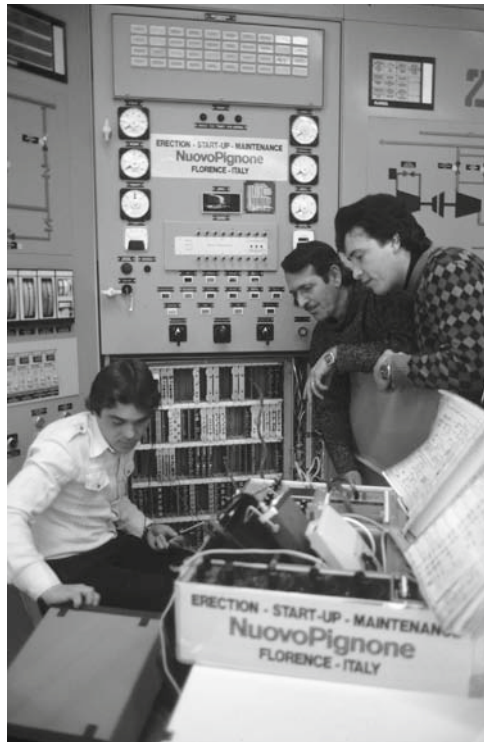
Figure 11.1 Italian technicians from Nuovo Pignone adjusting electronic equipment at one of the new compressor stations along the Yamal (Urengoi-Uzhgorod) pipeline.
