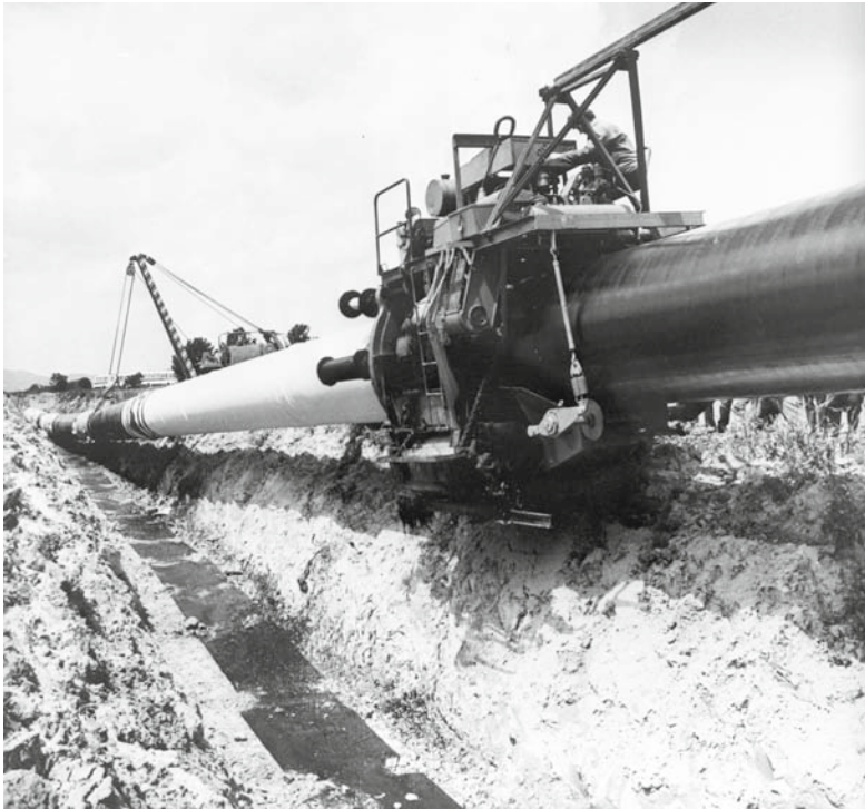
Figure 9.1 Construction of the first transit pipeline through Czechoslovakia, July 1971.
