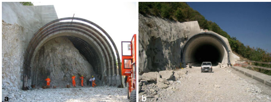
Fig. 2.7 Tunnel portal affecting the slope obliquely: in this case, stabilization structures were: a placement of tie rods on a reinforced concrete head-beam and a steel ribs-reinforced portal, b completion of the reinforced concrete structure. (By Pizzarotti)
