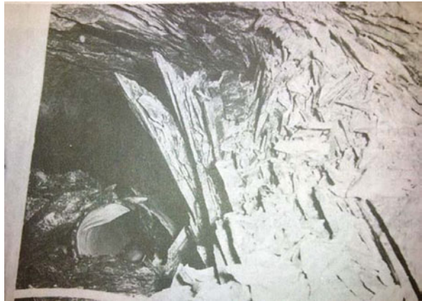
Fig. 1.2 Collapse under severe rock-burst conditions. (Hoek and Brown 1980)
