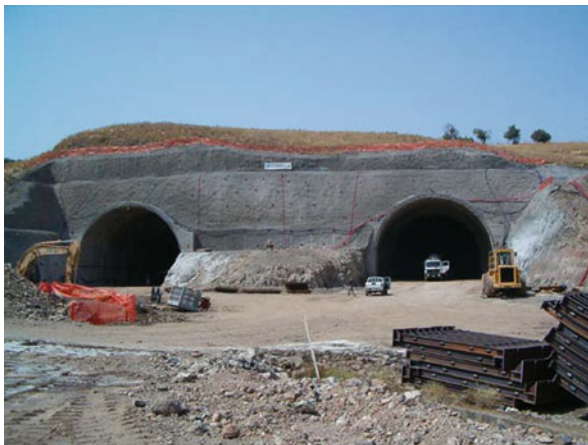
Fig. 1.17 An example of a tunnel portal with nailing of the slope. (By Pizzarotti)
