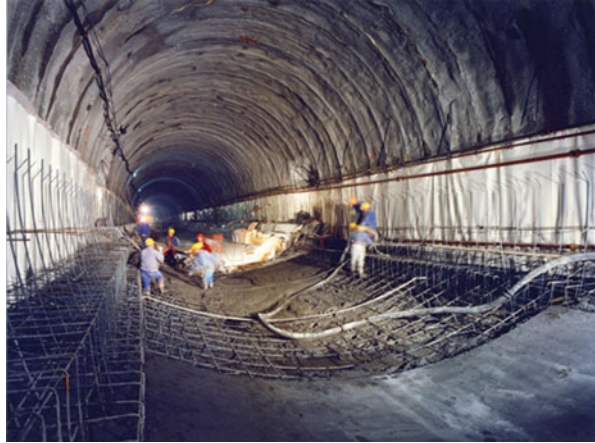
Fig. 6.56 Casting phase of the invert. (By Pizzarotti)
