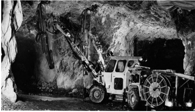
Fig. 6.29 Drilling with jumbo to install nails in the crown. (By Atlas Copco)
