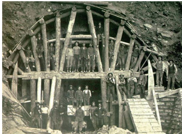
Fig. 6.2 South ramp of the Lötschberg tunnel: execution of the portal in loose soil, about 1910. (Kovari and Fechtig 1996)
