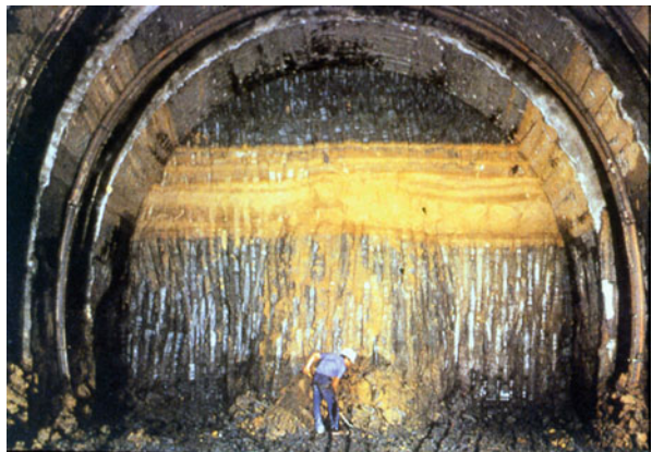
Fig. 6.46 Tunnel excavated with precutting method. (By Rodio)
