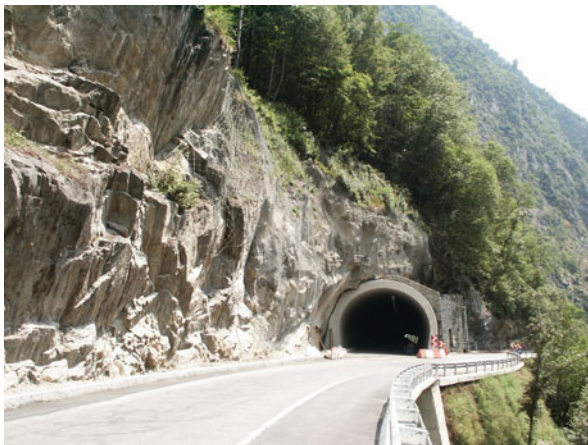
Fig. 1.14 An example of a shallow tunnel along the side of a valley. (By Pizzarotti)
