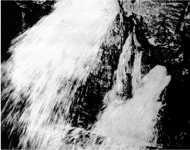
Fig. 1.21 An example of water inflow in the Simplon tunnel (historical photo)
