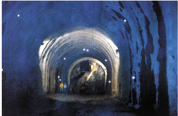
Fig. 8.4 Optical targets. (by Pizzarotti)
