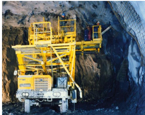
Fig. 6.29 Drilling with jumbo to install nails in the crown. (By Atlas Copco)
