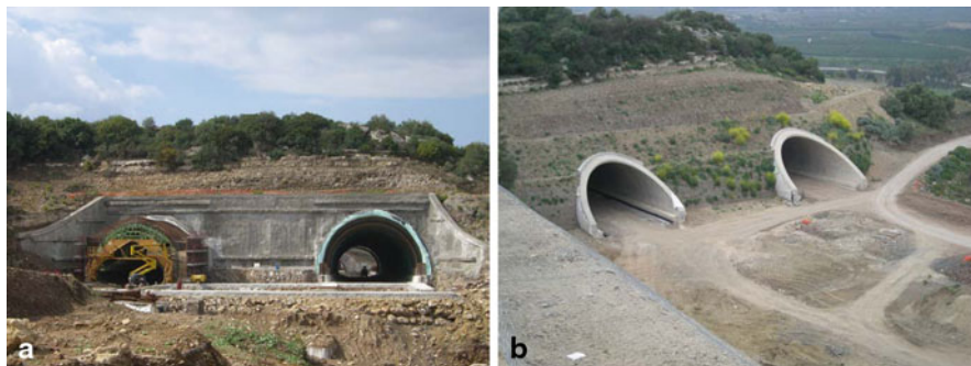
Fig. 1.18 Stabilization of a tunnel portal by retaining walls with anchors a during construction, b final configuration. (By Pizzarotti)
