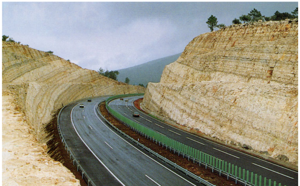
Fig. 1.3 Motorway A1. Solution open excavation
