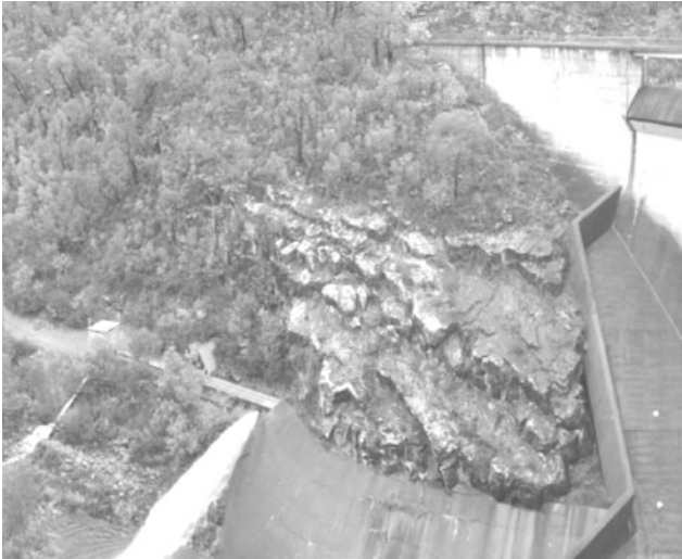
Fig. 38.3 Right abutment of arch dam with variably bedded quartzite mass that required stability assessment
