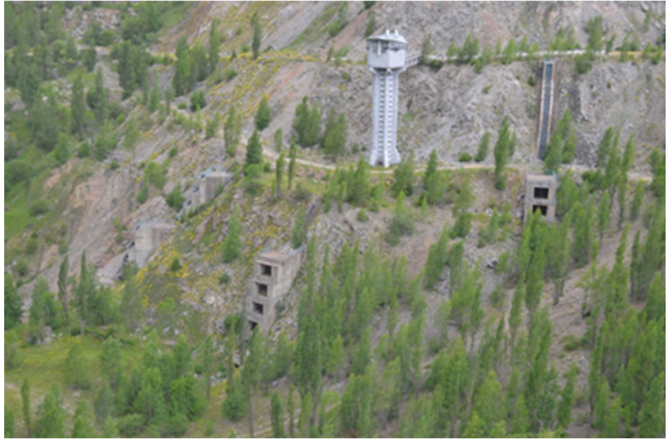
Fig. 50.8 Medeo dam mud-flow reservoir. The system of water outlets, young forest at the dam's slope, July 2013. Photo by A. Koshkin
