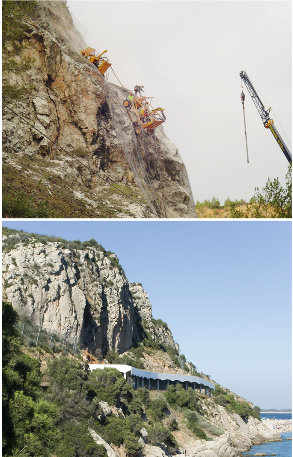
Fig. 1.5 Serra da Arrábida. Retaining works and false tunnel
