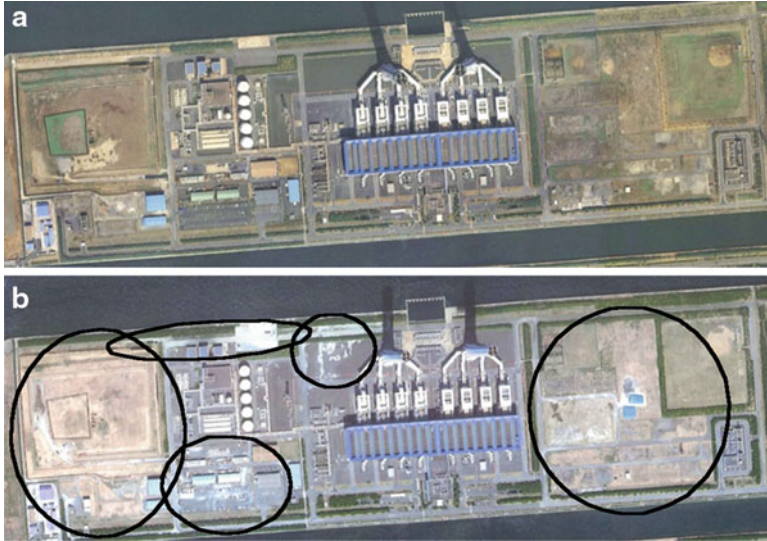
Fig. 1.97 Soil liquefaction in power plant around the Tokyo Bay (2011 Tohoku earthquake). (a) Before the earthquake (2009.10.16). (b) After the earthquake (2011.3.31) (identification of liquefaction traces by aerial photographs, circles show the traces of the sand boiling)
