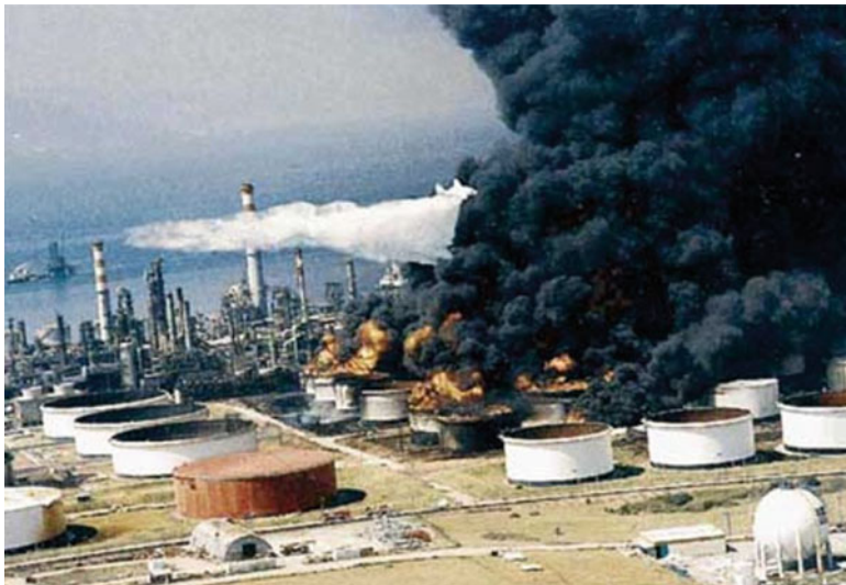
Fig. 1.11 Fire of tanks by long-period component of earthquake ground motion (1999 Kocaeli earthquake, Turkey, at Tüpraş oil refinery)
