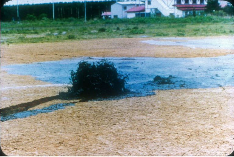
Fig. 3.1 Sand and water boiling due to soil liquefaction (1983 Central Japan Sea earthquake) [1]
