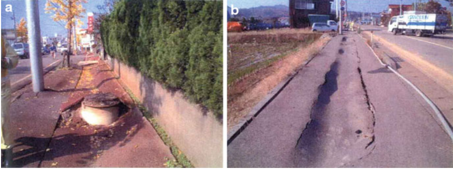
Fig. 1.74 Damage to buried sewage pipes (2004 Niigata-Chuetsu earthquake). (a) Uplift of a manhole by liquefaction of backfilling soil (at Nagaoko). (b) Subsidence of ground surface by liquefaction of backfilling soil (at Ojiya)
