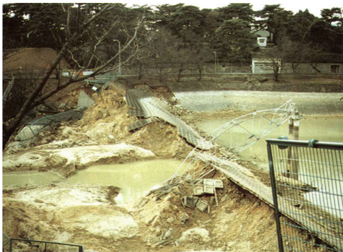
Fig. 2.25 Slide and sinkage of Niteko earth dam (1995 Kobe earthquake)
