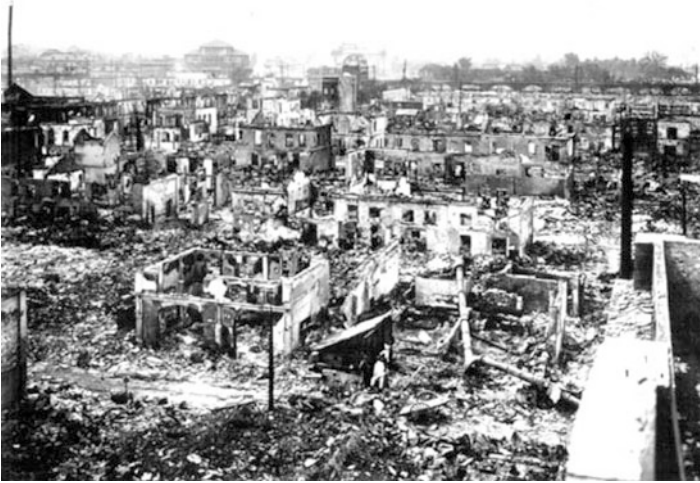
Fig. 2.2 Damage to modernistic buildings by 1923 Kanto earthquake (home page of the National Science Museum)
