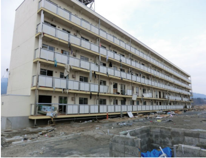
Fig. 1.95 Five story concrete building survived from the tsunami (2011 Tohoku earthquake, at Rikuzen-Takada)
