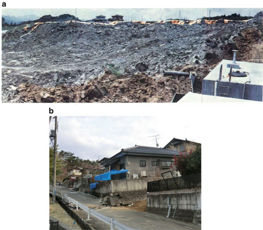
Fig. 6.12 Slope failures of residential areas. (a) 1978 Miyagi prefecture offshore earthquake (Shiroishi city). (b) 2011 Tohoku earthquake (Sendai city)
