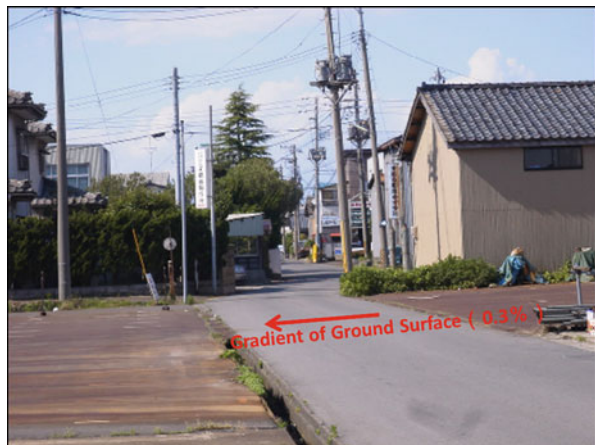
Fig. 4.32 Curved road by liquefaction-induced ground displacements (1964 Niigata earthquake)
