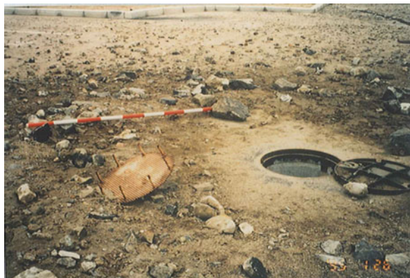
Fig. 3.4 Gravels boiled out of ground due to liquefaction (1995 Kobe earthquake)
