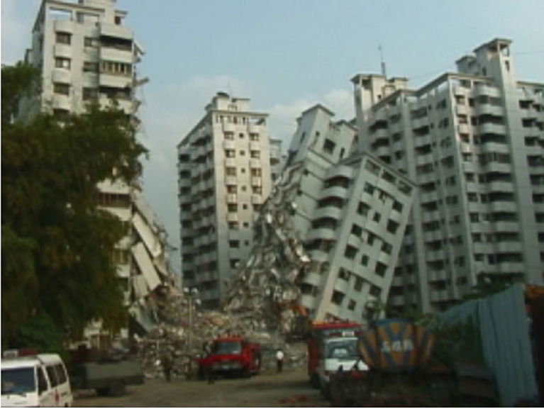
Fig. 1.22 Collapse of reinforced concrete buildings caused by strong ground motion (1999 Chi-Chi earthquake, Taiwan)
