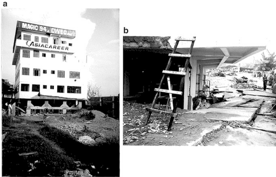
Fig. 6.37 Subsided and inclined concrete building with five stories due to soil liquefaction (1990 Ruzon island earthquake, Phillipines, at Dugupan). (a) Damaged building. (b) Subsidence and inclination (Max. subsidence: 1.5 m, inclination 3^\circ )
