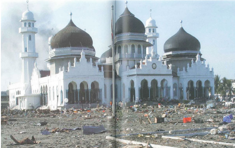
Fig. 1.35 Mosque survived from the tsunami (2004 Sumatra offshore earthquake and tsunami, at Banda Aceh)
