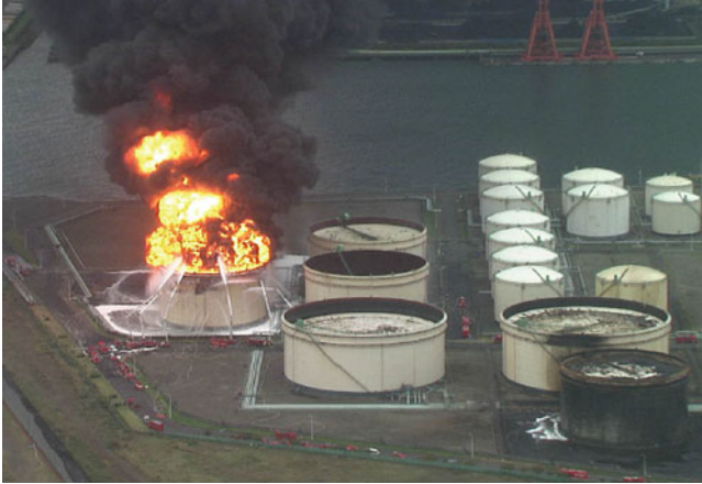
Fig. 1.67 Fire of oil tanks (2003 Tokachi offshore earthquake, at Tomakomai, after Kyodo Tsushin)
