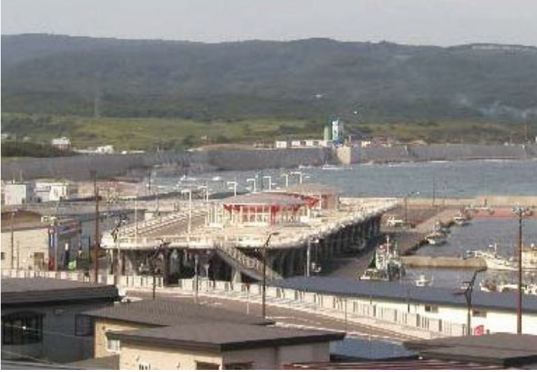
Fig. 1.53 Shelter terrace constructed after the tsunami
