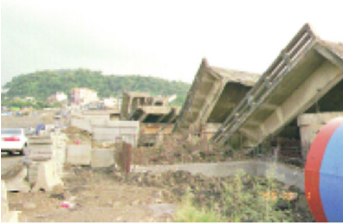
Fig. 1.18 Collapse of Yi-Jiang bridge crossing earthquake fault (1999 Chi-Chi earthquake, Taiwan)
