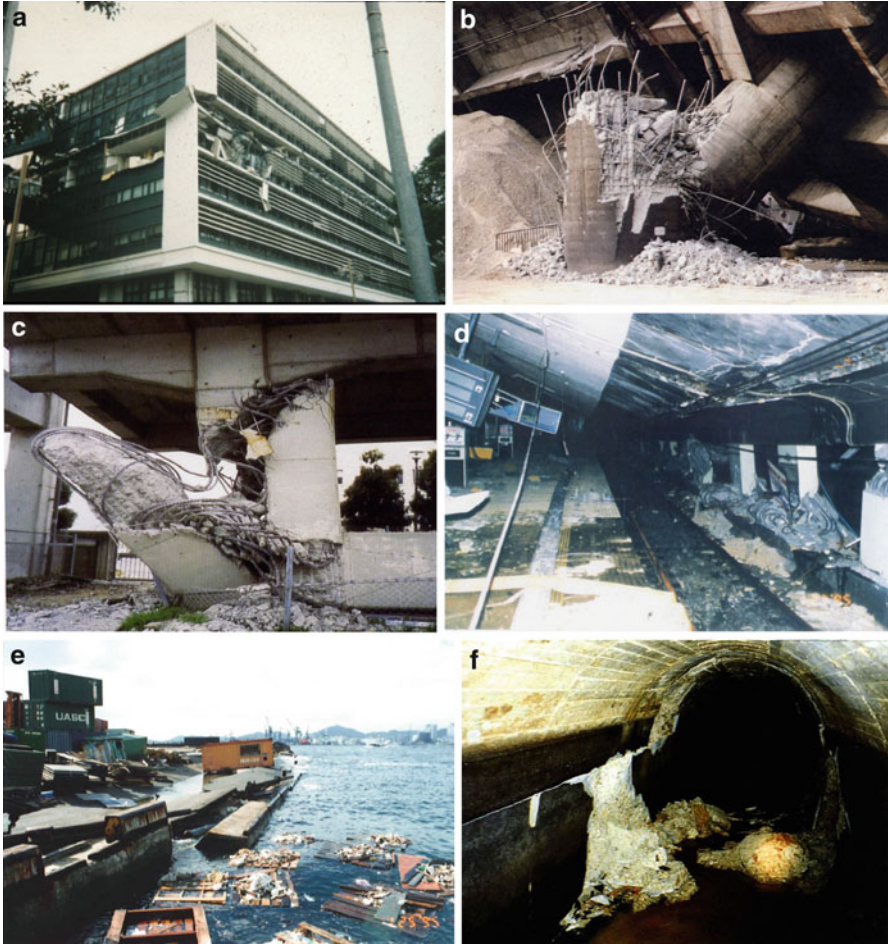
Fig. 1.61 Damage to building, road, railway, subway and tunnel (1995 Kobe earthquake, Japan). (a) Collapse of a building. (b) Shear failure of concrete pier of road bridge. (c) Shear failure of concrete column of railway bridge. (d) Shear failure of columns of subway. (e) Large inclination of quay wall. (f) Damage to a tunnel for water transmission
