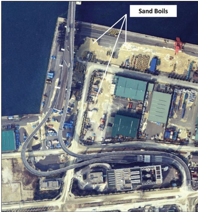
Fig. 4.91 Sand boils around a highway bridge (1995 Kobe earthquake at Rokko island in Kobe)
