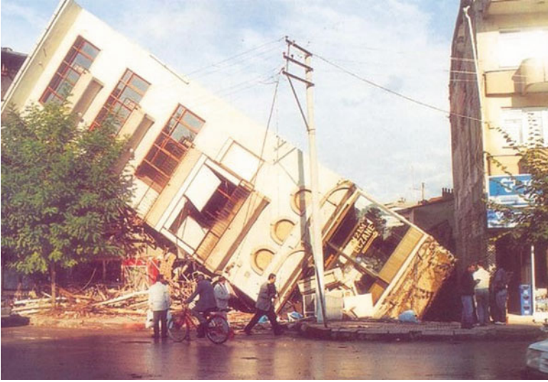
Fig. 1.12 Collapse of a building due to soil liquefaction (1999 Kocaeli earthquake, Turkey, at Adapazarı)
