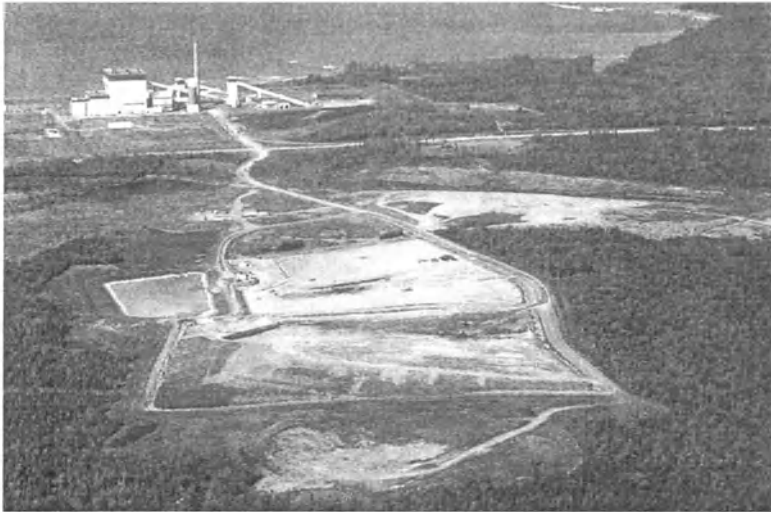
Fig. 1. Point Aconi Generating Station (Cape Breton, Nova Scotia) in the background, with the residue landfill site in the foreground.
