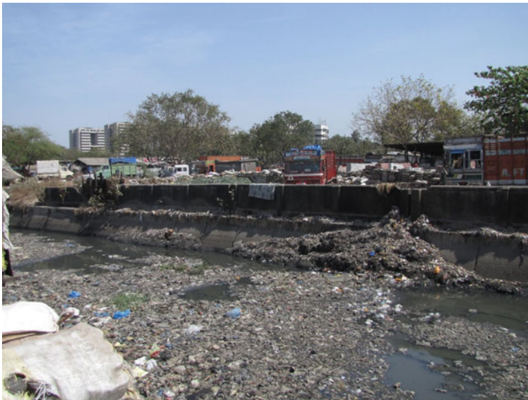
Fig. 5.11 Open sewer in Dharavi slum, Mumbai, India: Garbage has been dumped and is accumulating in open sewers close to residences. Sludge accumulates in low areas and gives rise to foul odors
