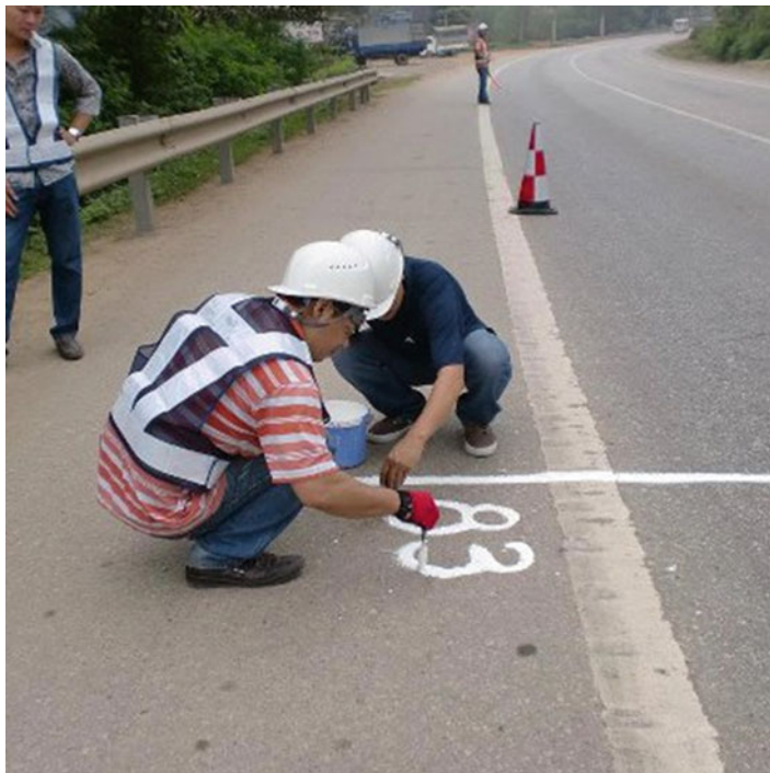
Fig. 7.5 Checking kilo-posts with Vietnamese engineers
