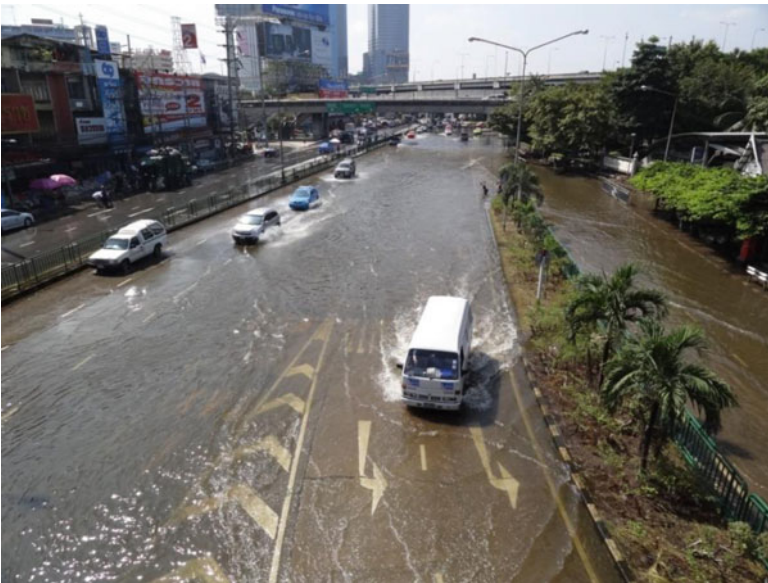
Fig. 3.10 Flooding around the Bangkok subway Phaholyothin station, 2011
