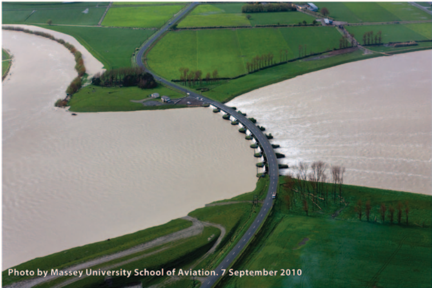
Fig. 10.2 The Motua sluice gates and spillway. (Source: Photograph by Massey University School of Aviation and sourced from Horizons Regional Council)
