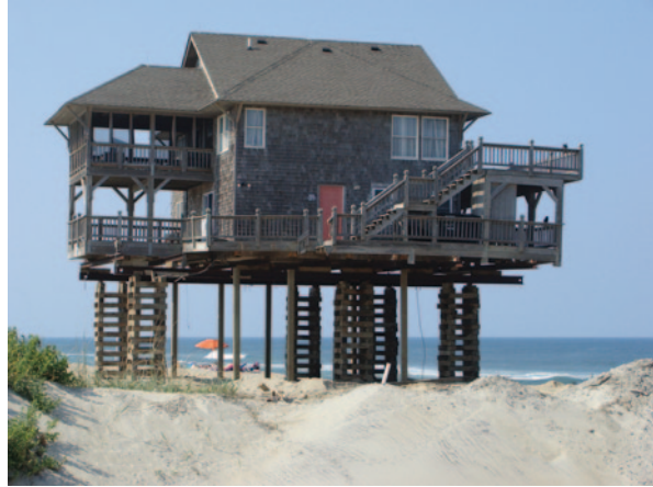
Fig. 9.5 Home elevation project on the Outer Banks of North Carolina. The image demonstrates the extreme measures individual property owners will take in an effort to protect their investment including elevating their home on a highly dynamic barrier island in front of what remains of a protective coastal dune. (Source: Photograph by Gavin Smith)
