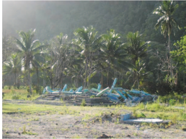
Fig. 13.2 Example of typical damage to houses along the south coast of Upolu as a result of the September 2009 tsunami (photo taken March 2010). (Source: Photograph Michele Daly)
