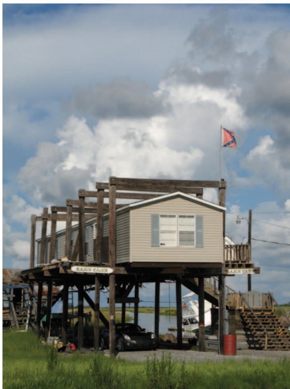
Fig. 15.7 Mitigation measures, Grand Isle, Louisiana. (Source: photograph by Bruce Glavovic)
