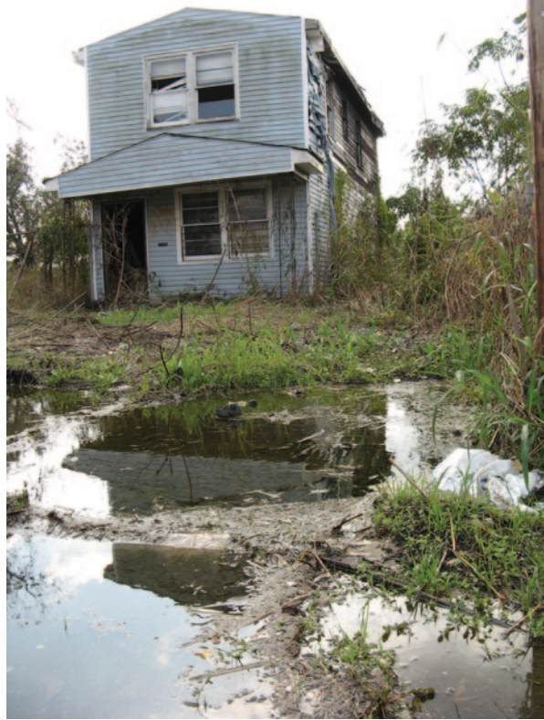
Fig. 15.3 Derelict house, Lower 9th Ward, New Orleans. (Source: photograph by Bruce Glavovic)
