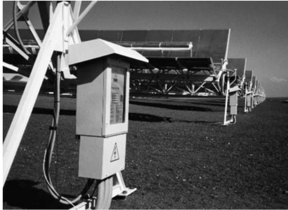
coordinates employed are not matched with the real tracking axes employed, such as for example would happen if providing horizontal Az.-El. coordinates to a two axis Tilt-Roll tracker. Some scanning scheme is used by the tracking axes to obtain some precise sun pointing and the correct axes turning angles from which to obtain tracking error measurements, which are then to enter the box labelled error forecasting, which produces corrections to be added to the next “raw” sun ephemeris coordinates.
