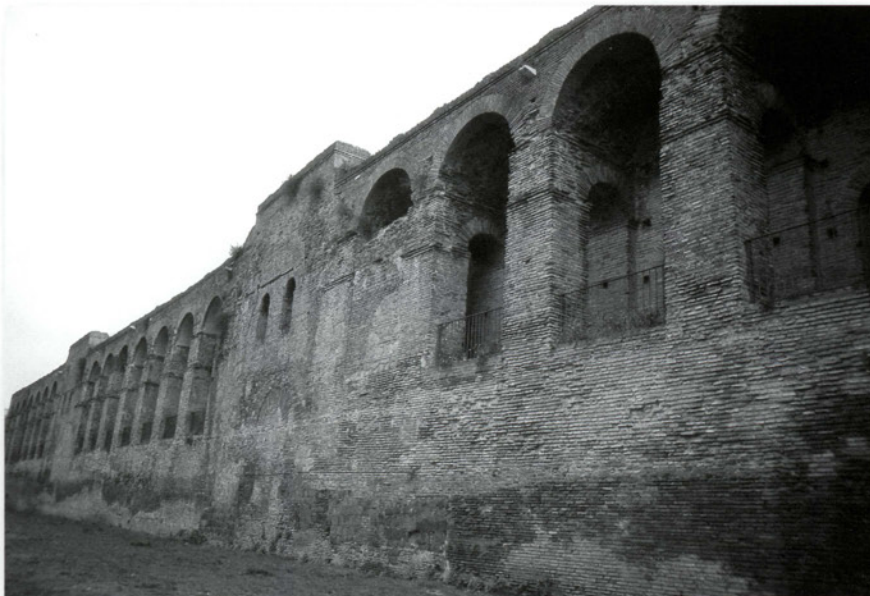
An interior view of Aurelian's wall in Viale Carlo Felice between the Amphitheatrum Castrense and Porta Asinaria, showing the Maxentian galleried wall sitting upon the Aurelianic gallery. (Author's collection)
