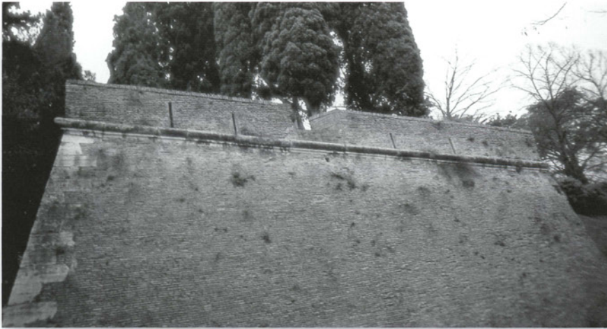
The Bastion in Viale Aurelio Saffi, erected under Pope Urbanus VIII (1643), equipped with gun-ports and loops. Guns of all calibres could be either fired over the parapet, or concealed and fired through embrasures cut into the parapet. (Author's collection)
