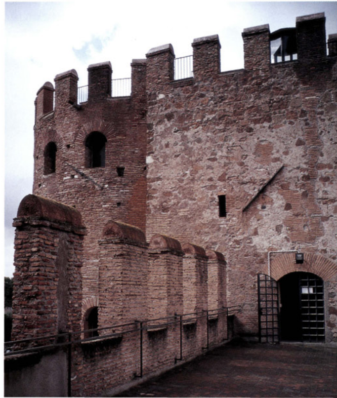
A close-up shot of the west gate-tower of Porta Appia, showing the rampart-walk and battlements; note the height of the merlons. (Author's collection)
