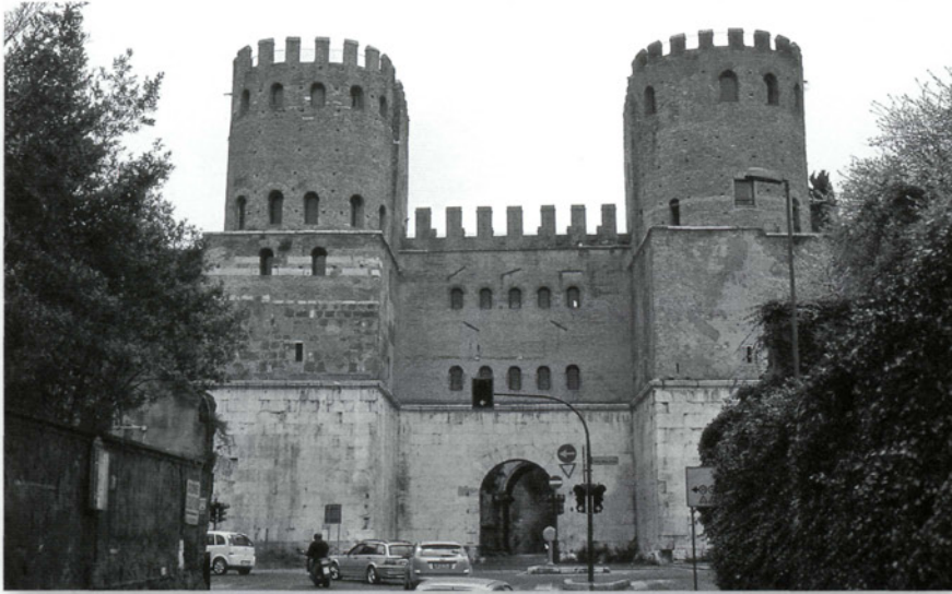
An exterior view of Porta Appia, looking north in Via Appia Antica. Originally, like all Type I gateways, Porta Appia was equipped with a double-span archway flanked by round-fronted towers. (Author's collection)
