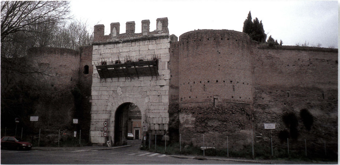
Exterior view of Porta Latina, looking west in Via Latina. This Type II gateway was altered under Honorius, whereby the single-span archway was reduced in width. The right-hand tower is original, but that on the left is Belisarian in date. (Author's collection)
