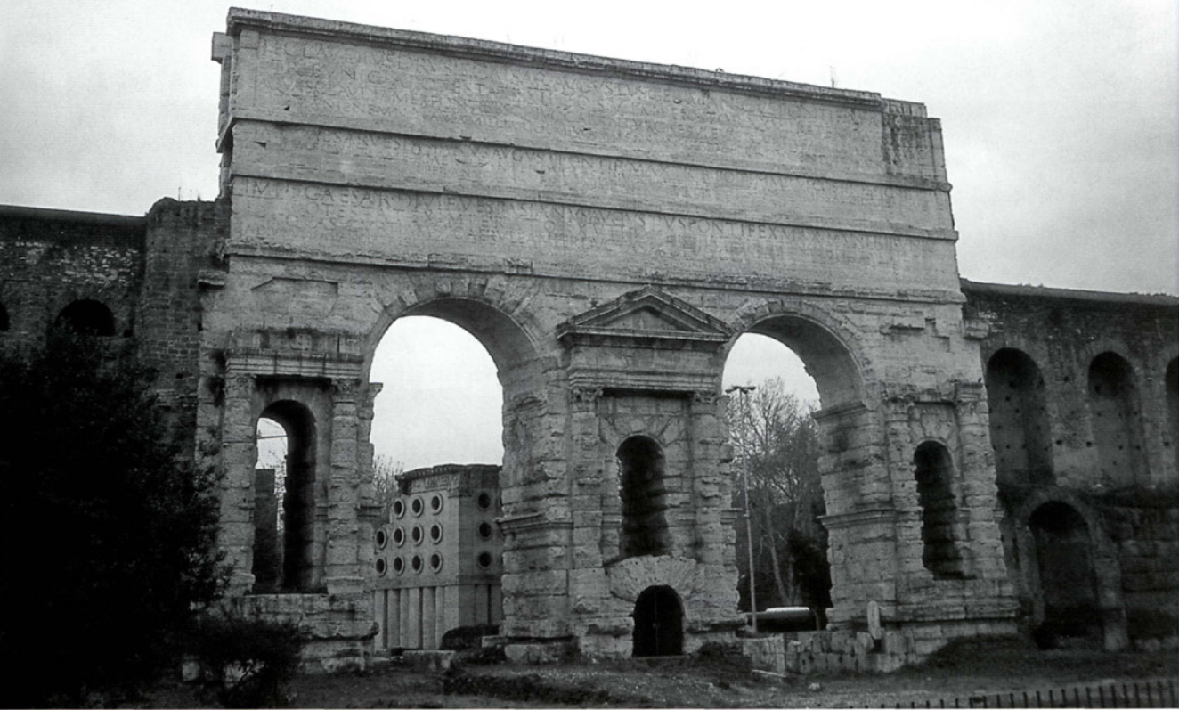
A Claudian monumental arch carrying the Aqua Claudia-Anio Novus, subsequently incorporated into Aurelian's wall to form the portals of Porta Praenestina-Labicana. (Author's collection)
