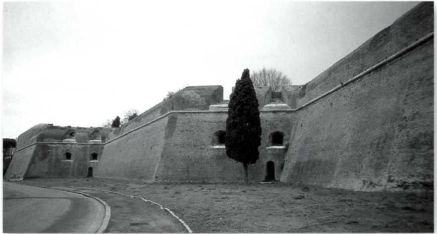
The Bastione del Sangallo (1538–42), an exterior view looking west in Viale di Porta Ardeatina. Quadrilateral, angled bastions were designed to resist artillery bombardment rather than human assault; the age of ‘vertical defence’ had passed. (Author’s collection)
