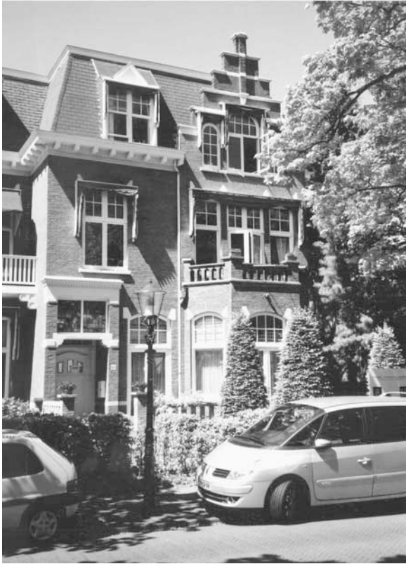
Plate 10. Van Stolkweg 10 (the “rabbit hole”), the nerve centre for Van den Heuvel’s many operations from 1962 to 1986 (Source: author)
