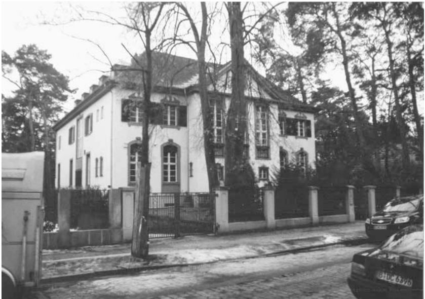
Plate 18. The Haus der Zukunft on Goethestraße in Zehlendorf, Berlin. This was used for training courses for participants from the Netherlands and other countries during the 1960s (Source: author)
