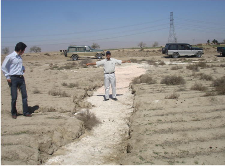
Fig. 16.16 An example of surface fissures in Mashhad Valley caused probably by excessive groundwater withdrawal and associated aquifer-system compaction. The fissure is located northwest of Mashhad City and to the east of the Tous. A GNSS station is marked by a triangle in Fig. 16.15 near the city of Tous (Source Motagh et al. [72])
