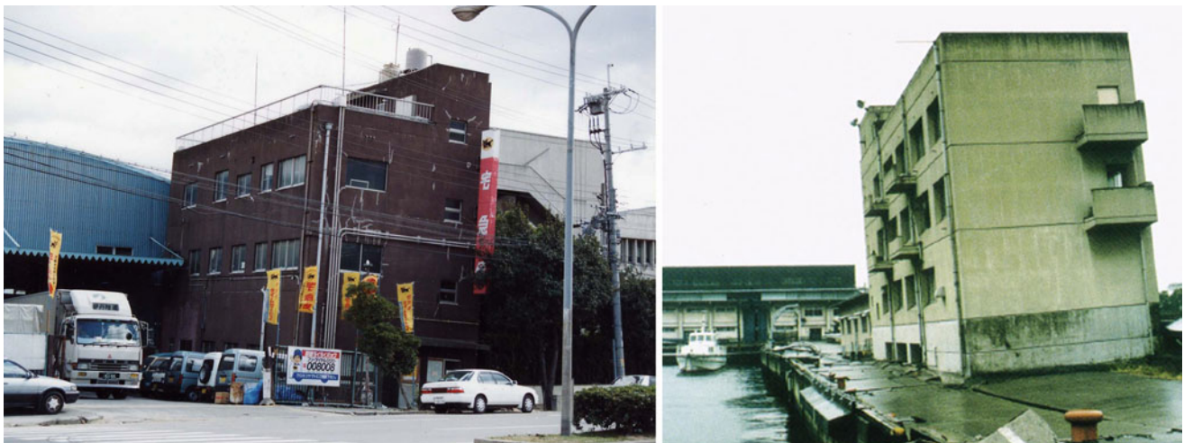
Fig. 7 Building failures after the 1995 Kobe earthquake
