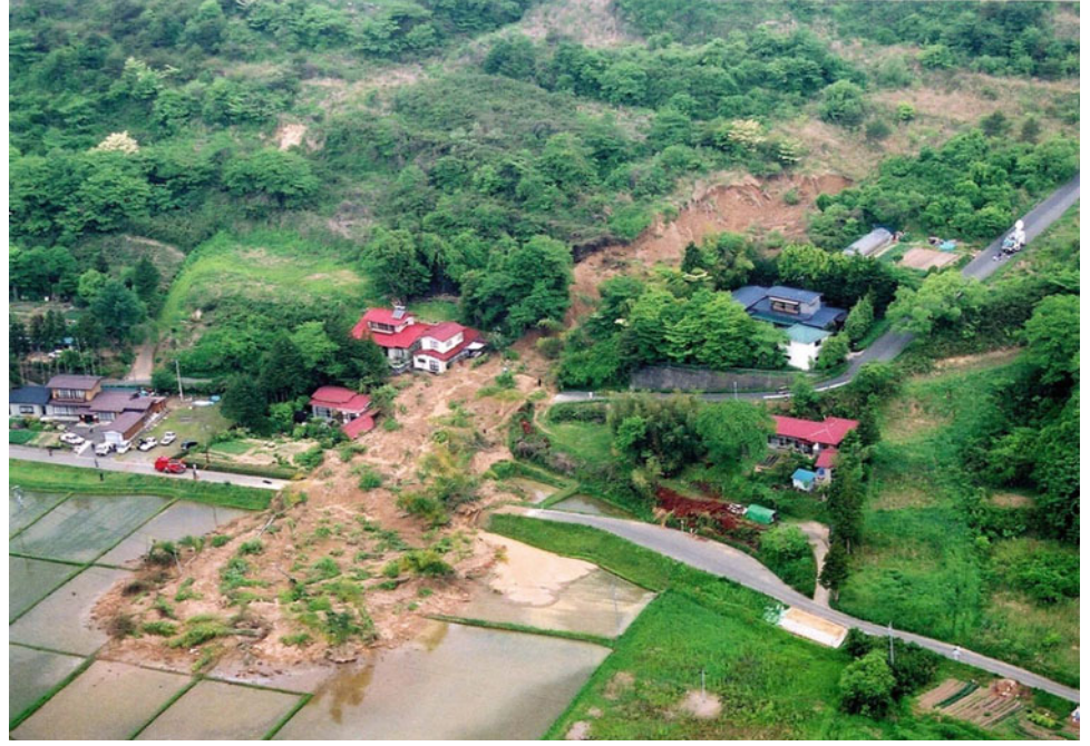
Fig. 3 Aerial photograph of the collapsed fill slope (Miyagi Engineering Co. Ltd.)
