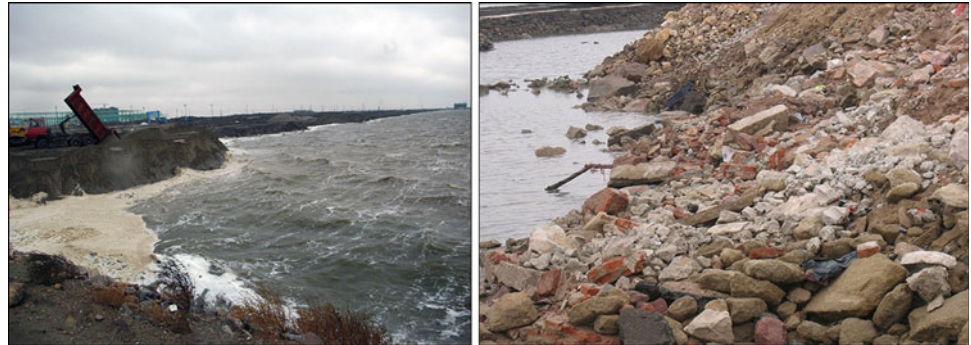
Fig. 3 Miscellaneous fill site in Weihai, Shandong province
