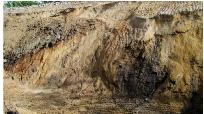
Fig. 6 Interface of sandstone and mudstone at K177 + 500 section
