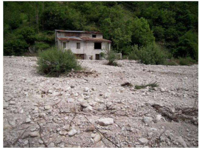
Fig. 5 Flooding of the external areas of the riverbed
