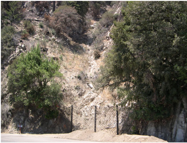
Fig. 2 Site 1 immediately after install (Courtesy Duffy)
