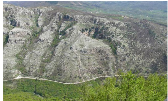
Fig. 1 View of the stiff rocky slope, over the Strada Provinciale Monte Cigno
