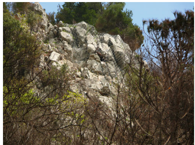
Fig. 17 Active stabilization of stiff rocky slopes with SPIDER® S4
