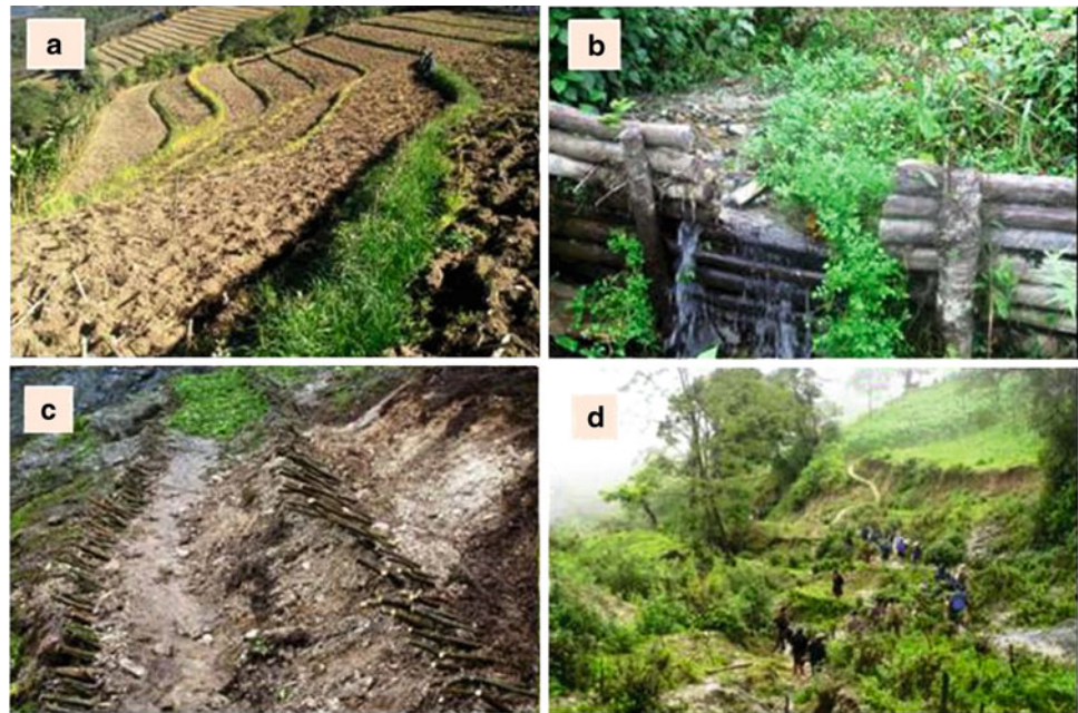
Fig. 3 Bio-technical measures for landslide mitigation – (a) Hedgerows introduced to reduce, surface, sheet and rill erosion, (b) Log check dams to mitigate gully erosion, which is completely filled with eroded debris from upslope, (c) Brush layering on landslides, and (d) Communities carrying out plantation in the landslide areas, part of the maize field washed away (Photo NSSC 2005a)
