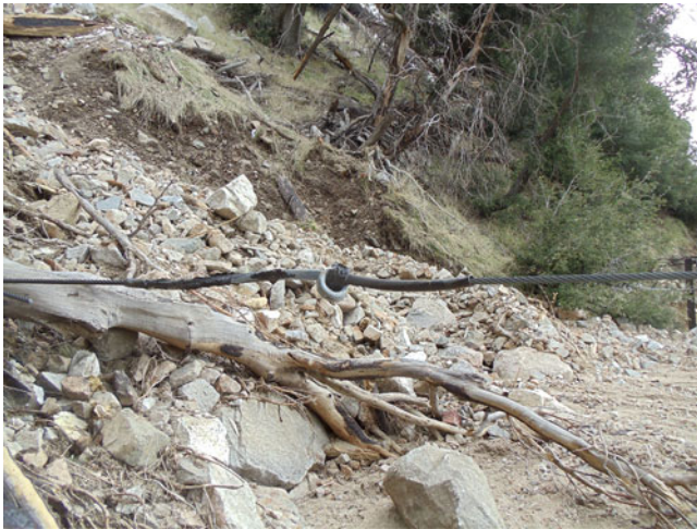
Fig. 9 Braking element ring completely closed in upslope tieback rope (Courtesy Duffy)
