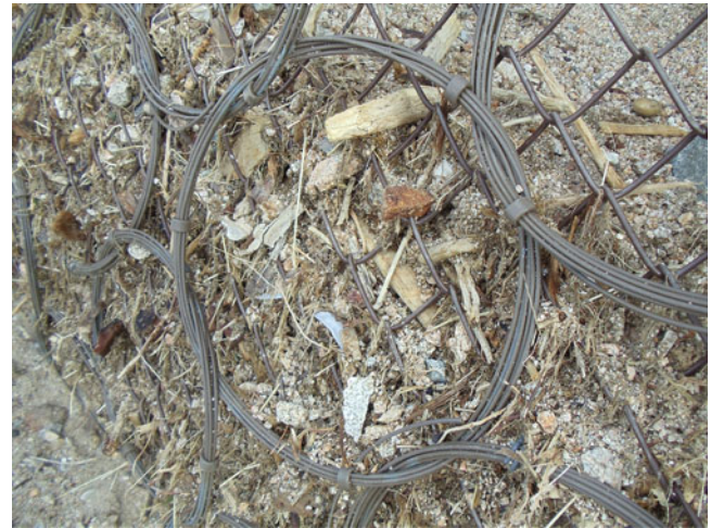
Fig. 10 Fine material and organic matter retained by nets and mesh (Courtesy Duffy)
