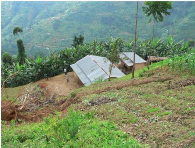
Fig. 5 Artificial terrace on steep slope without drainage system and lateral support. In the lower left corner of the photo (where tree fell) can be seen a shallow landslide and developing scarp
