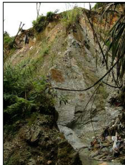
Fig. 10 Discontinuities in La Blanquizala creek
