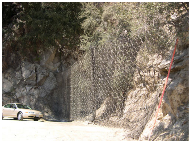
Fig. 4 Site 2 after installation
