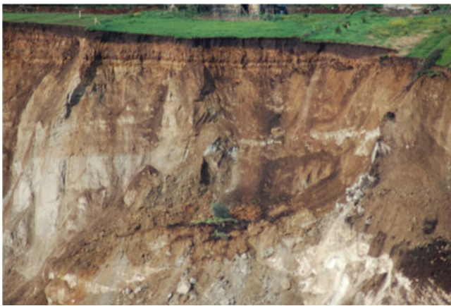
Fig. 4 Particular of the cracks and fracture on the upper north side of the landslide (Picture by Doglioni 2010)
