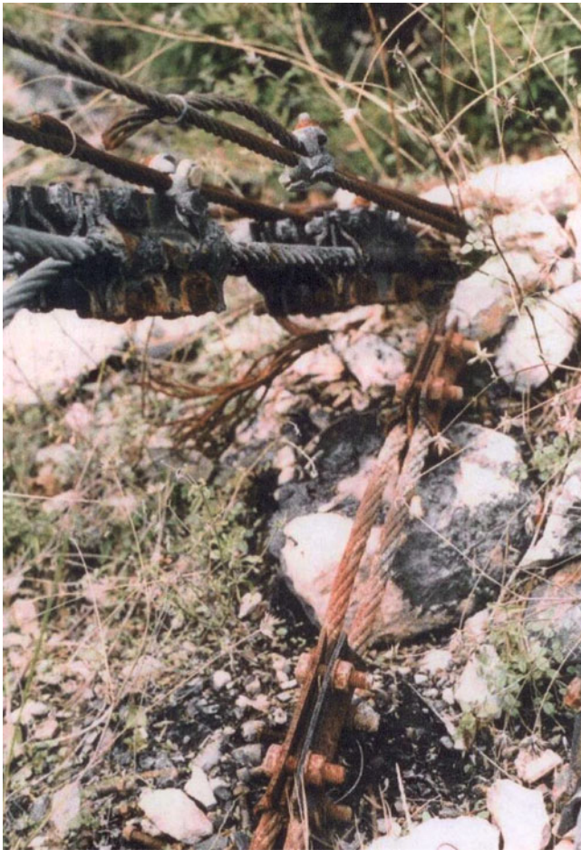
Fig. 13 Braking elements burned by wildfires
