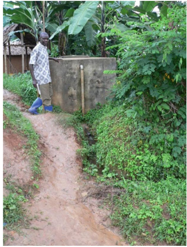
Fig. 4 Water tank releases water into the ground and causes erosion
