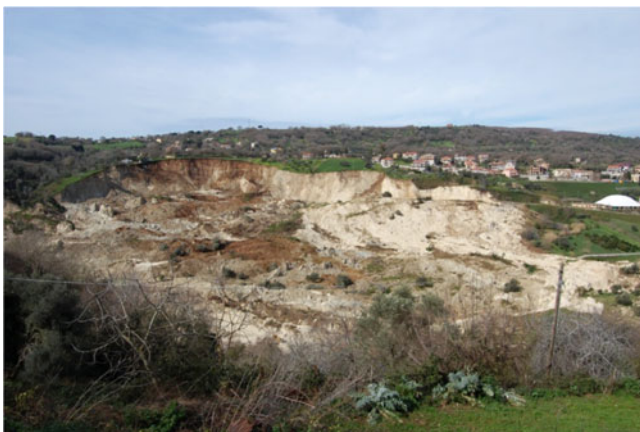
Fig. 2 Overview of Maierato landslide (Picture by Doglioni 2010)
