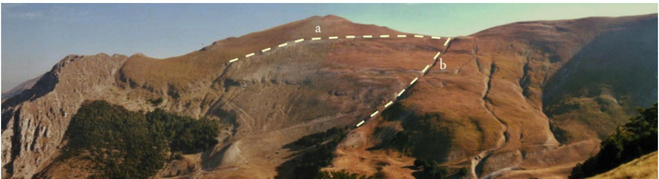
Fig. 5 The western slope of the Mount Bove shaped by geomorphological processes of different type, and the gravitational deformation in its central portion; a and b are the main discontinuities which bound the phenomenon
