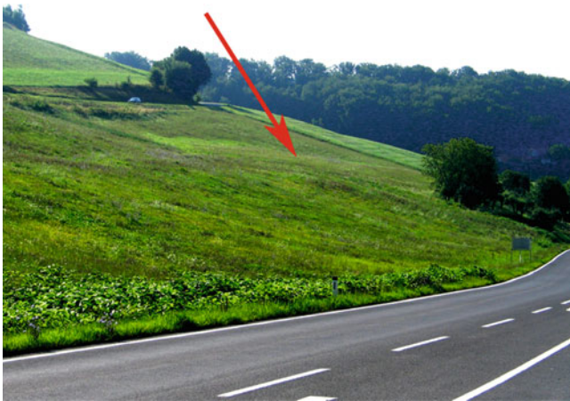
Fig. 2 Example of a slope that is affected by a deep seated creep process. Zones of depression, flattening ( red arrow ) and convex soil accumulation are visible. District of Jennersdorf
