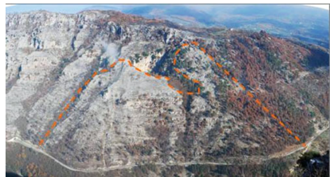
Fig. 4 Overview of the whole investigated area
