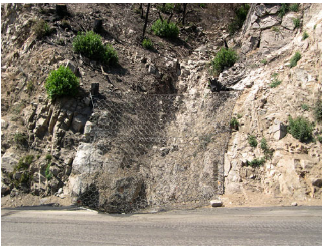
Fig. 6 Site 7 after install
