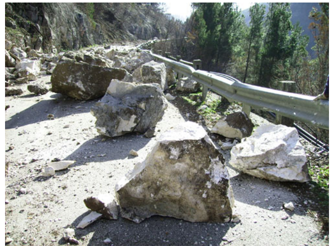
Fig. 15 Boulders on the road after slopes cleaning
