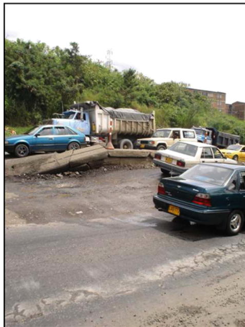
Fig. 4 Landslide in manmade fill of Northern Freeway
