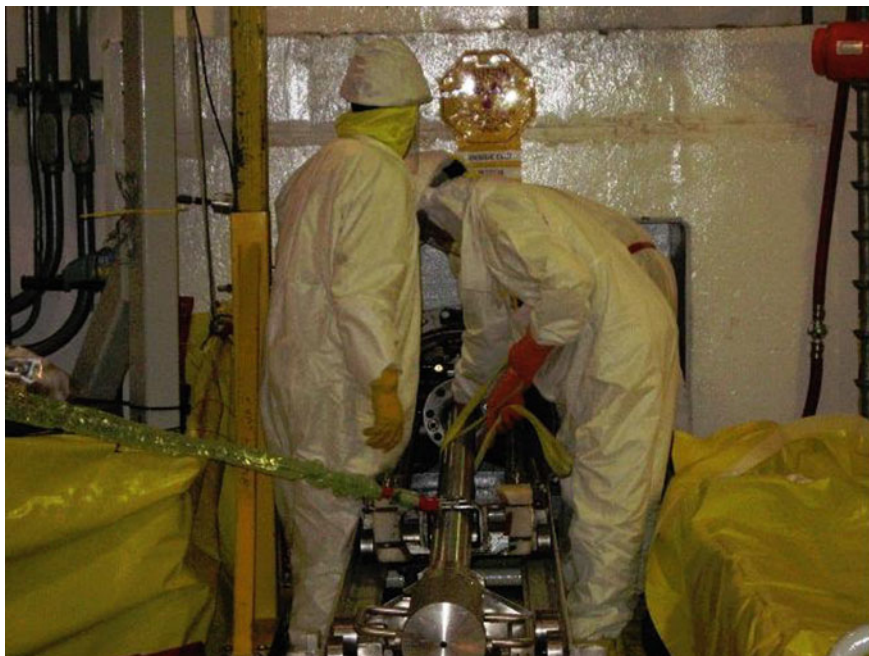
Fig. 6.22 A control rod drive mechanism being removed from the drywell (Courtesy of Progress Energy Inc.)
