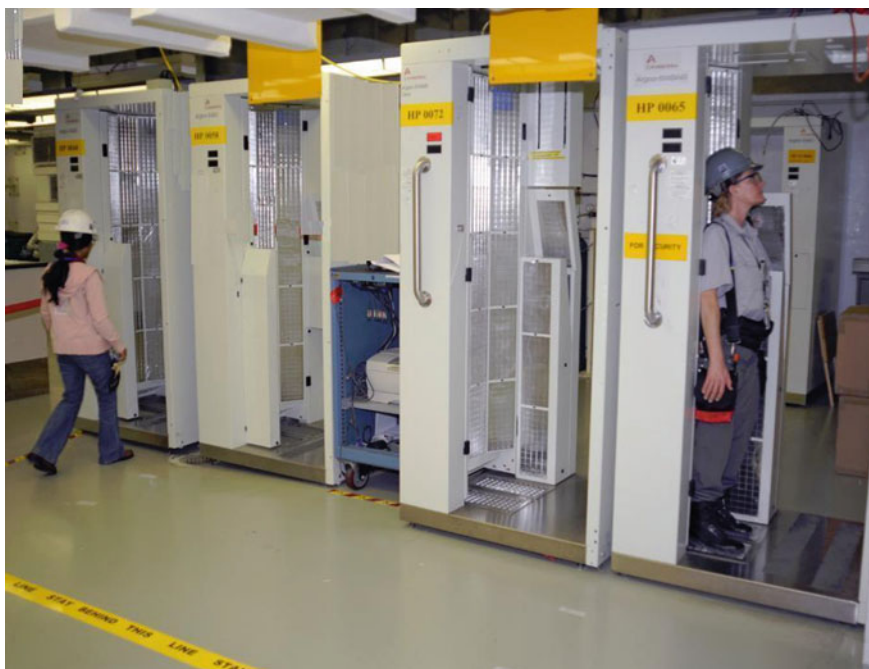
Fig. 6.18 Workers exiting the RCA are monitored by PCMs positioned at the RCA exit point. The RCA access control office is located to the left of the PCMs in this photograph. A gamma-sensitive portal monitor can be seen in the background behind the PCM shown on the right hand side of this photo. After exiting the PCMs workers then pass through the portal monitors (Courtesy of Luminant)
