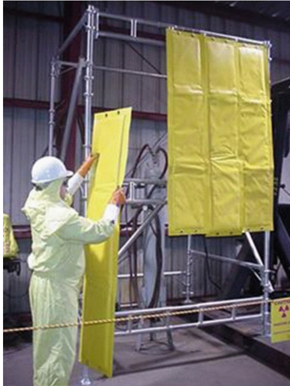
Fig. 7.9 Use of quick-erect Excel scaffolding as a rack to hold temporary shielding (Courtesy of BHI Energy www.bhienergy.com )
