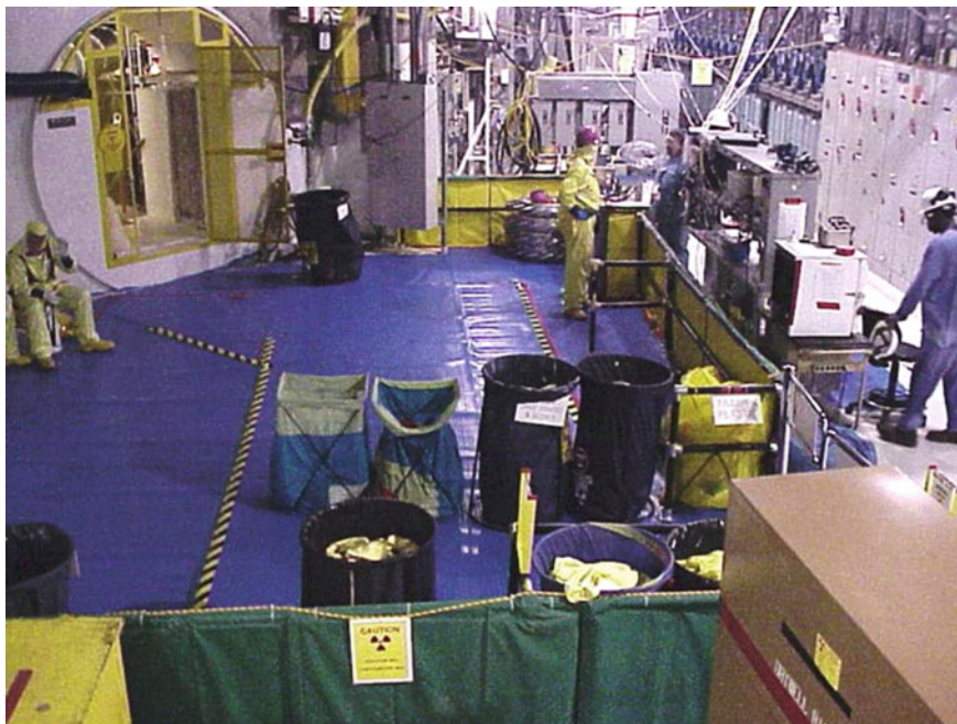
Fig. 6.21 Access control area established at personnel airlock entrance to a drywell to support outage activities. The RP control point is on the right hand side equipped with video monitors and various radiation monitoring and survey equipment (Courtesy of Progress Energy Inc.)
