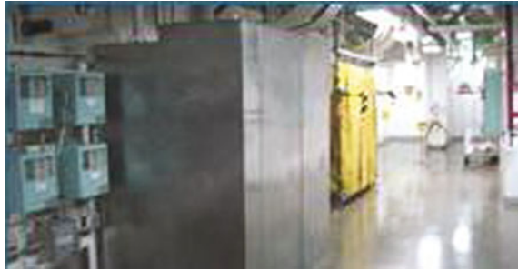
Fig. 9.16 Water shield utilized to provide long-term shielding in general plant walkway area (Courtesy of Nuclear Power Outfitters, www.nuclearpoweroutfitters.com )
