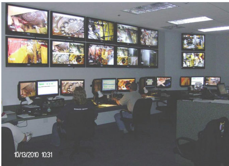
Fig. 6.23 This figure depicts a remote monitoring facility used by radiation protection personnel to monitor multiple ongoing radiological work activities during outages. The facility provides video coverage and is equipped with direct communication to the multiple work locations shown on the monitors (Courtesy of Florida Power and Light Company)
