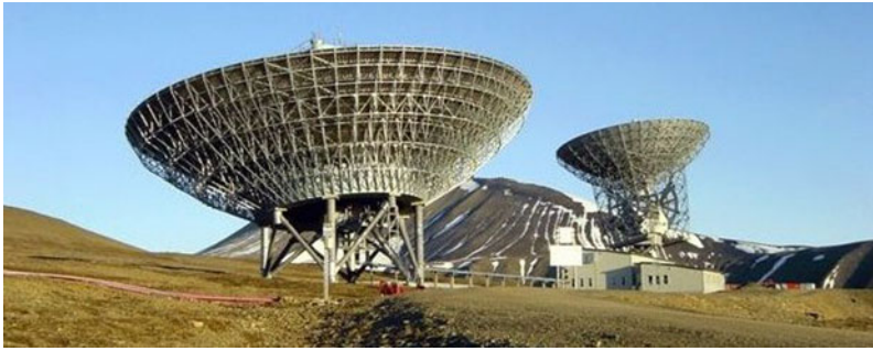
Fig. 14.1 The 42 m field-aligned dish ( left ) of the EISCAT Svalbard Radar near Longyearbyen and the steerable 32 m dish ( right ). The facility started operation in 1996 and several research projects have been using the results of this radar facility during the period of the CAWSES Priority Program. (Picture: EISCAT Association)
