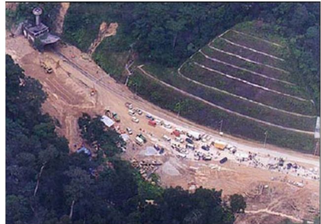
Fig. 9 General view of debris flow at Genting Sempah
