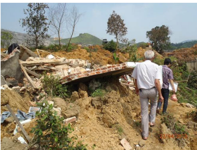
Fig. 6 A house was completely destroyed
