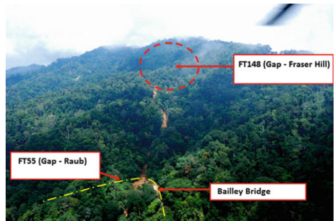
Fig. 7 Aerial view of the road at FT 148 and FT 55, the impact of a debris flow in February 2009
