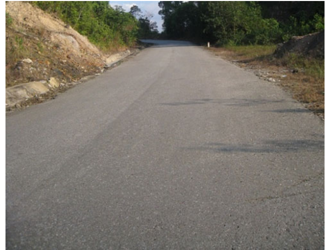
Fig. 4 No deformation or cracks on the road at landslide No. 21
