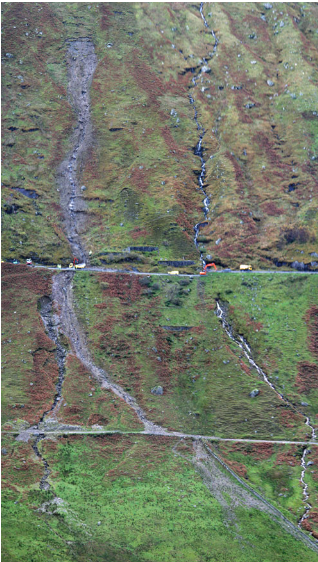
Fig. 1 View of the 28 October 2007 debris flows at the A83 Rest and be Thankful
