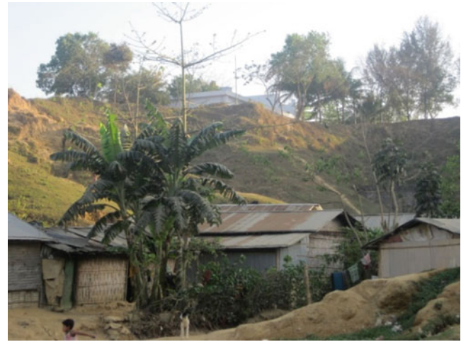
Fig. 1 Vulnerable locations in a built-up area
