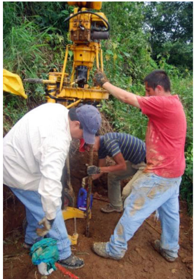
Fig. 7 Installation of the equipment
