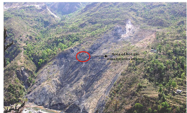
Fig. 2 Field photograph showing the view of the Rawana landslide and the area of hot gas emanations in 2005
