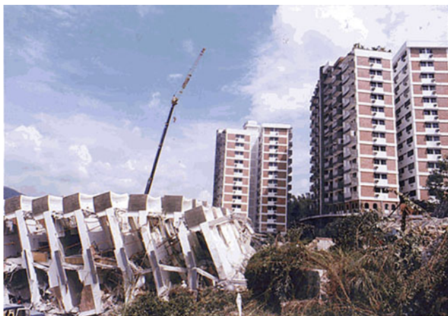
Fig. 1 The collapsed apartment building with the abandoned ones in the background
