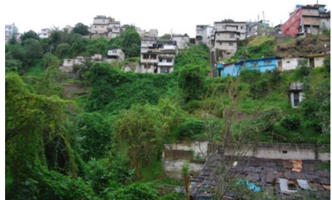
Fig. 2 Settlements on steep slopes and unstable susceptible volcanic soils
