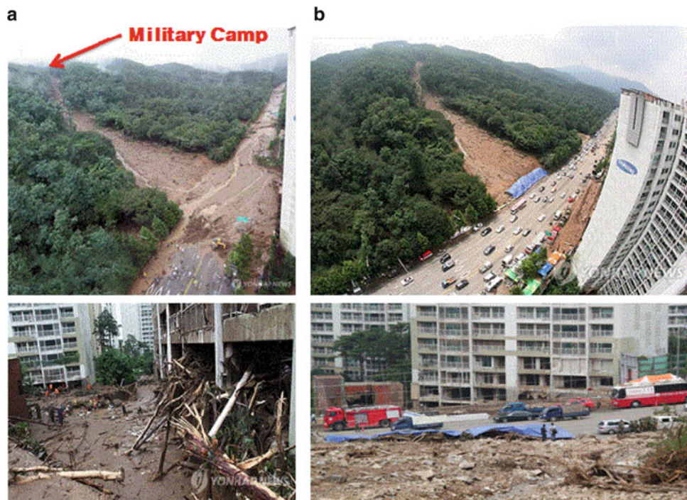
Fig. 2 Twelve large landslides occurred associated with 230 mm rainfall at Mt. Umyeon, Seoul on 27th July 2011. The landslides caused 18 deaths and 51 were injured. The proximity of a military camp at the
