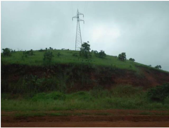
Fig. 1 Electrical facility on a hill near Nsukka, South-East Nigeria
