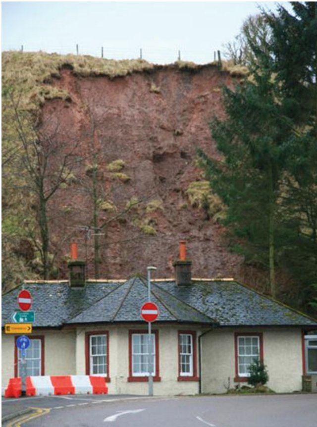
Fig. 4 Urban landslide at Bervie Braes, Stonehaven, on the north-east coast of Scotland (February 2010). The landslides at Bervie Braes occur on a raised sea cliff
