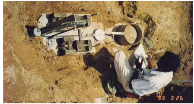
Fig. 4 Field direct shear testing equipment and installation work before testing
