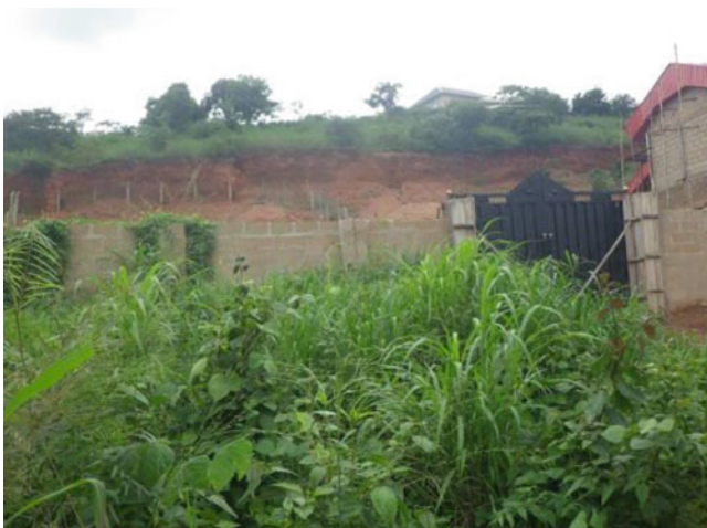
Fig. 3 A residential zone on a vulnerable hillside in Nsukka
