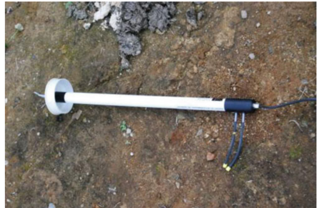
Fig. 6 Piezometer installed on the slope. A 60 m wire connects the piezometers to the automated-registry system
