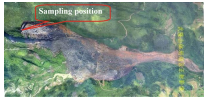
Fig. 1 Image of the Jiweishan landslide
