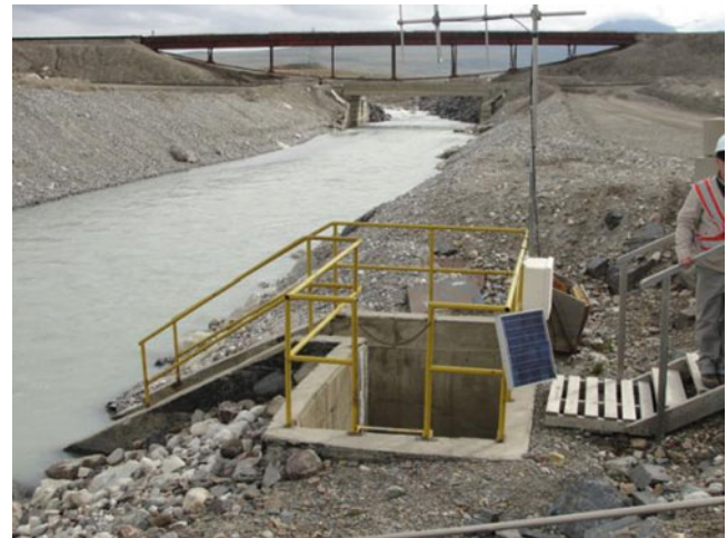
Fig. 7 July 2012. Pulp line across the Kumtor River and a hydrometric structure of the Kumtor Operating Company on the Kumtor River c. 4 km from the source
