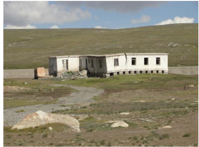
Fig. 6 Kumtor syrt. The Tien Shan weather station. 3,654 m asl. Not operational since 1948. The building has been deformed by permafrost degradation
