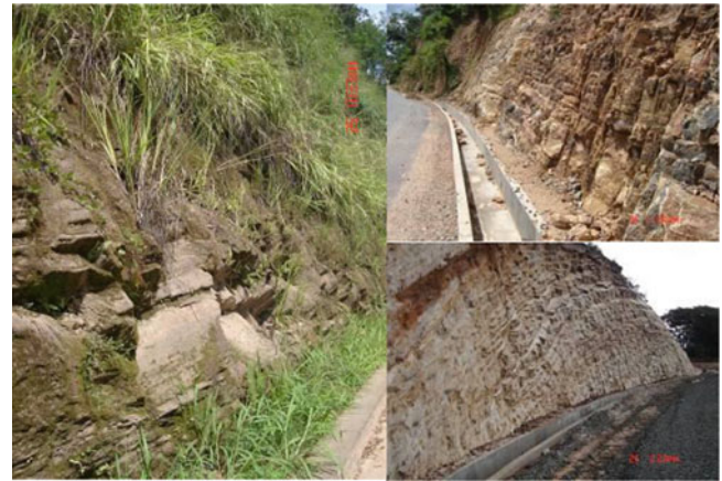
Fig. 16 Highly foliated under dip conditions at cutting with long term standstill section at tropical weather conditions
