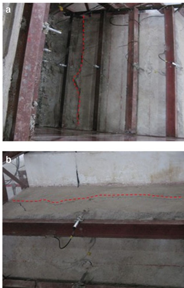
Fig. 7 Cracks in the mudstone slope model (a) toe of slope (b) crest of slope
