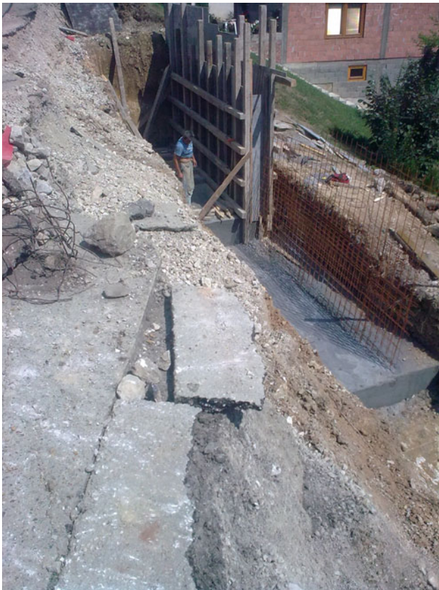
Fig. 7 Concreting of one section of retaining wall
