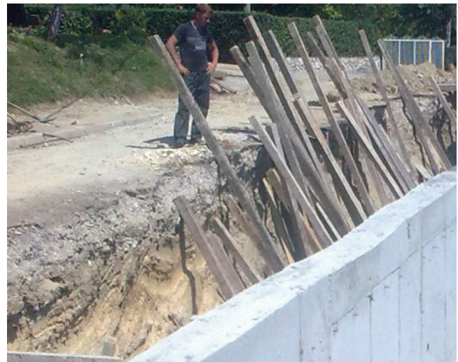
Fig. 8 Construction of a retaining wall for landslide remediation
