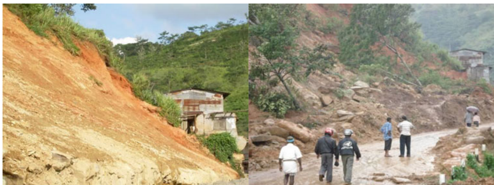
Fig. 3 An example of negligence during the construction stage to evaluate and design for stability of rock slope, geological setting, overburden parameters and land use during road widening works
