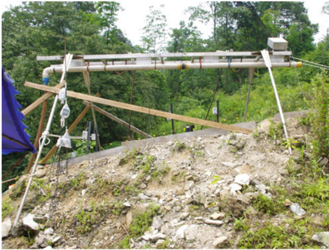
Fig. 7 Photo of the site together with the instruments
