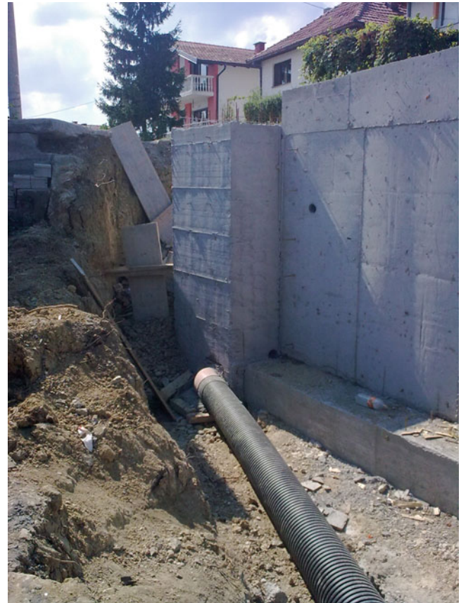
Fig. 10 Drainage of drain water from the manhole
