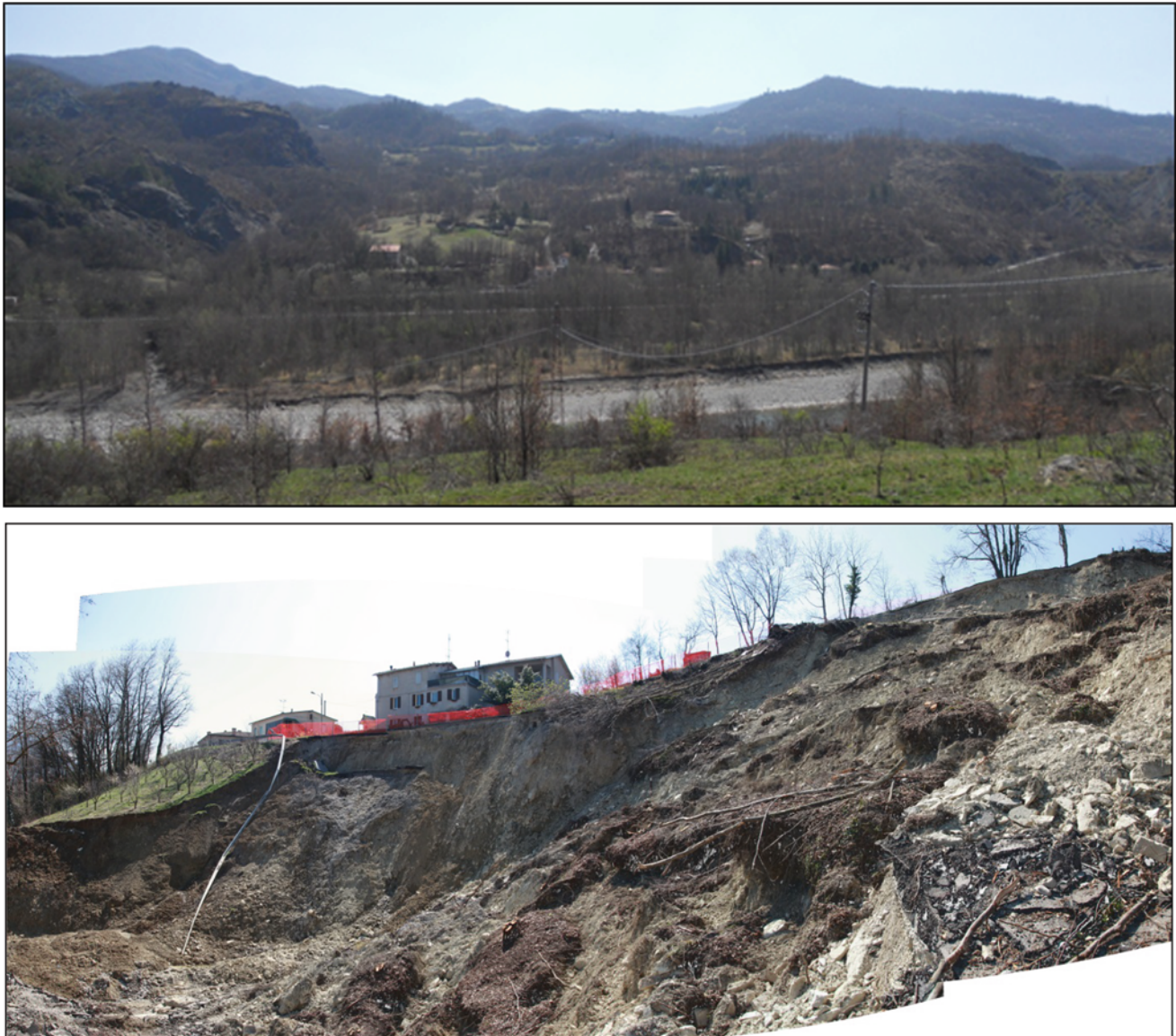
Fig. 3 View of the the Roccamurata landslide taken from the left bank of the Taro River ( above ); the Boschetto landslide crown area, taken a few days after its reactivation ( below )
