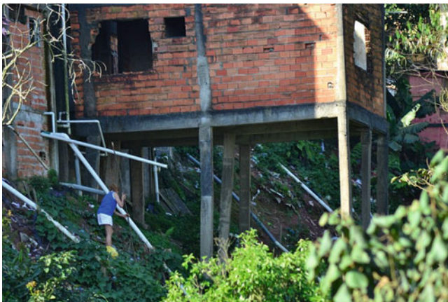
Fig. 2 In this photo, there are many drainpipes installed by the inhabitants themselves. These pipes throw away waste water in the slope (Source: Erica Akemi Goto 2011)
