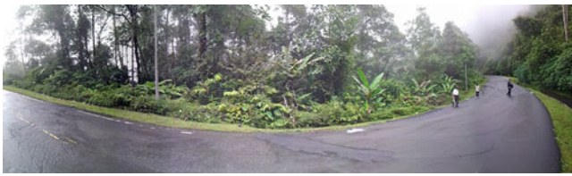
Fig. 7 Panoramic view of embankment fill at Federal Road between Penampang and Tambunan
