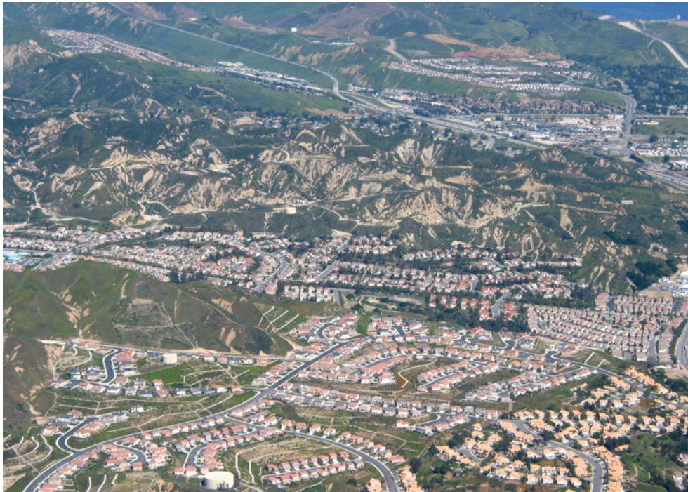
Fig. 1 Landslides are characterized by a complex distribution in space and time, which makes cost estimation difficult. This photograph shows widespread landslide activity on highly urbanized slopes in southern
