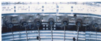
Water catchment boring
