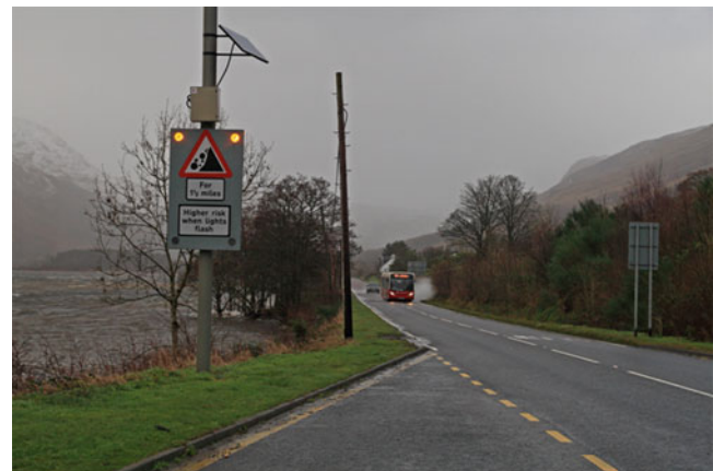
Fig. 2 Wig-wag warning sign in operation
