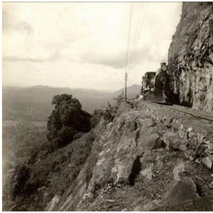
Fig. 1 Construction of Colombo—Kandy Railway in Sri Lanka during, British era 1796–1948 (Source: http://lankapura.com )
