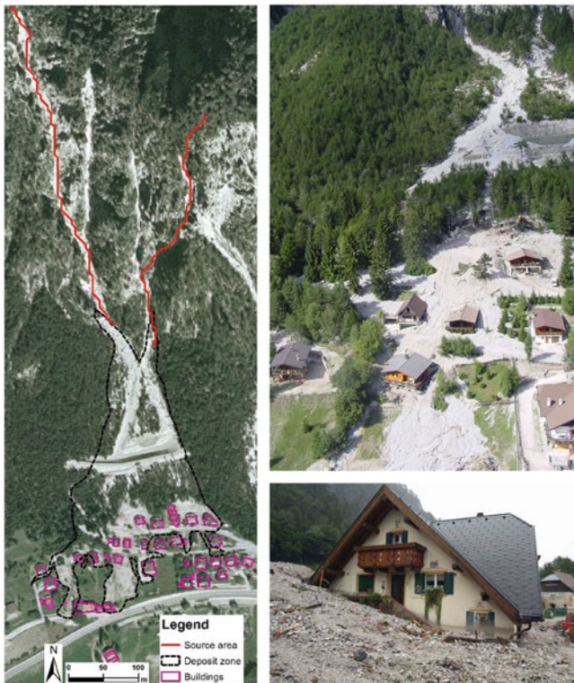
Fig. 1 (Left) The Abitato Cucco 2003 debris flow from the initiation to the deposit zone and (right) the breach of the barrier which damaged several houses
