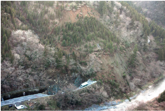
Fig. 1 A S&R activity was done in the deposit of a landslide where mass of up-slope was still sliding during activity
