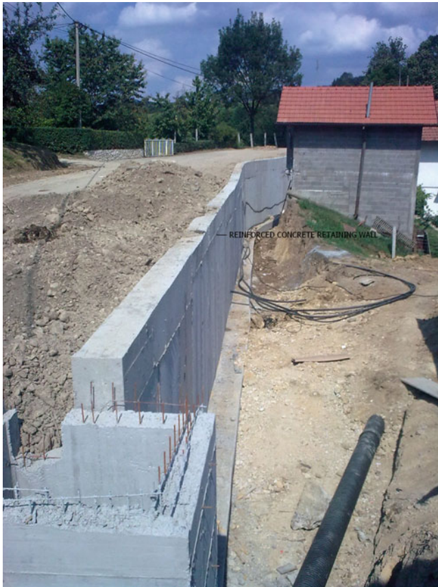
Fig. 9 Reinforced concrete retaining wall and revised manhole
