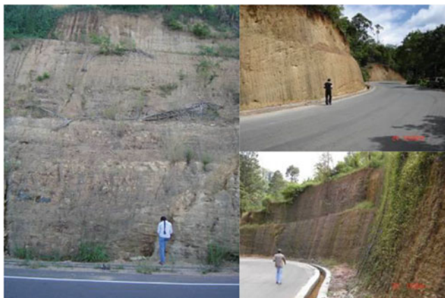
Fig. 15 Typical field showing completely weathered rock cutting, which remains as stable even after subjected to periodic wetting and drying in last 20–30 years
