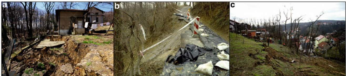
Fig. 3 Examples of landslides endangering/damaging houses or public roads in the winter of 2013 in Zagreb
