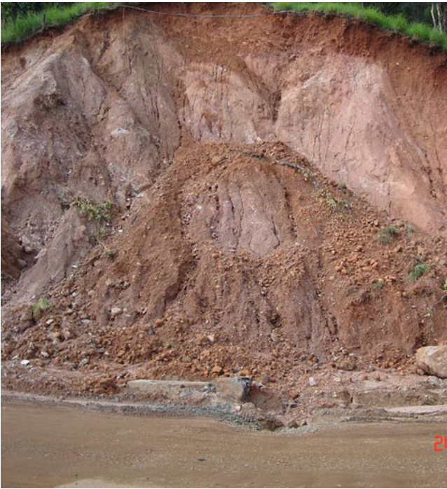
Fig. 7 Relatively large soil slump feature in residual soil due to lack of appropriate remedial measures
